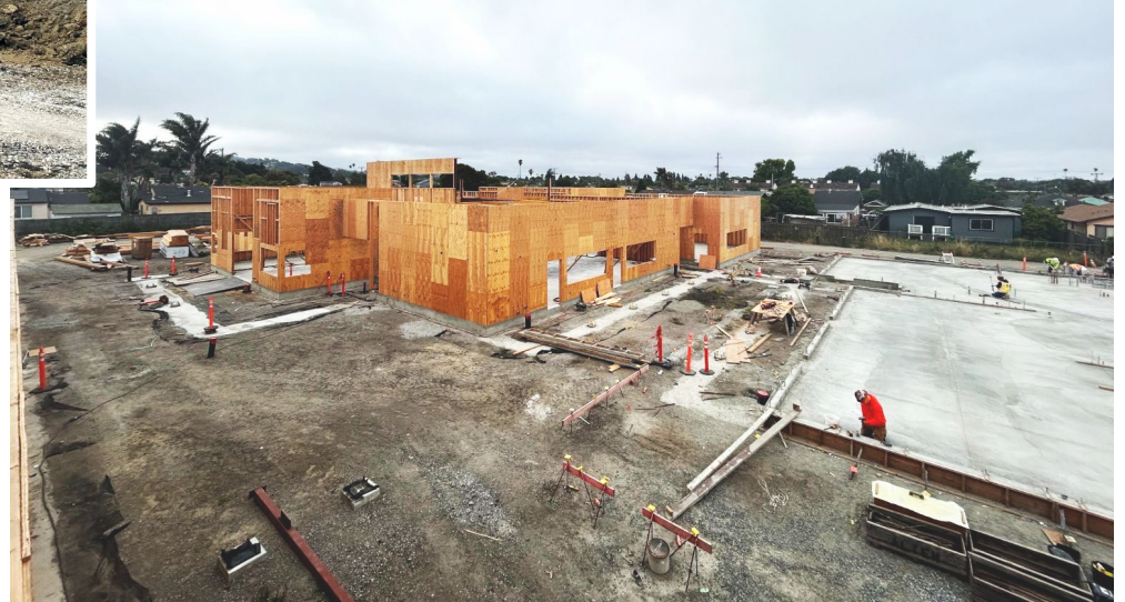
Building B - Wall Framing
