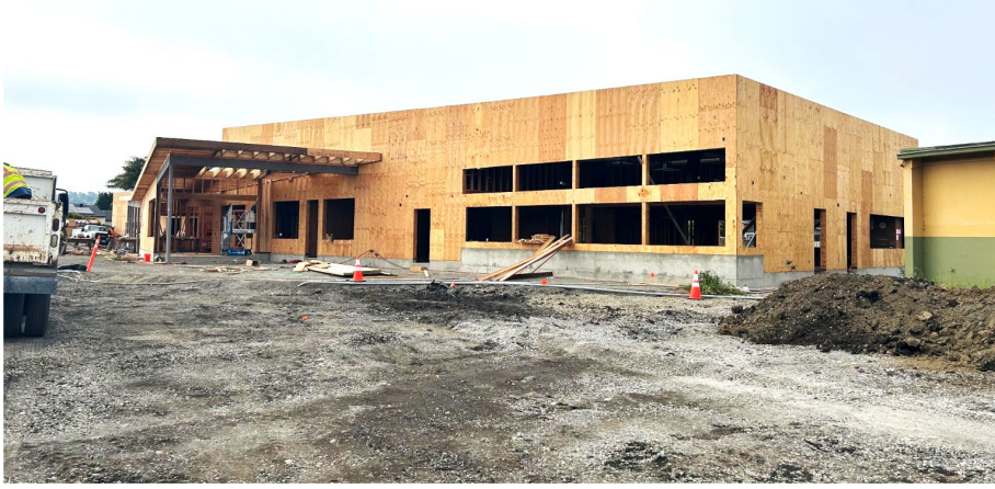
Building A - Utility Rough In
