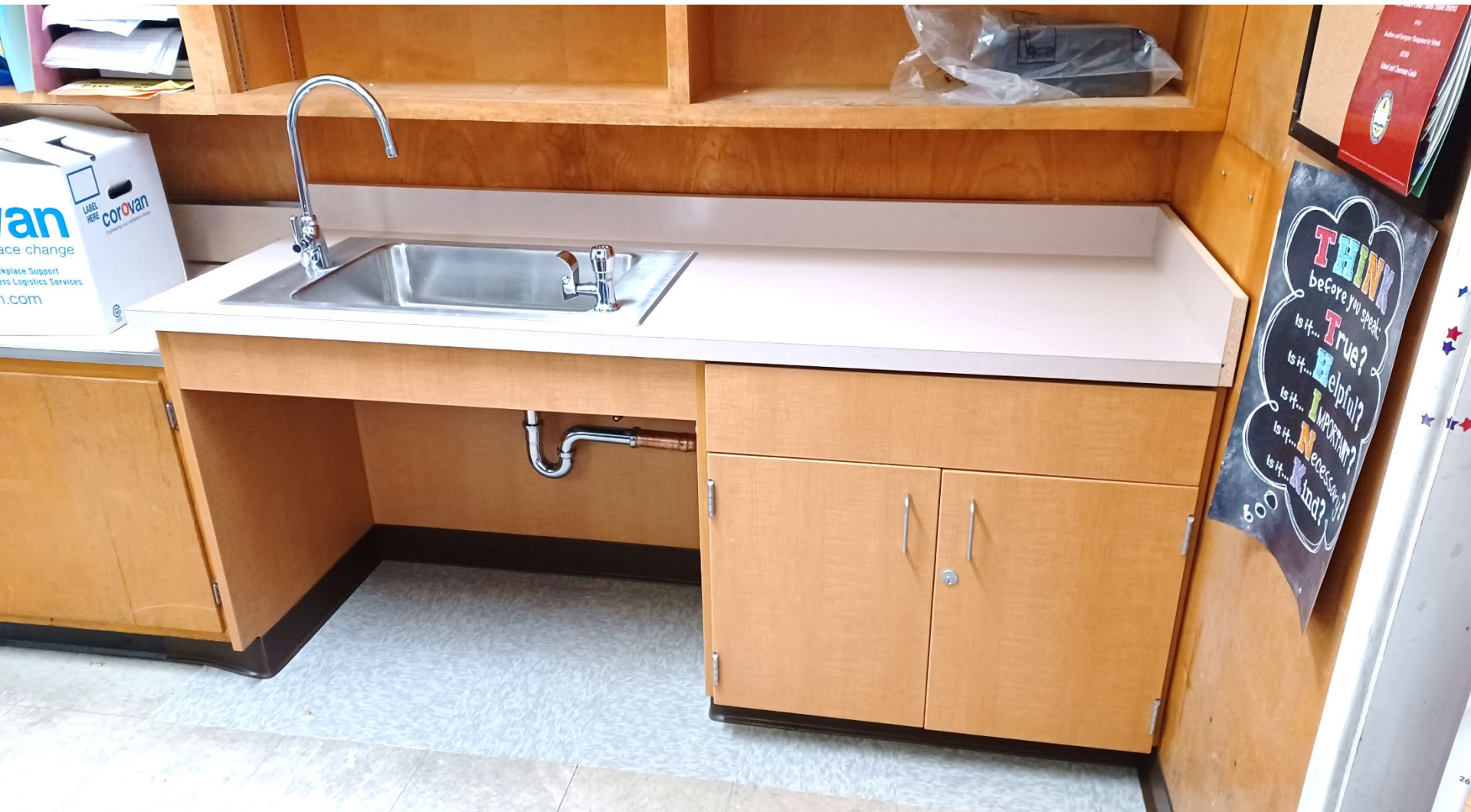
New Classroom Sinks
