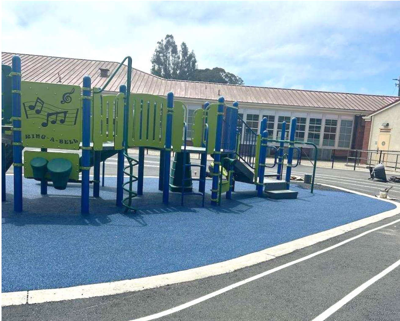
New Kindergarten Play Structure – Installing the Safety Surface
