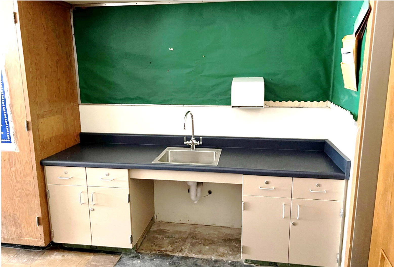
New Classroom Sinks
