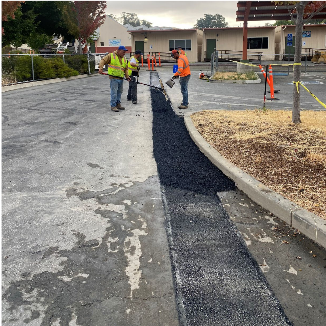
New Underground Utility Pathways – Installing asphalt patch
