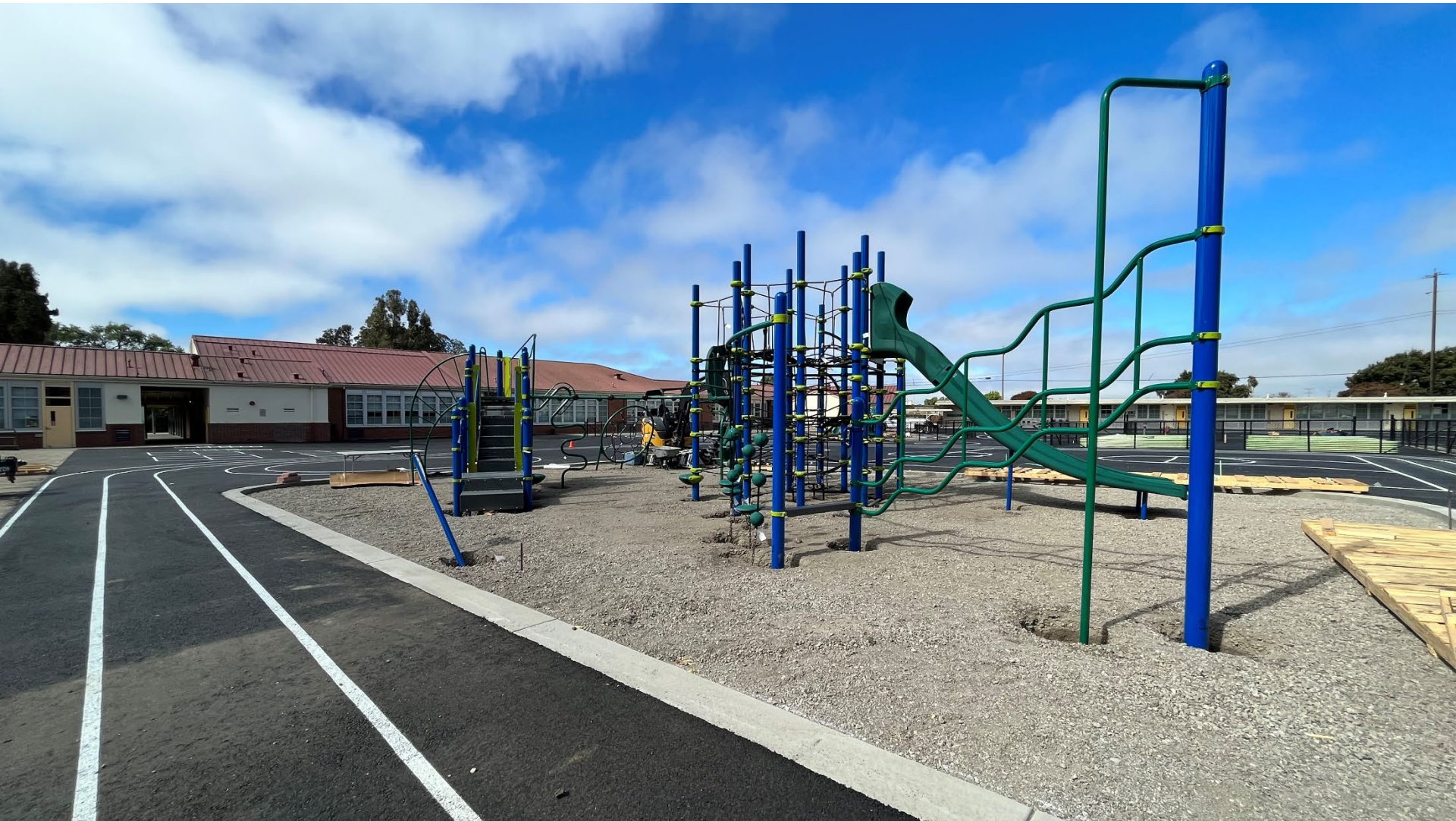
New Primary Play Structure – Installing the Foundations
