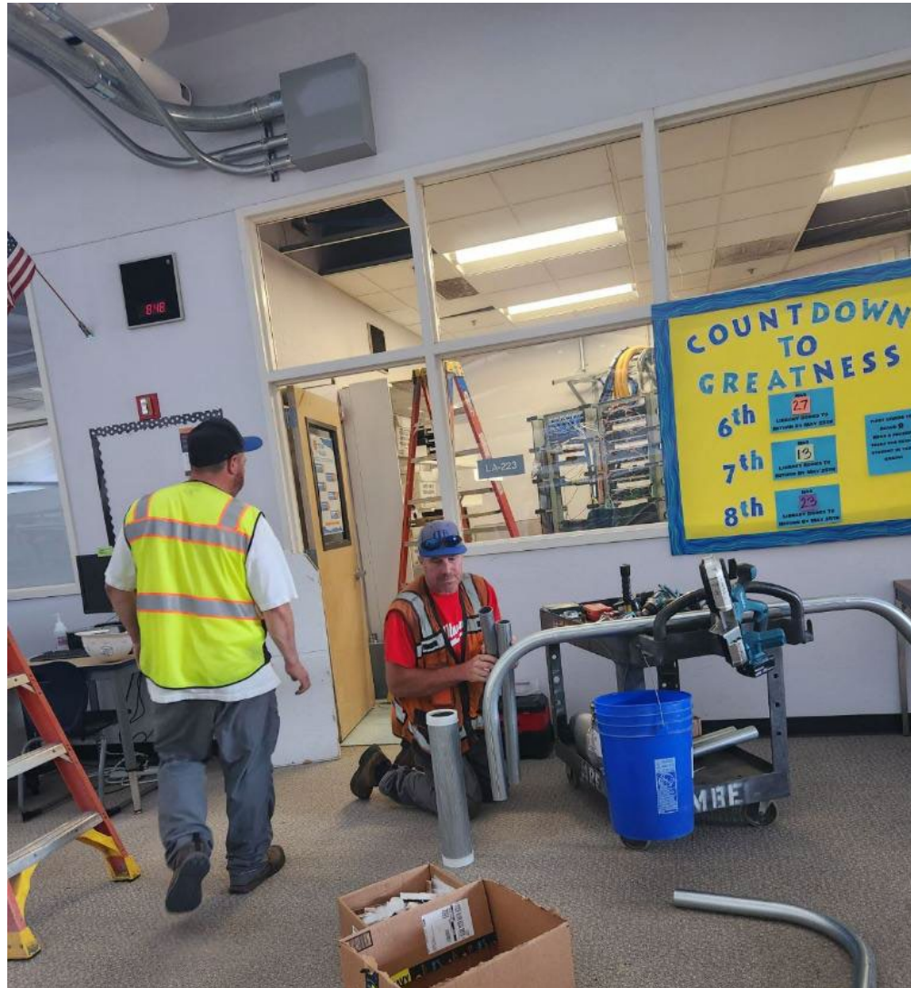
New Utility Pathways – Installing Conduit
