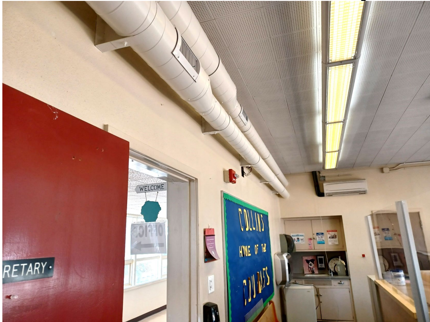
New Duct Work in the Main Office
