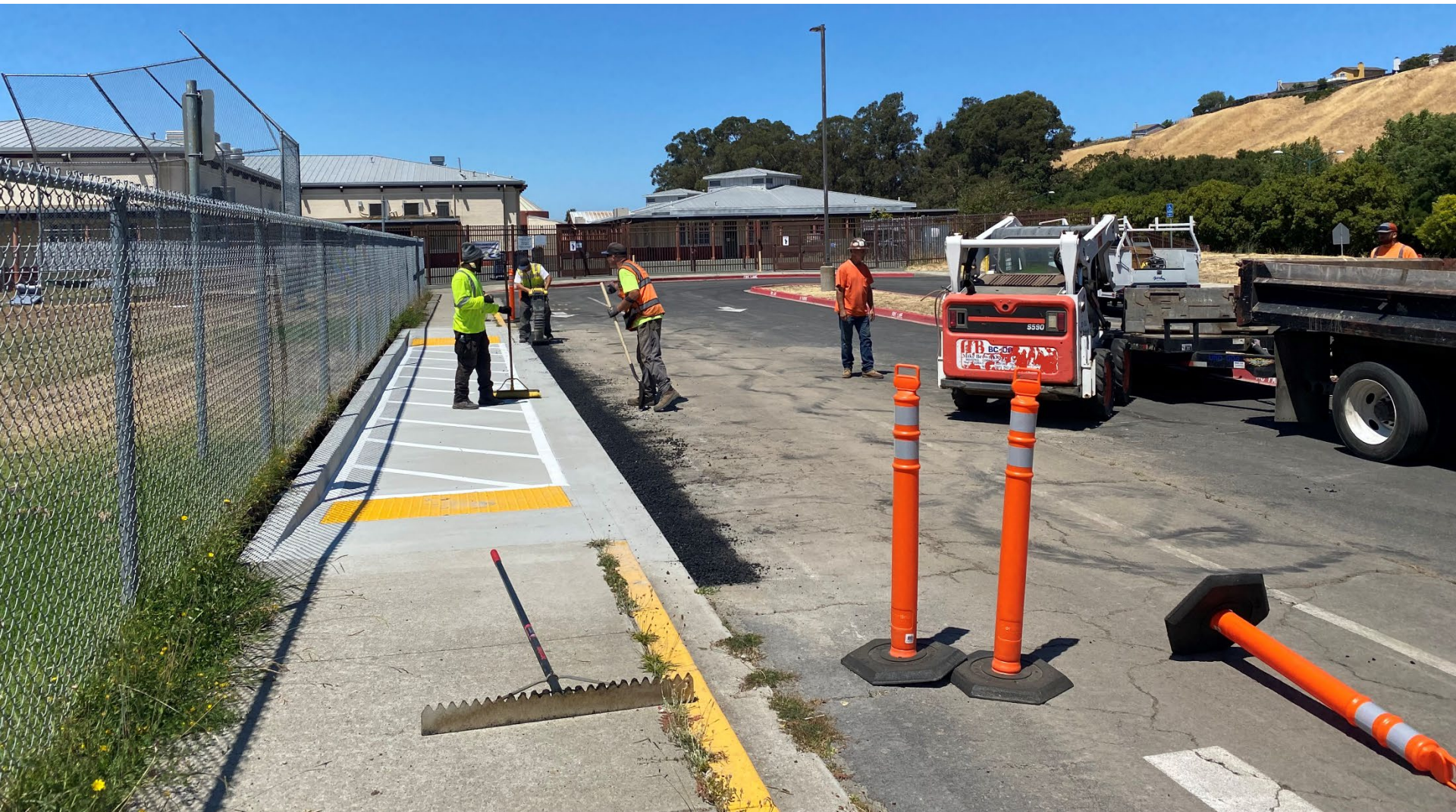
Middle School Drop Off – Installing asphalt
