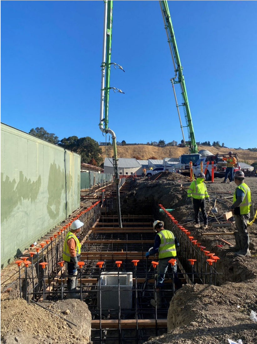
Installing the west side bio basin
