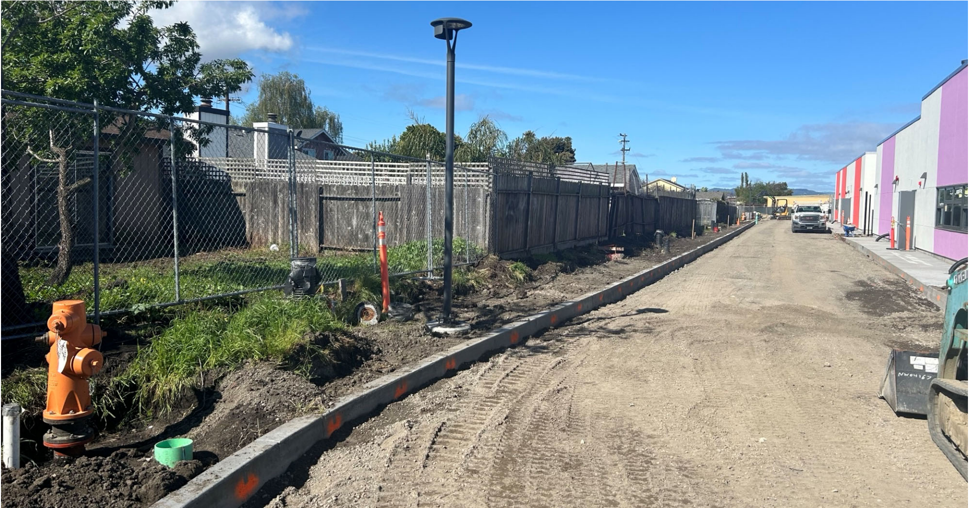
Curb and Gutter for the Emergency Access Road
