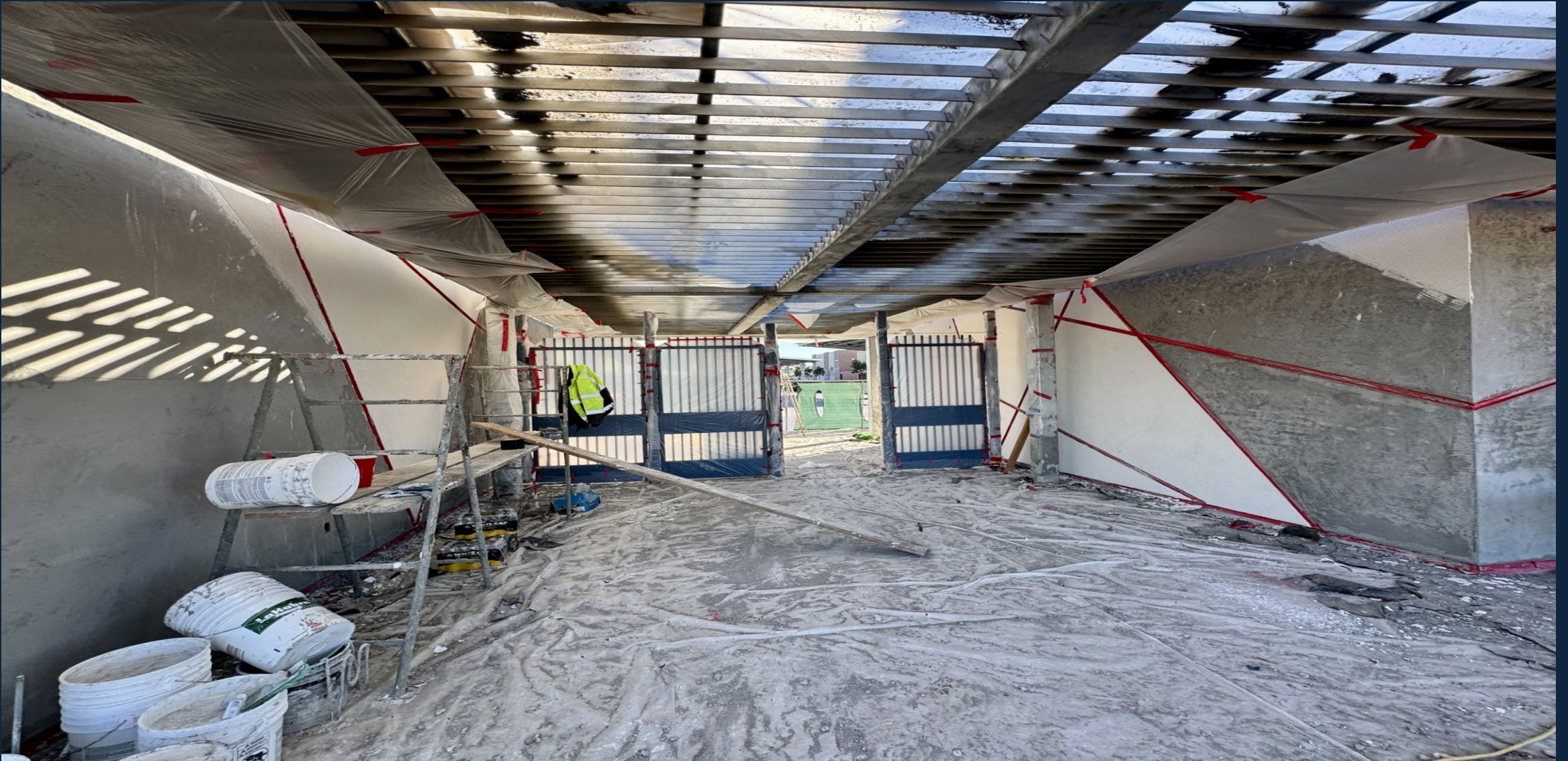
Ornamental Fence Installed at Entrance
