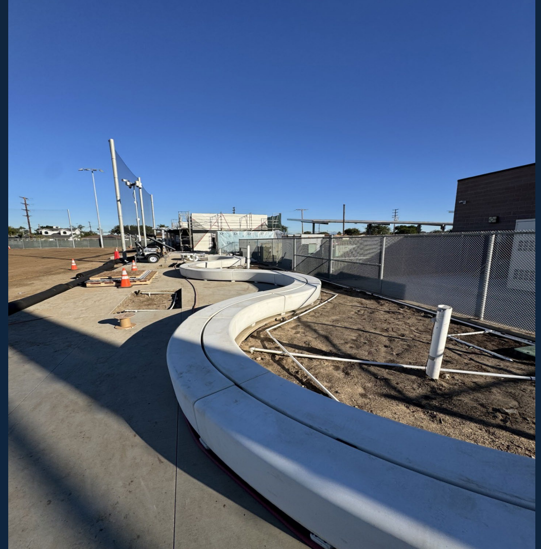
Concrete Seat Wall Installed
