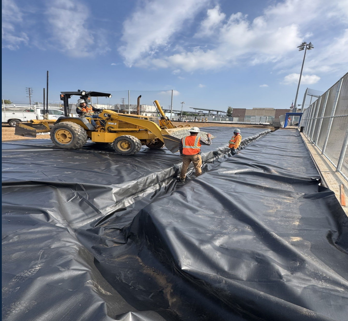
TenCate Installing Perimeter Drain Lines
