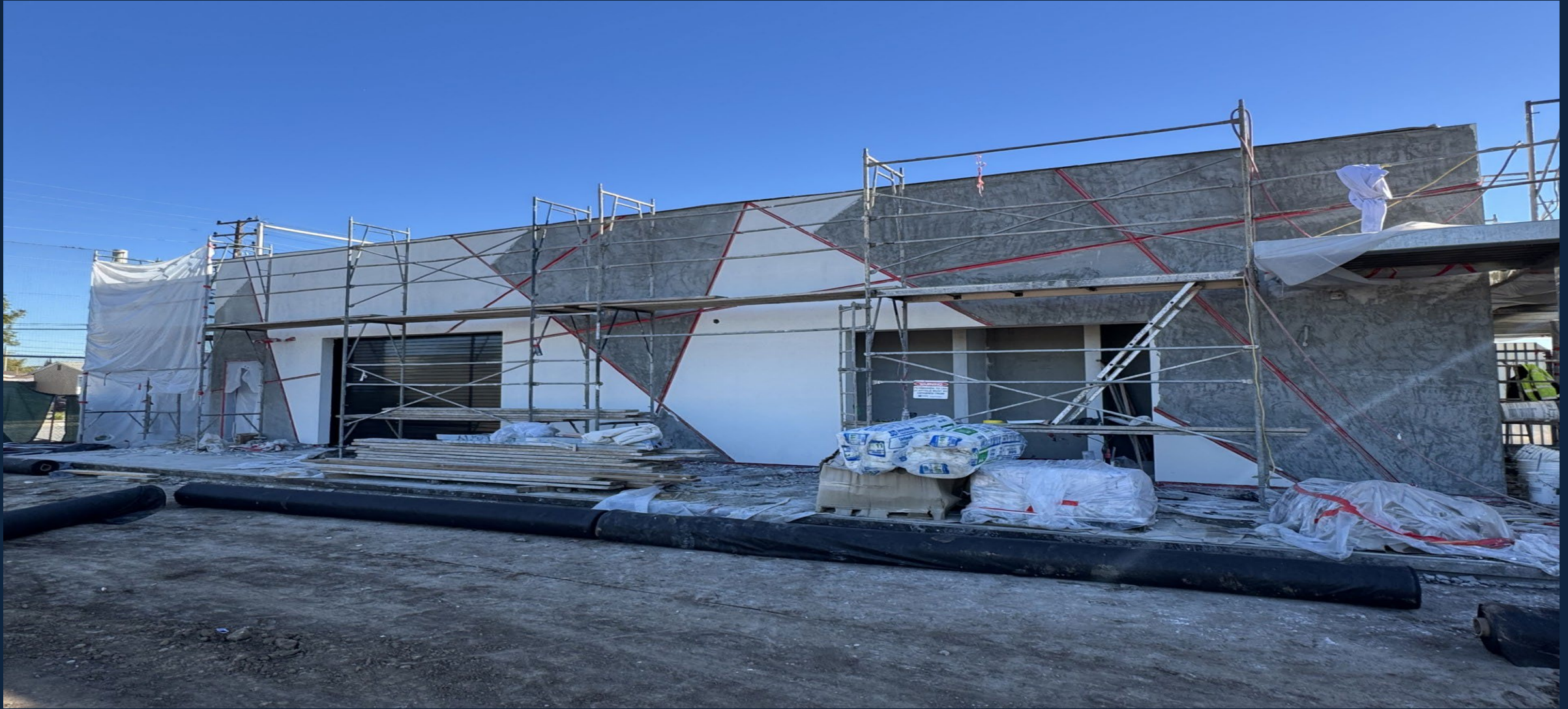
Restrooms & Storage Building – Back View
