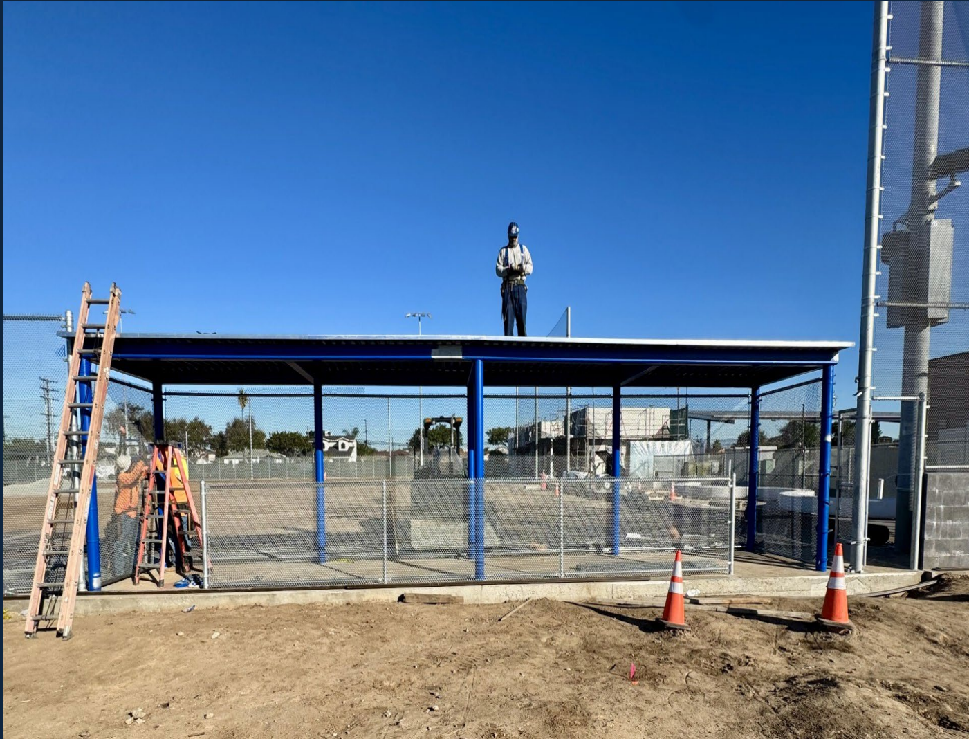
Dugouts Erected, Painted & Metal Decking Installed
