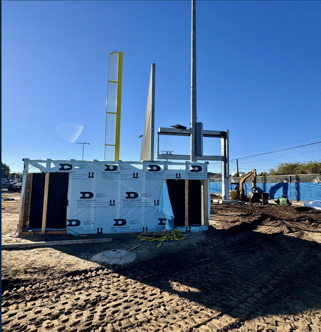
Digital Marquee Ready for Installation
