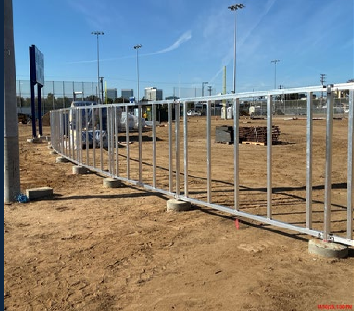
Removable Outfield Fence Was Test-Fitted on Both Ball Fields
