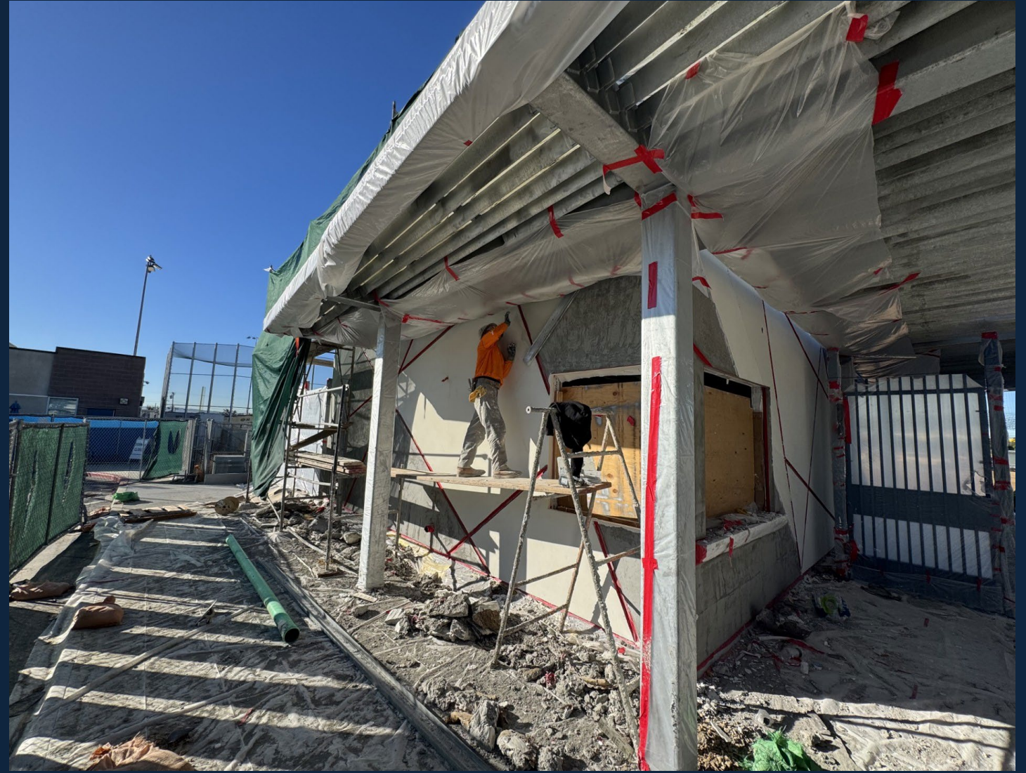
Color Coat Installation in Progress
