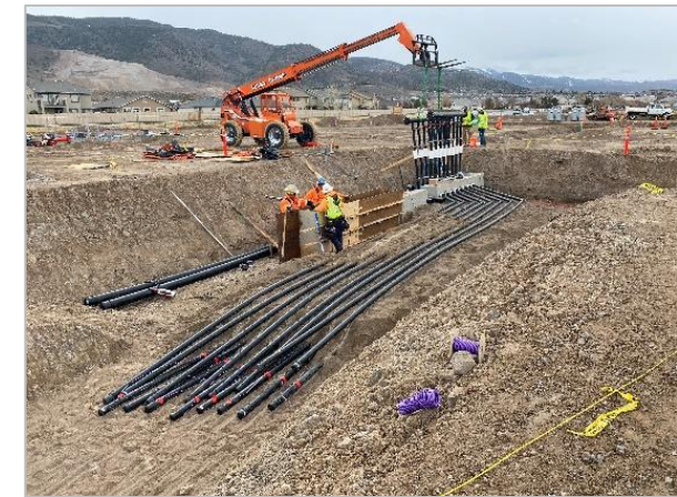
Construction of JWood Raw Geothermal Loop
