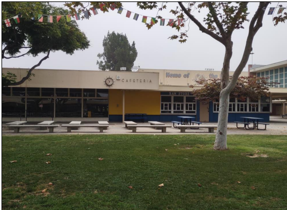
Figure 4. Cafeteria, west elevation facing quad
