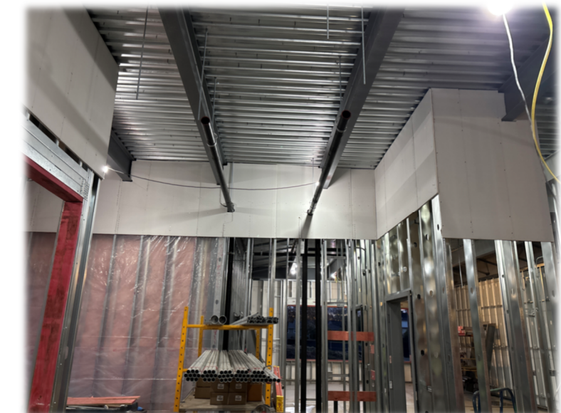
Windermere UPK Interior Drywall
