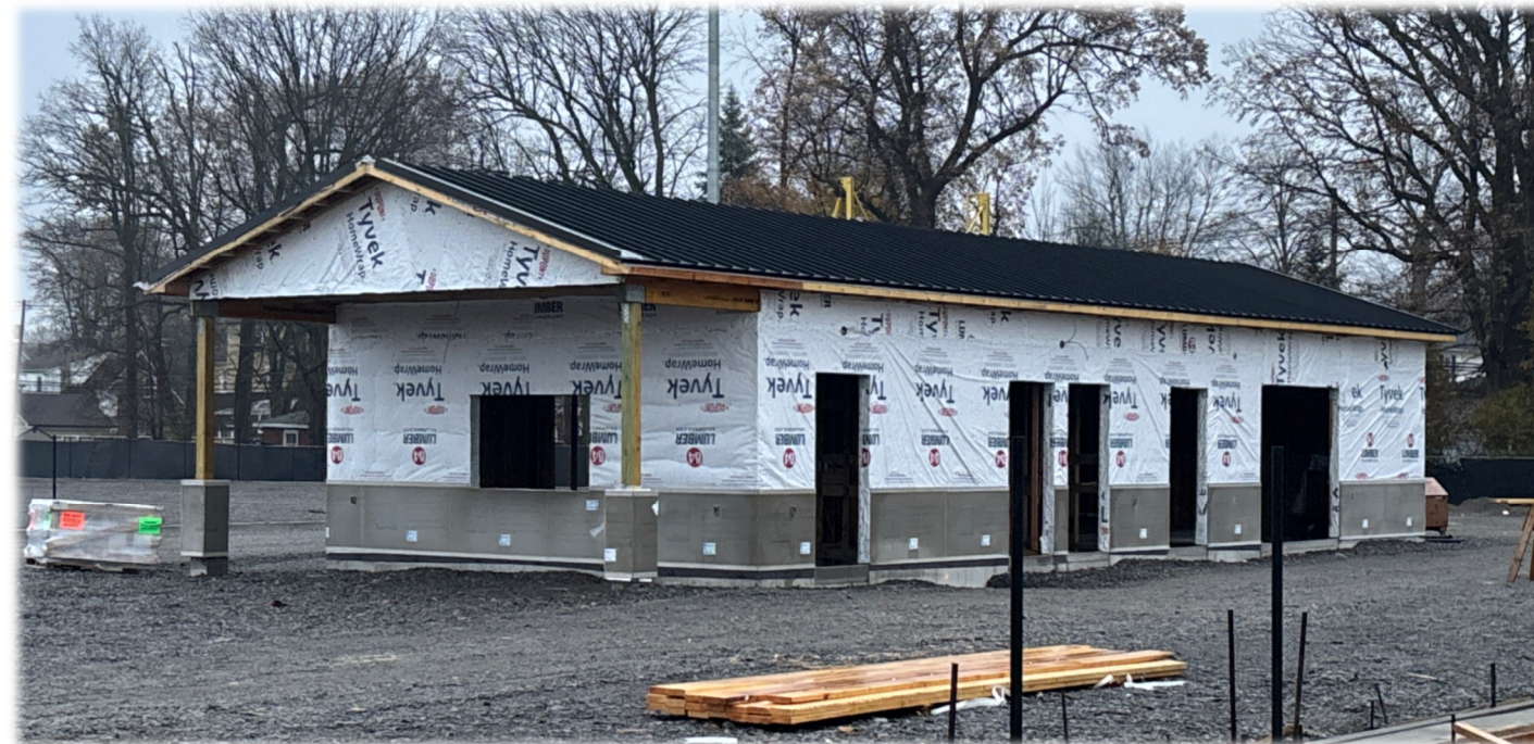
Exterior Waterproofing and Metal Roofing at the Concessions Building
