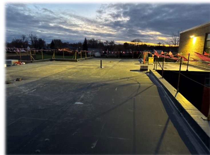
Windermere UPK Roofing
