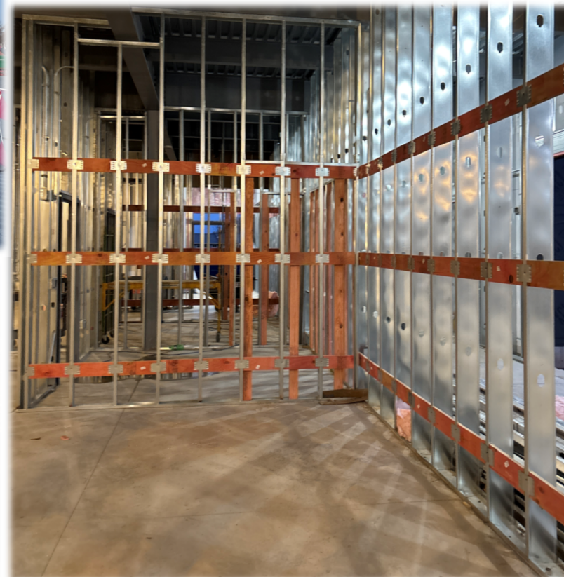
Windermere UPK In-Wall Blocking
