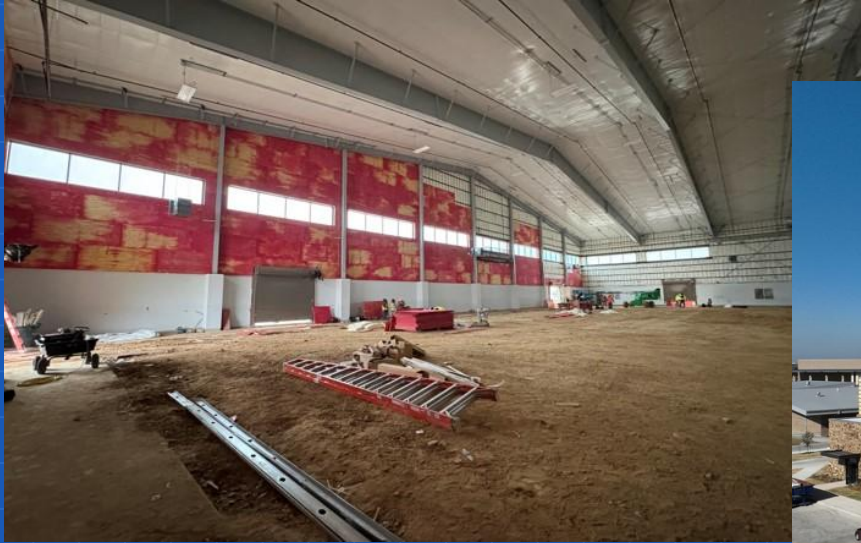
Installing plywood on the walls of the indoor activity center
