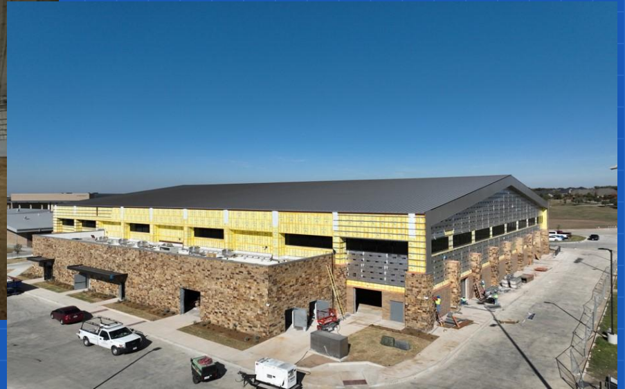
Exterior metal wall panel installation
