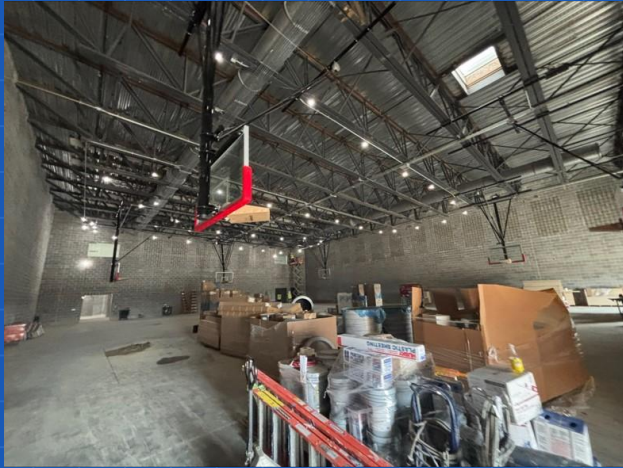
Gymnasium - preparing for block fill and paint
