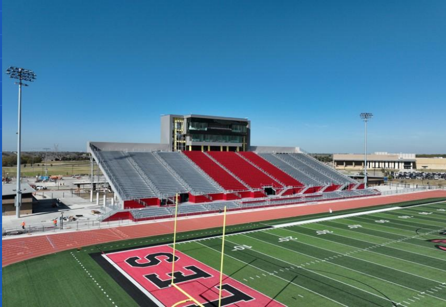
Stadium seating installation ongoing
