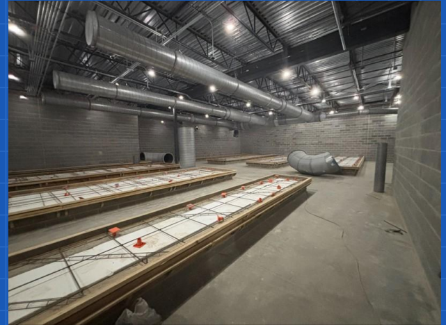
Locker room - preparing to pour concrete benches
