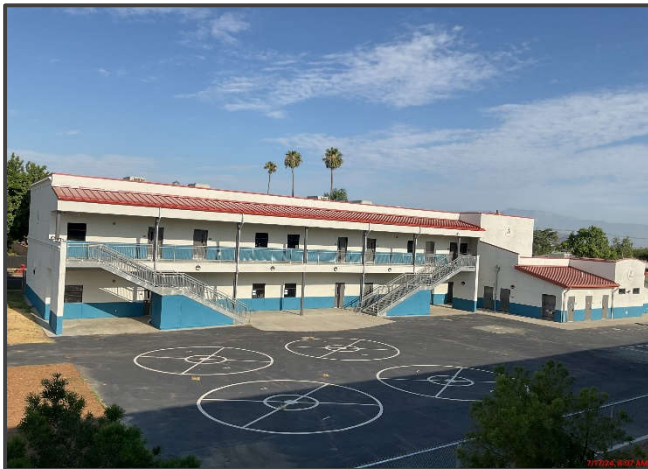
Library building repainted
