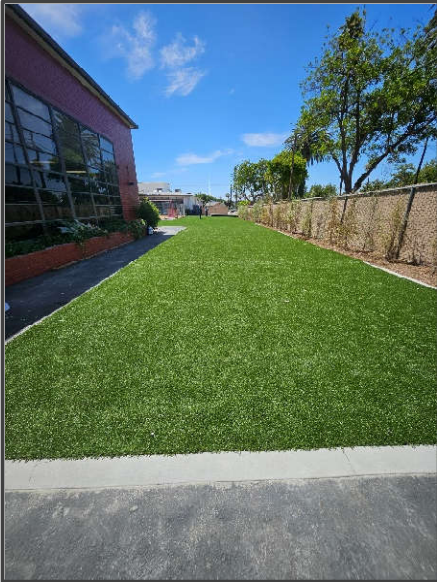
Turf Installation – Bldg. A
