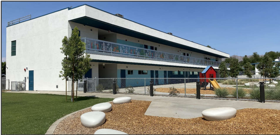
New 2-Story Classroom Building
