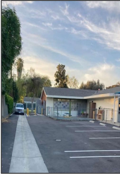
New Electrical Service
