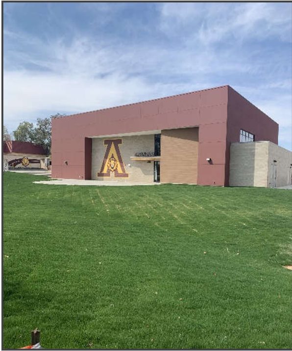
Exterior Auxiliary Gym
