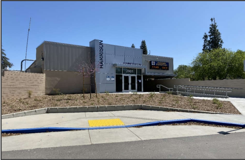
Completed Administration Building
