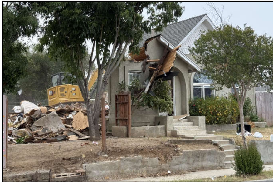
Eastside – Demolition of residential structure
