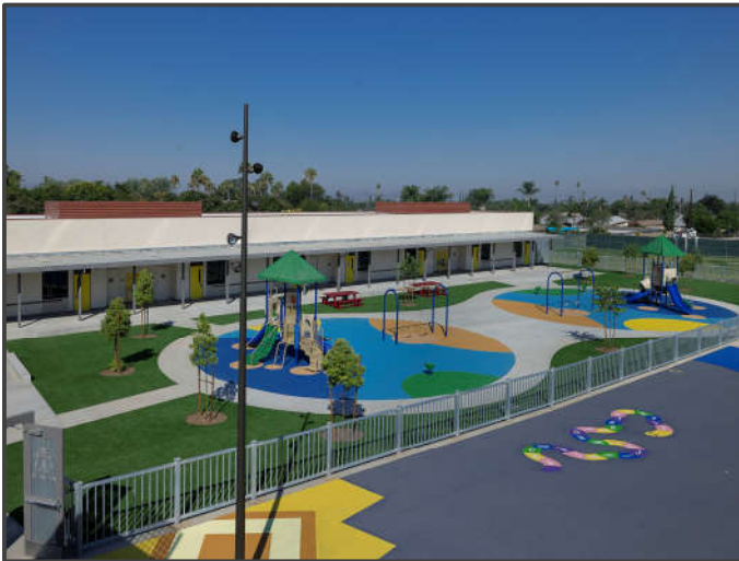
Building C & Kindergarten Playground
