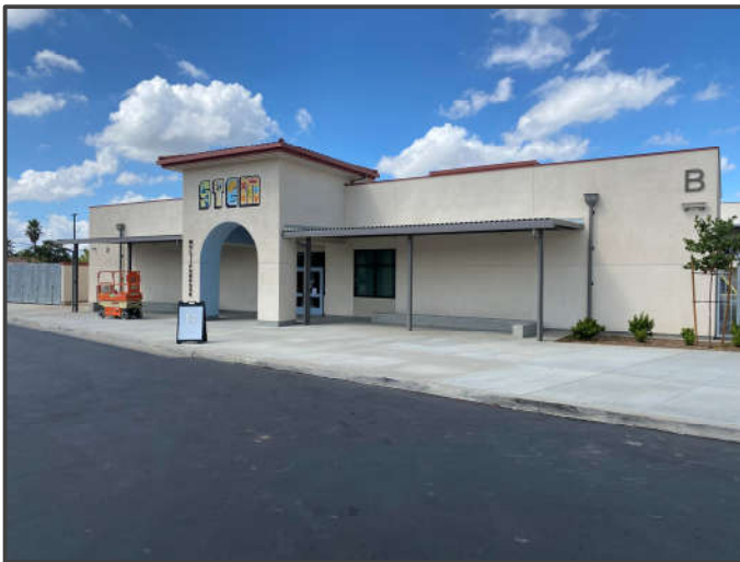
MPR – Building B
