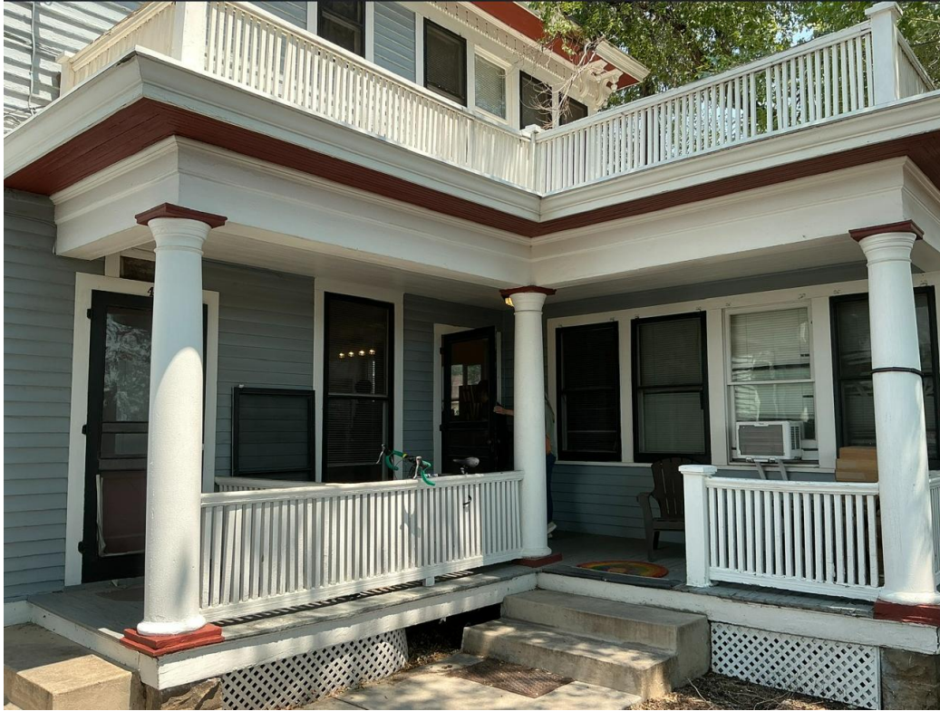
South single story porch detail at early addition
