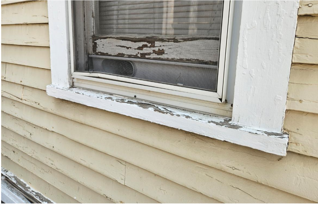
Window condition detail showing aluminum storm windows
