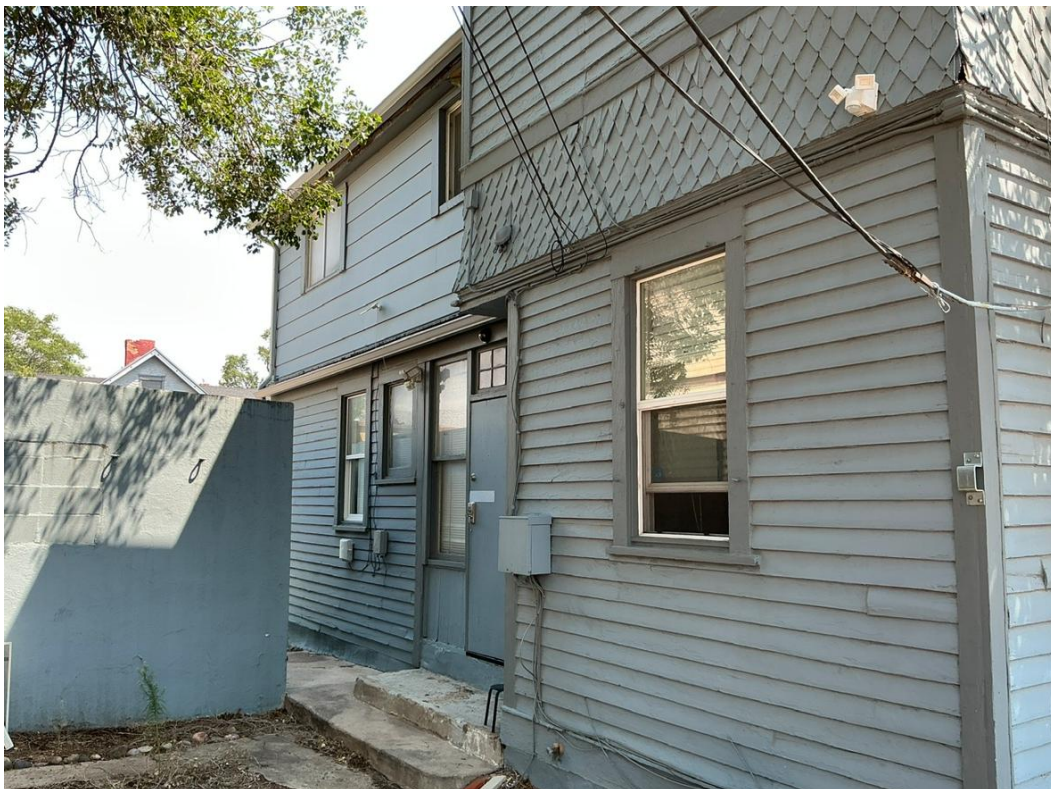
West façade - showing detached garage, 1900s and mid-century additions
