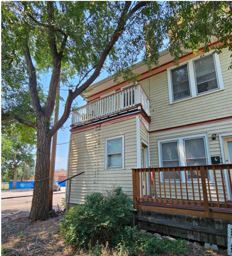
East façade – partial showing vinyl siding below with clapboard siding above
