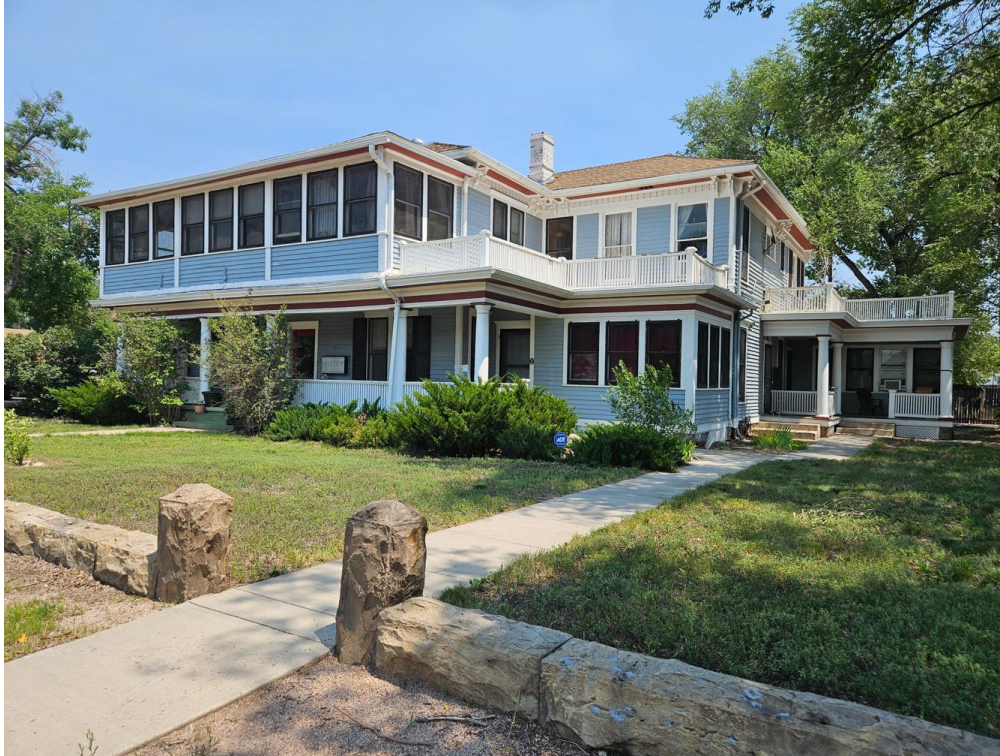
South/West façade – note original low stone wall present along Nevada and St. Vrain
