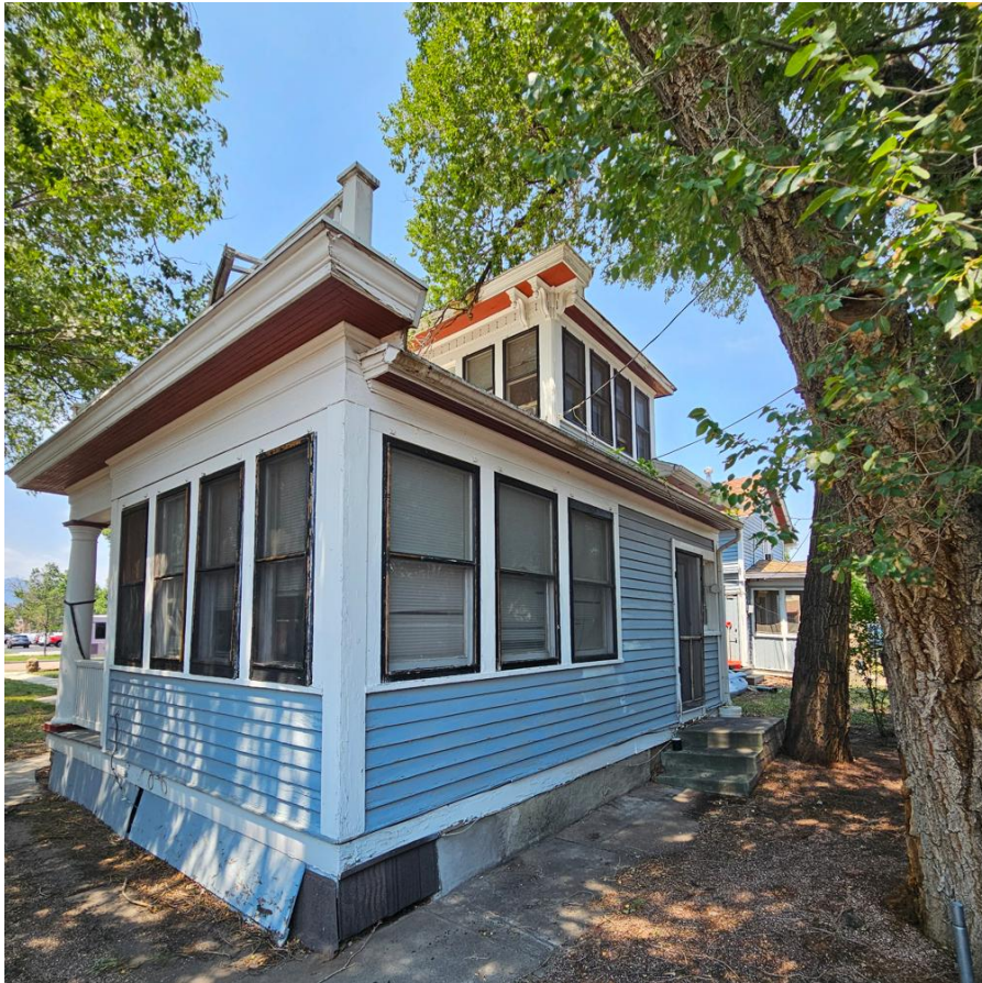
South east corner at early addition
