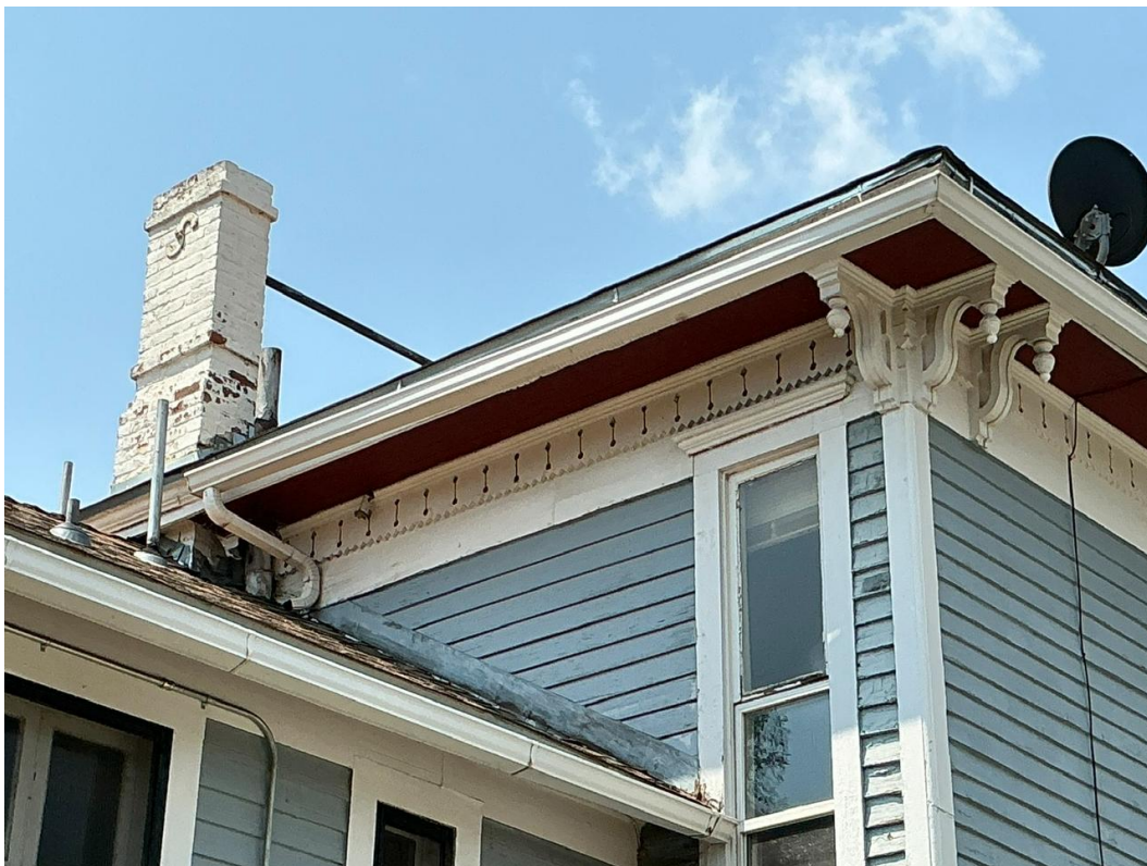
Condition detail at original kitchen chimney (1 of 3 chimneys)
