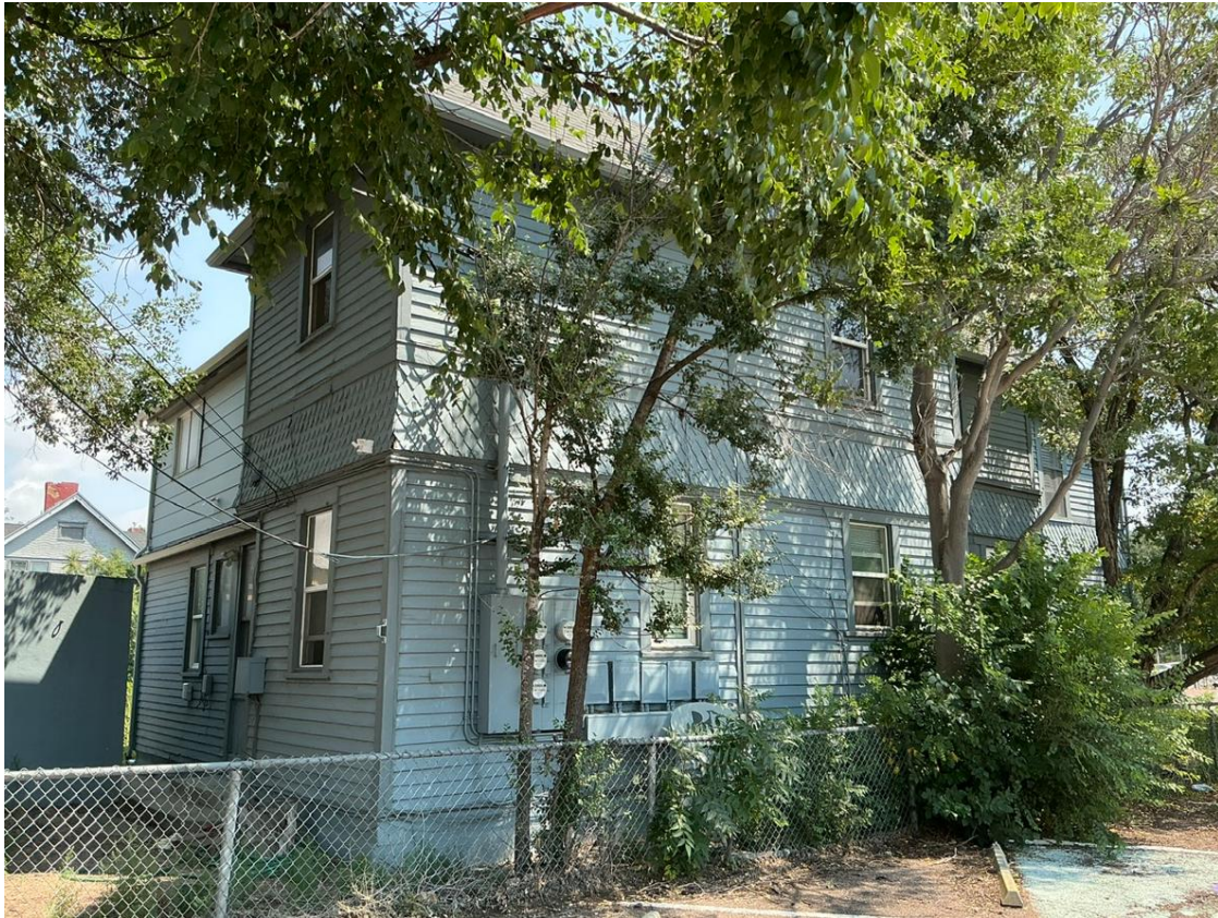
South West façade – showing 1900s two story addition to the original structure
