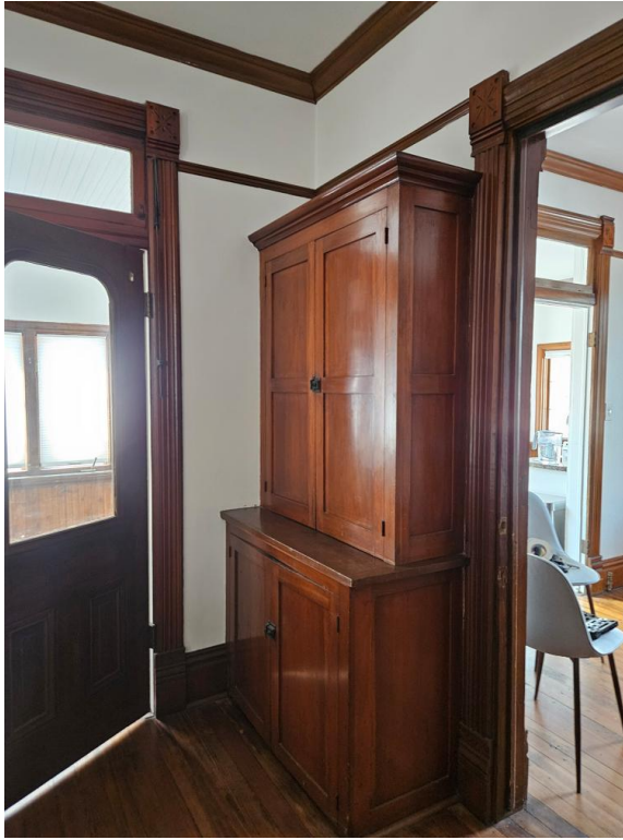
Interior built-in casework details
