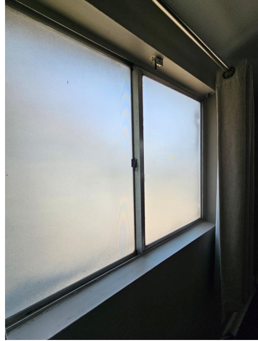
Aluminum windows at mid-century addition
