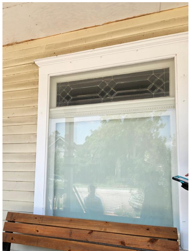
Window Detail at North Façade
