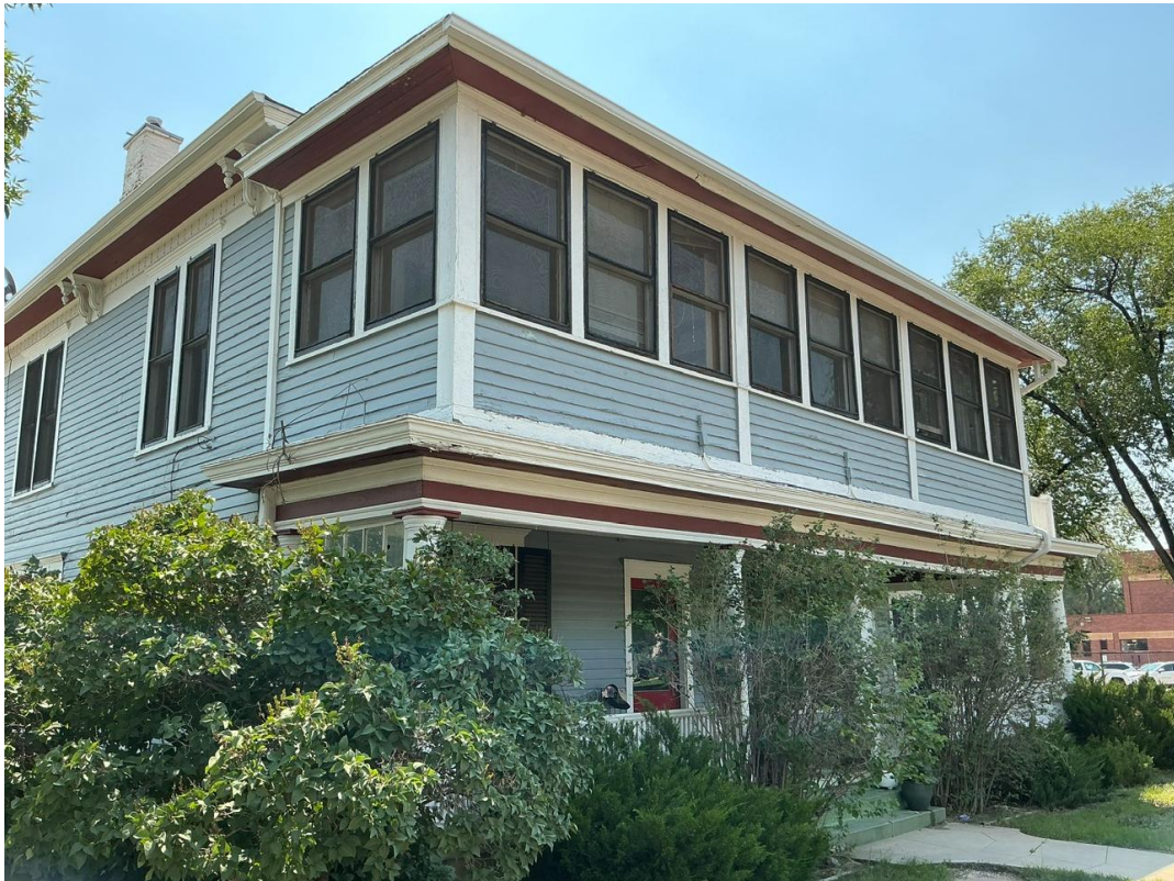
View of “sleeping porch” enclosed shortly after construction
