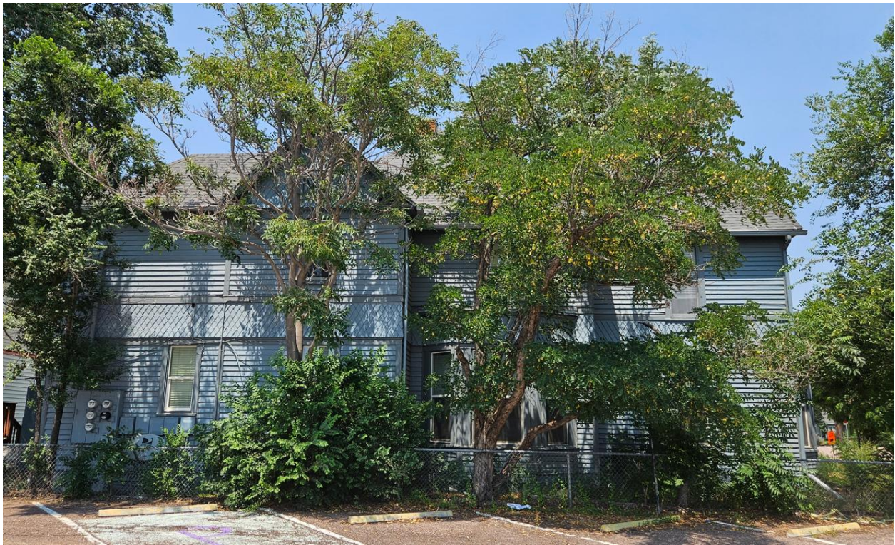
South façade from Palmer High School parking lot
