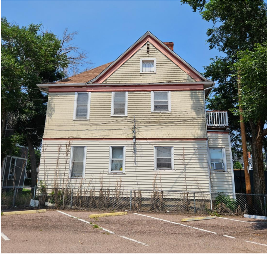
South façade - showing vinyl siding at lower level
