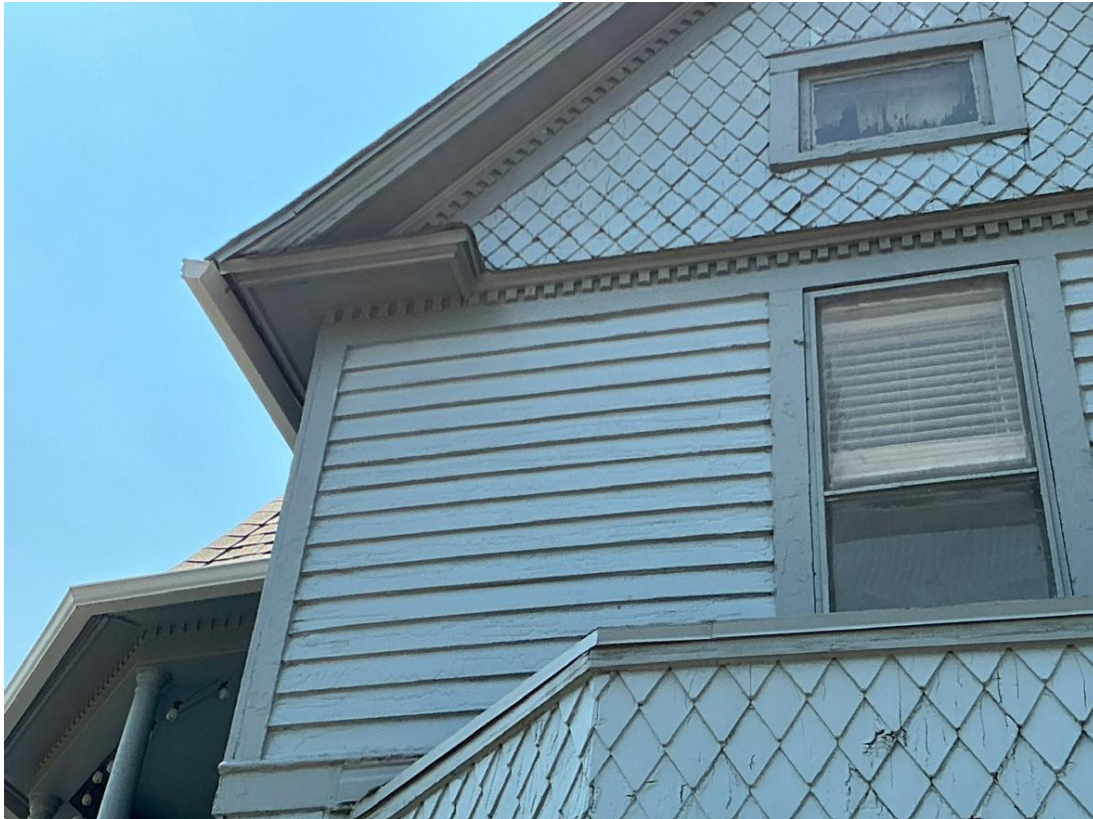
North façade detail
