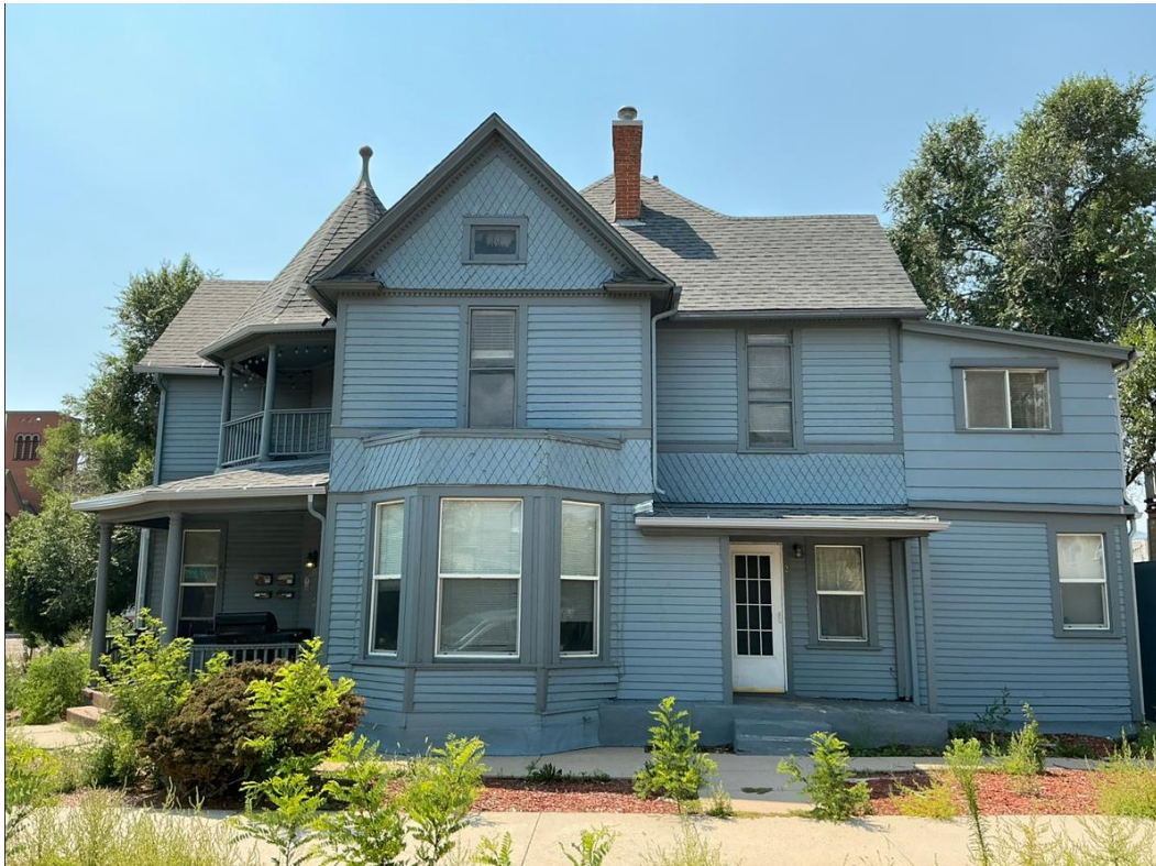
North façade - addition to the west estimated to have been constructed post WWII to 1967 based on aluminum single pane sliding windows and presence of addition in 1967 photography
