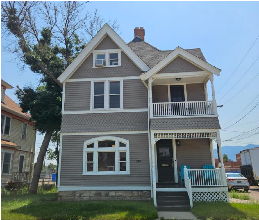
North primary façade
