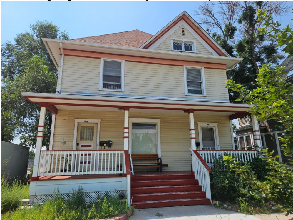
North primary façade
