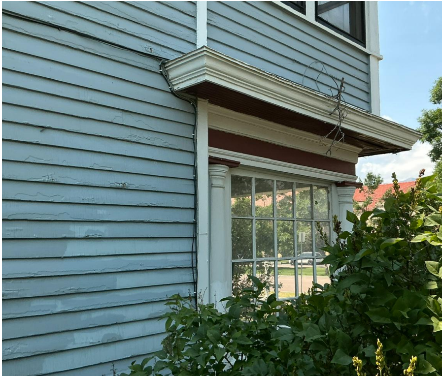
Condition detail at north facade
