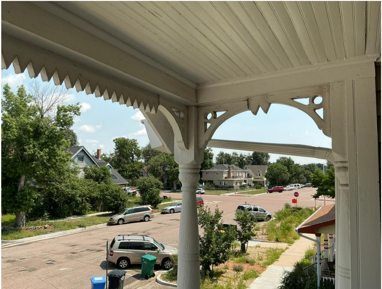
Detail at upper north balcony
