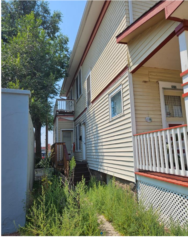
East façade – partial showing vinyl siding and replacement porch detail
