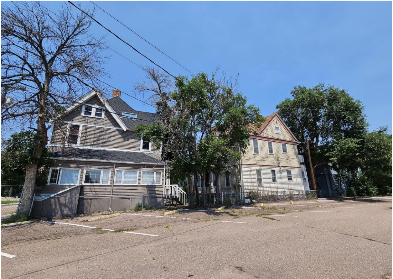
View of properties from Palmer High School parking lot looking north
