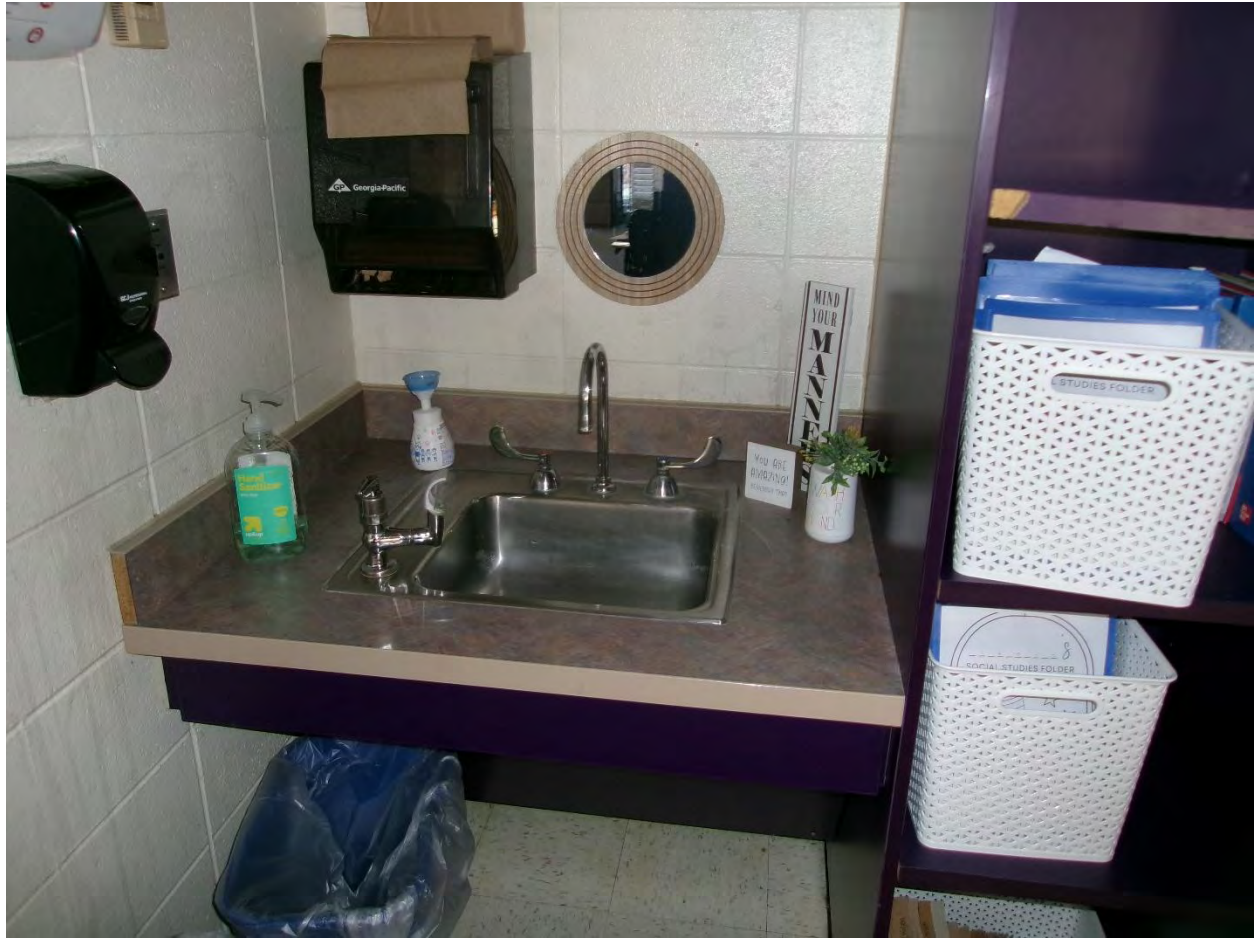
Westfield Intermediate School 17710 Shamrock Boulevard Westfield, Indiana Ground Floor-1988/1990's Construction Stainless Steel Sink Insulation No Asbestos Detected
