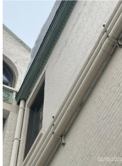
Exterior side C soffit inaccessible
