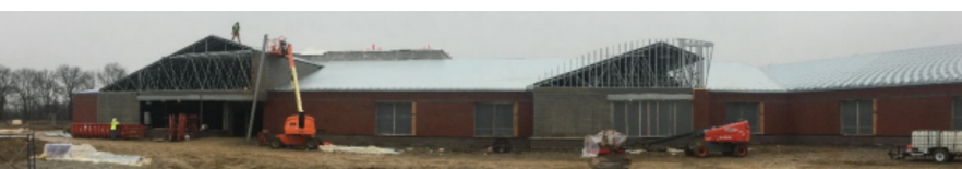
Winter 2019: Prairie Run Elementary getting under roof
