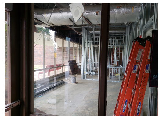
Big changes at Hylen Souders Elementary with the addition of the new lobby
