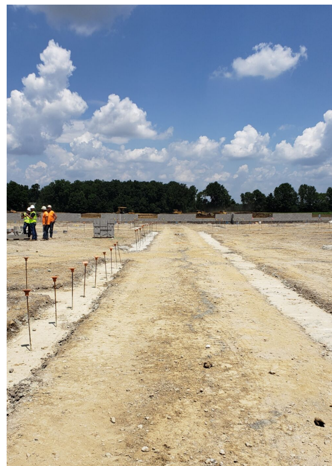
The view standing in elementary cafeteria looking north, down central classroom corridor
