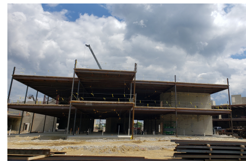
Watching the 3-floor classroom wing being built at the new high school
