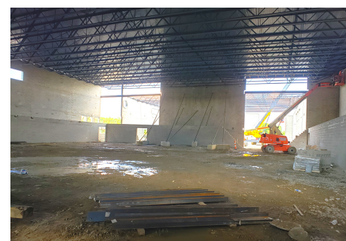
Looking inside the new high school competition gym
