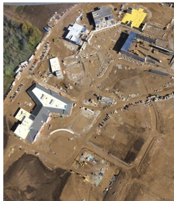
Aerial view of the joint construction site
