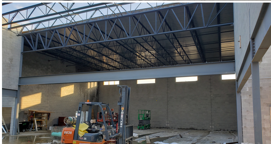
PRE view from student dining into the gym—the beam will support a movable partition wall
