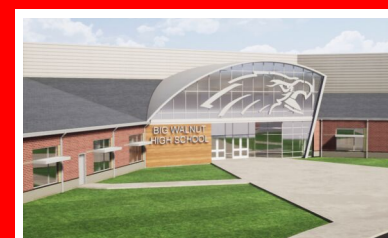
New High School: https://www.vswc.com/bwhs/
