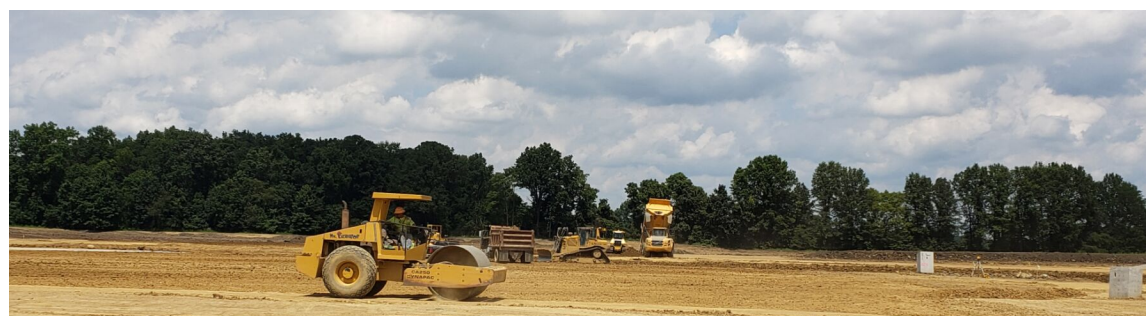
Preparing the ground to start the high school building
