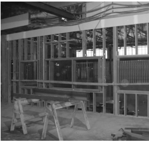
The cafeteria features that overlook the gymnasium.
