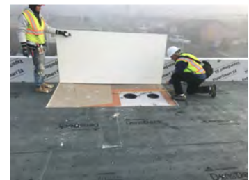
Installing the roof underlayment
