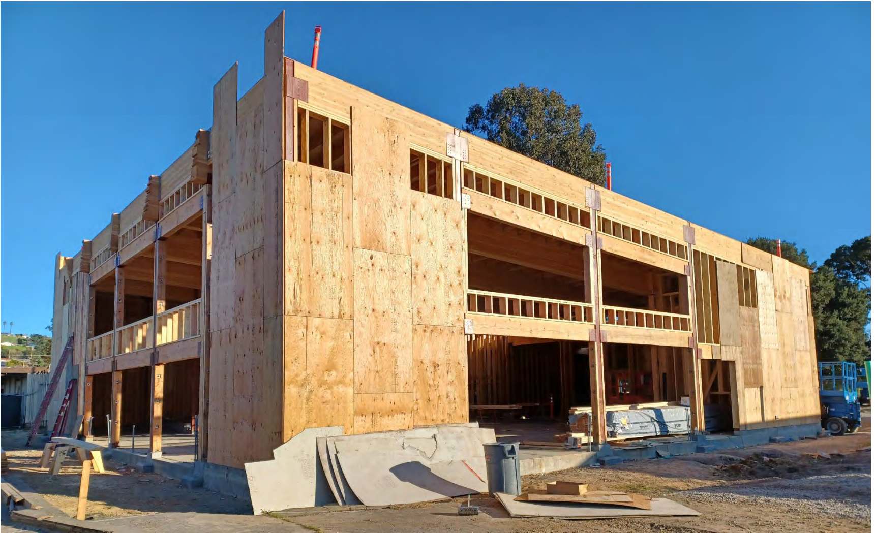
Sheathing on the main dining area
