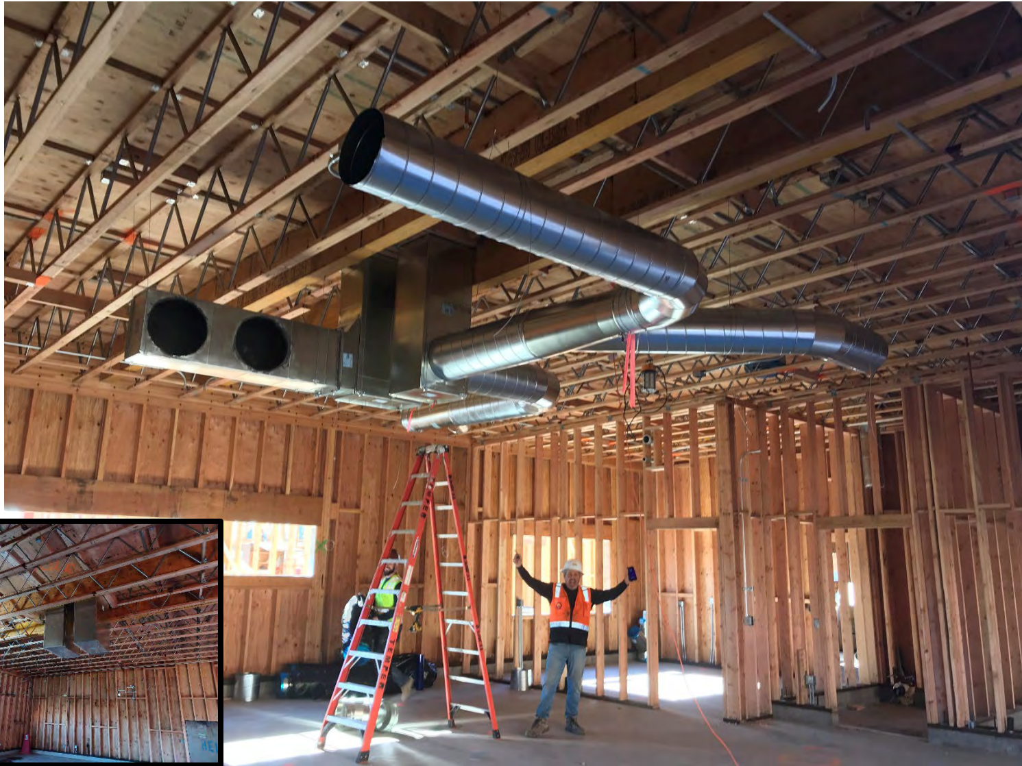
Building F – Ductwork installation
