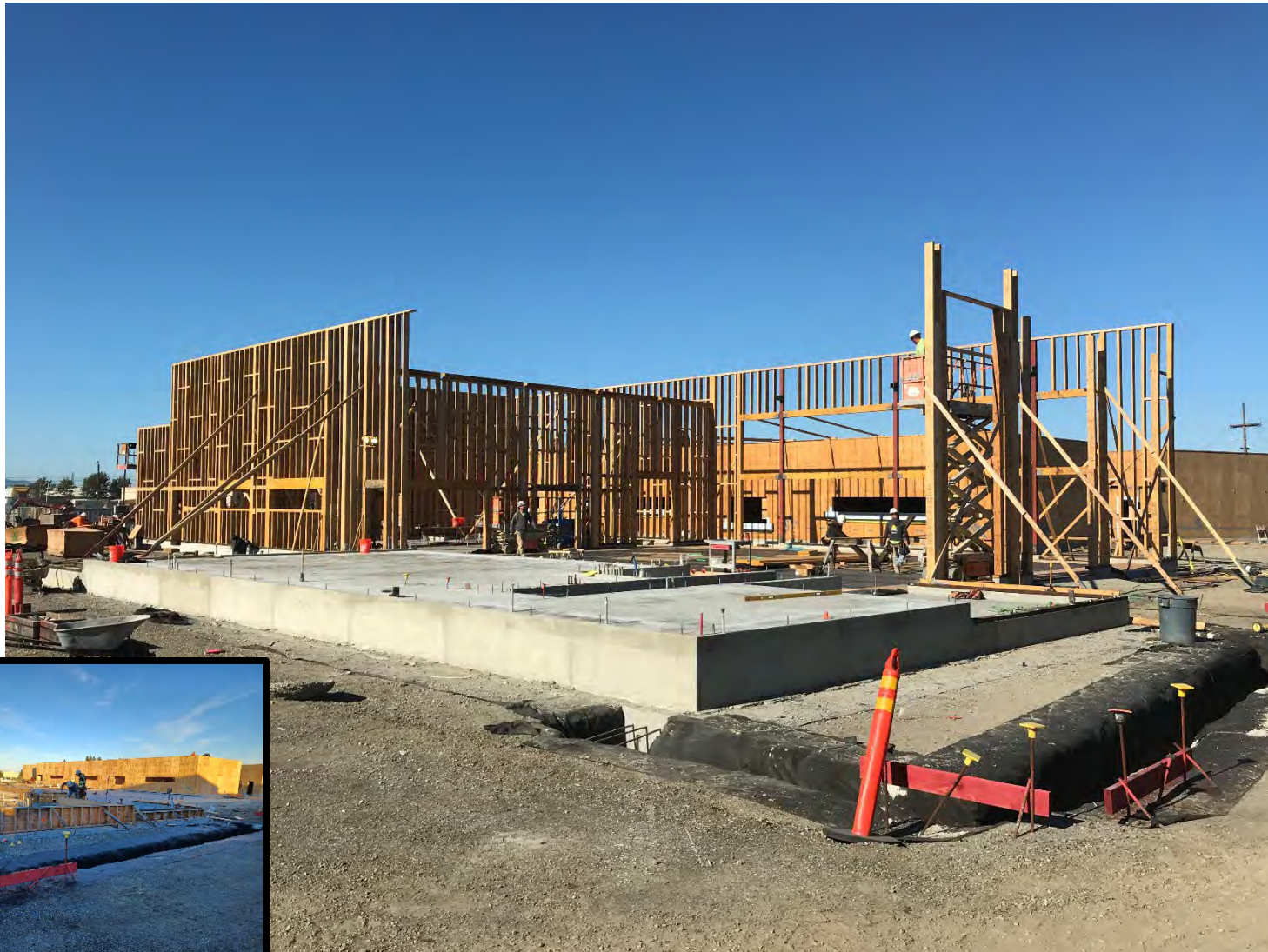
Building D – Framing
