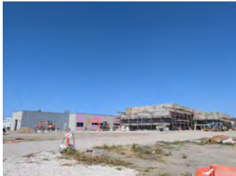
Building E (Kinder) and Building D (Cafeteria) Final Stucco Coat on building E and rough coat on building D
