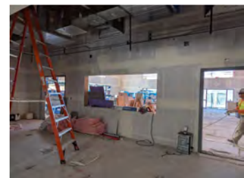
Gypsum Board Installation
