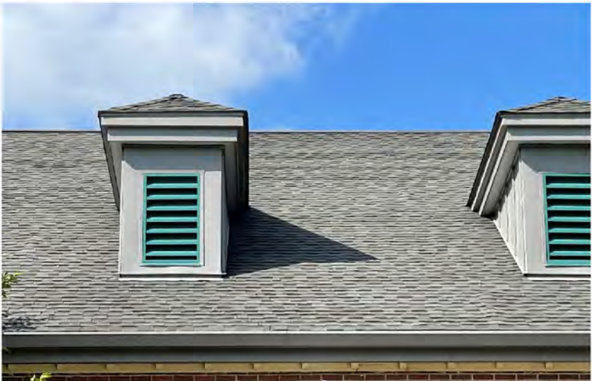
AE-52: Typical asphalt shingled roof and dormer assemblies.
