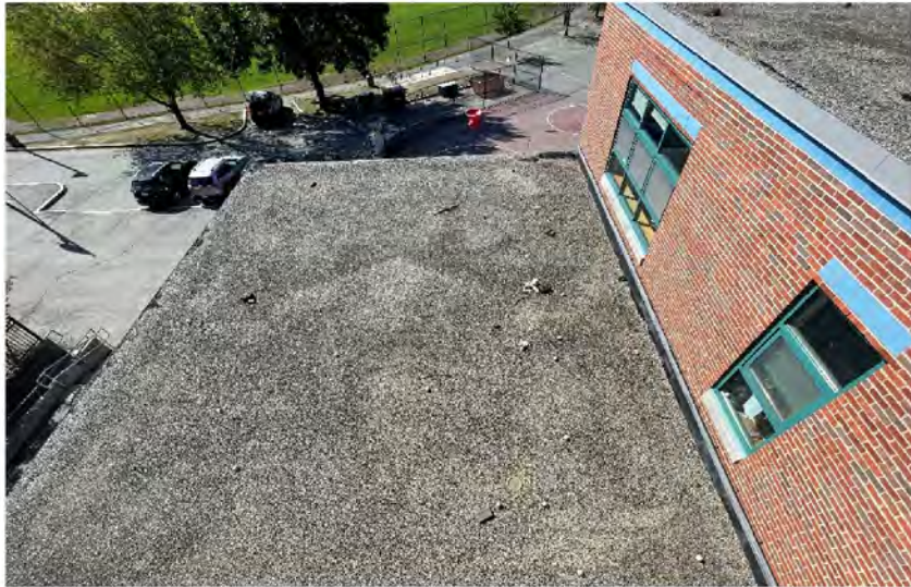
AE-45: View of low roof at Southeast corner of building
