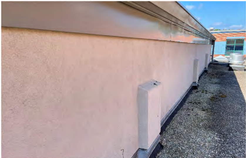
AE-27: Representative stucco façade above roof
