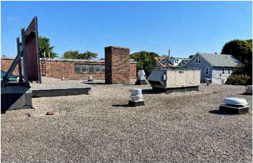
AE-42: Representative view of roofing at West side of building
