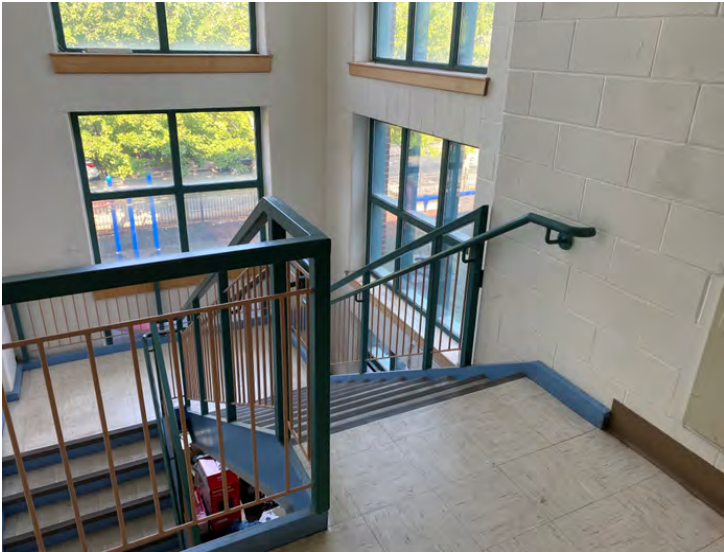
Typical Egress Stair
