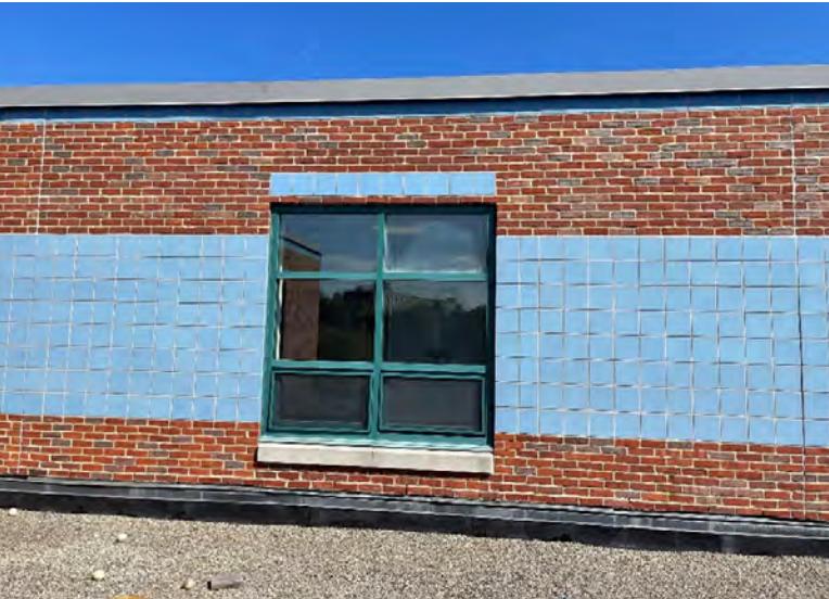
AE-C: Representative masonry façade and aluminum window assembly above the roof
