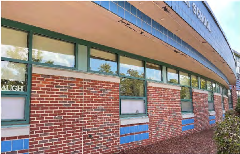
AE-9: Representative brick veneer, precast bands and aluminum windows
