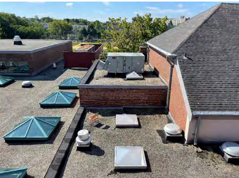
AE-D: Representative roof condition at intersection of buildings from different eras of construction
