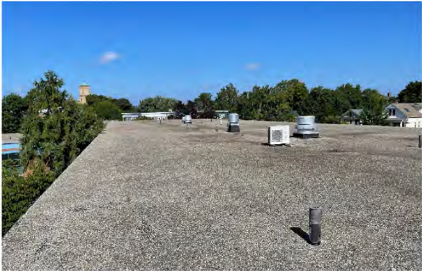
AE-46: View of roof along North end of building
