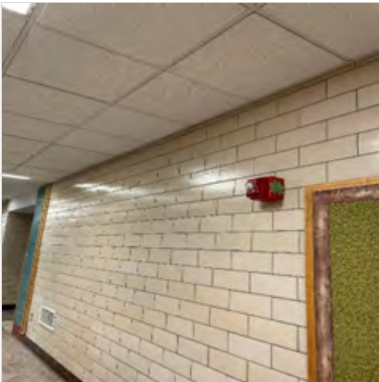
E-5: Existing Fire Alarm Device
