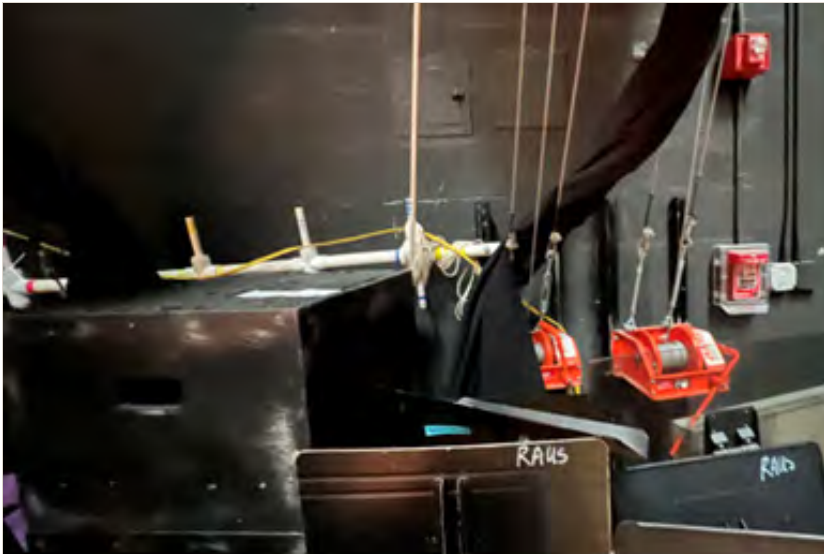
Existing Hand Winches and Makeshift Pinrail
