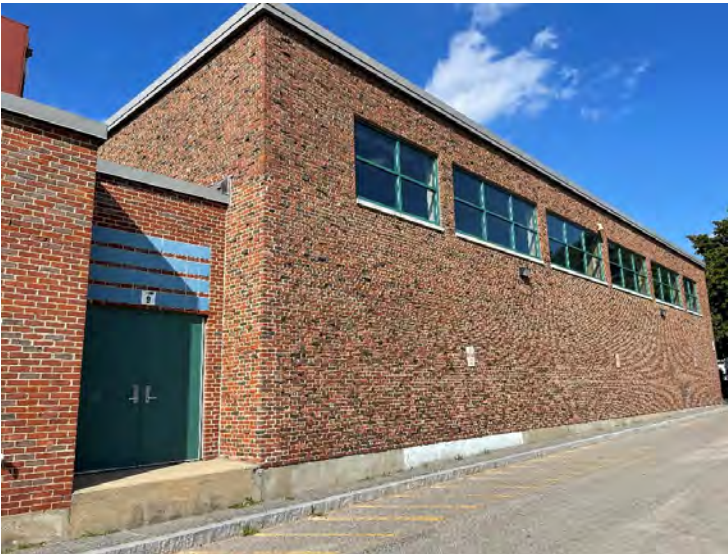
AE-B: East façade at older portion of building
