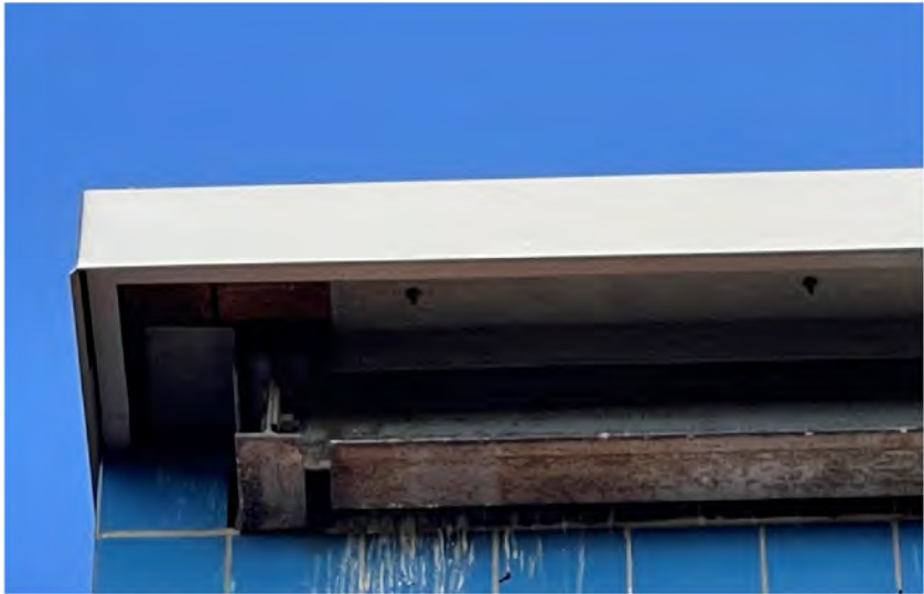
AE-33: Exposed steel beams on West Elevation
