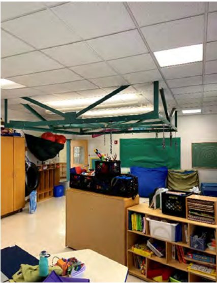
Photo ST-8: Hanging steel structure at OT/PT room
