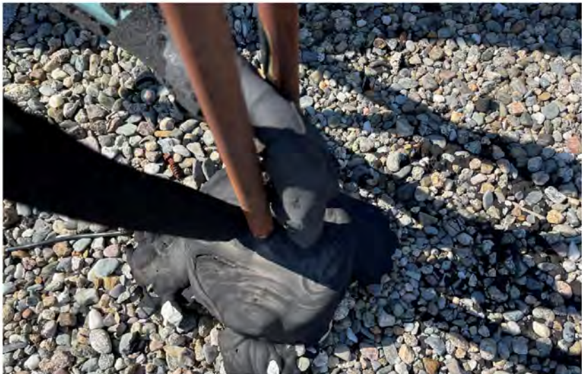
AE-51: Typical pitch pocket with pourable sealer.
