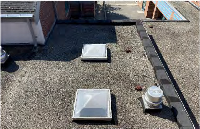
AE-44: General view at center of roof, typical unit skylights.
