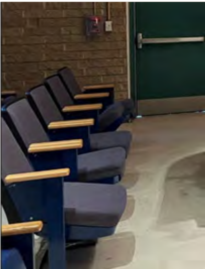
Auditorium Seating with Inoperable Return
