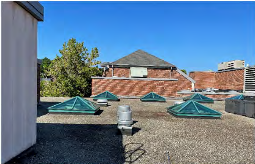
AE-43: General view of roof at center of West wing, typical metal framed skylights.
