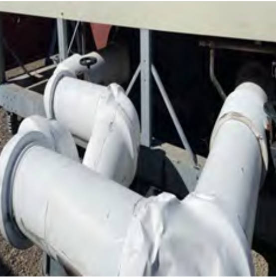
M-4: Chiller Piping Conditions
