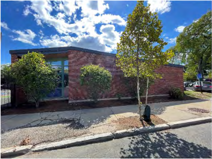
AE-7: North Elevation of E Wing
