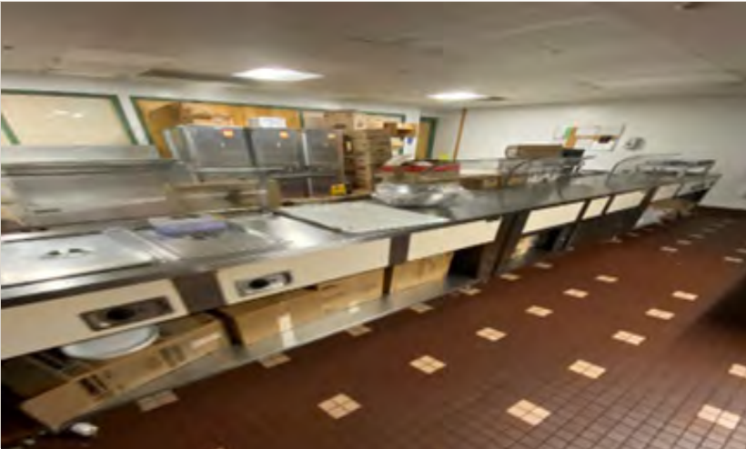
FS-1: The serving line is large enough for the school but does contain any refrigerated cold pans for safe display of cold food product at the proper temperatures.
