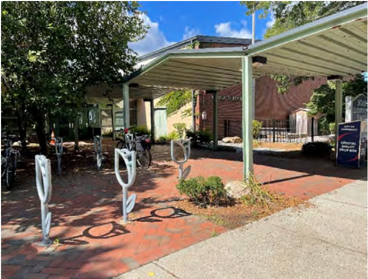
AE-A: Main Entrance at East Elevation of D Wing
