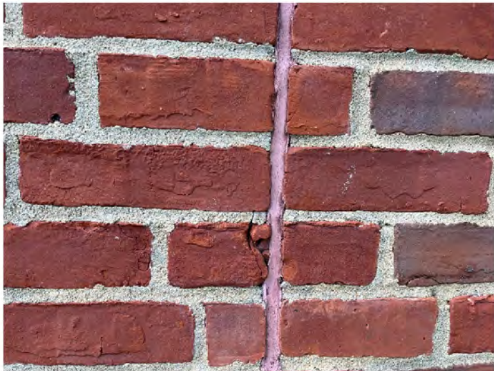
AE-24: Representative failing masonry control joint sealant
