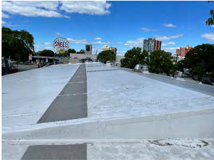
AE-54: Representative PVC roofing assembly
