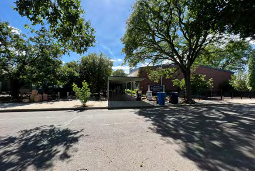
North side - Front Entrance
