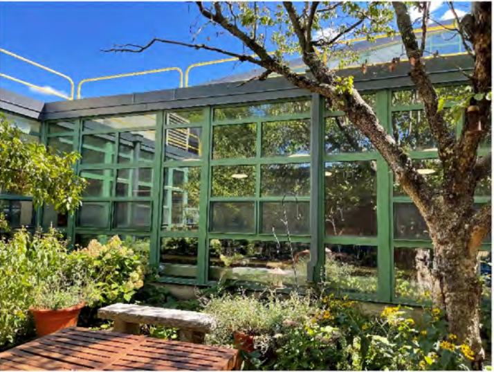
AE-12: Façade within Courtyard
