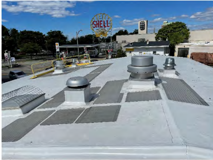
AE-56: Representative PVC roofing assembly with MEP units and unit skylight
