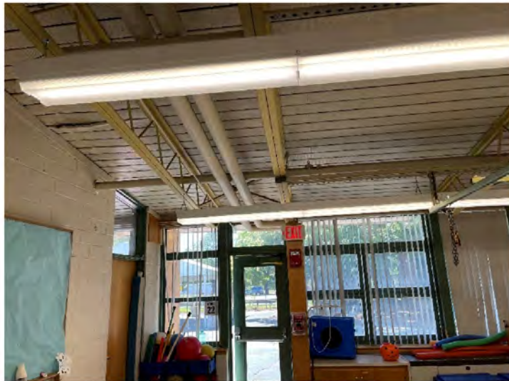
AE-23: Interior of typical classroom where roof trusses extend through facade.
