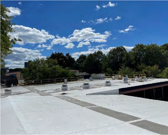
AE-D: Representative recently installed PVC roof
