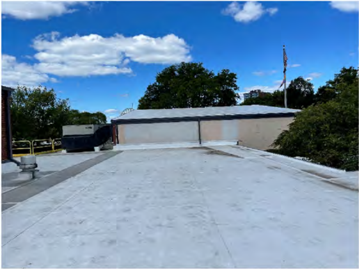
AE-55: Representative PVC roofing assembly
