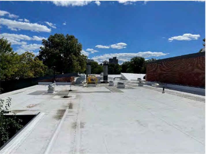
AE-58: Representative PVC roofing assembly
