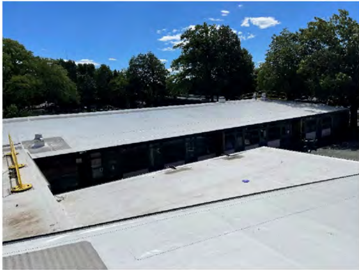
AE-57: Representative PVC roofing assembly
