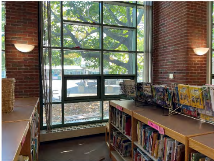
AE-40: Interior of curtain wall within Library
