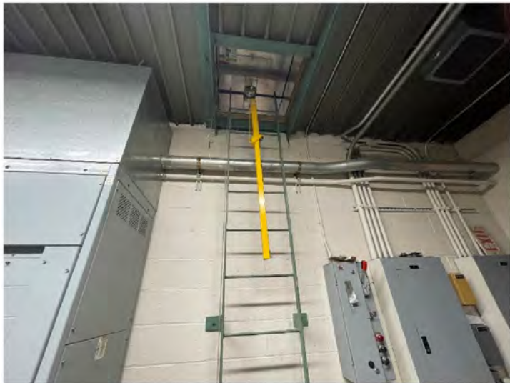
AE-67: Interior of wall mounted ladder at roof access hatch
