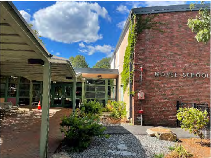
AE-4: East Elevation of D Wing at Main Entrance
