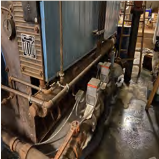
M-1: Mechanical Room Conditions
