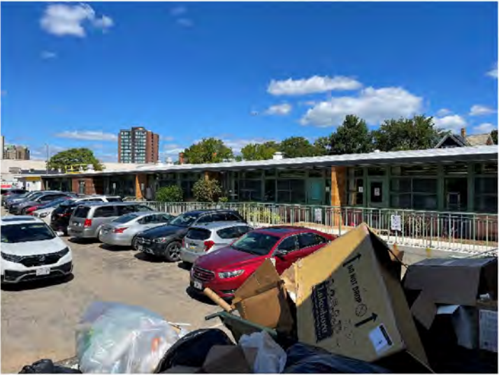
AE-11: West façade at E Wing
