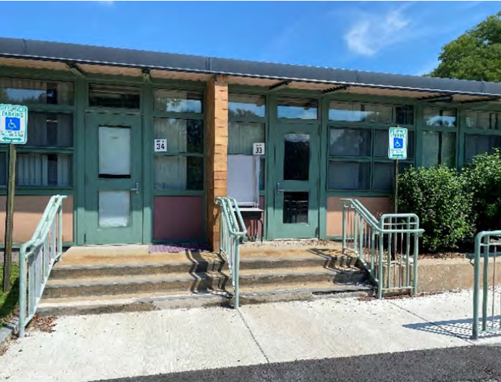
Exterior Egress Stairs
