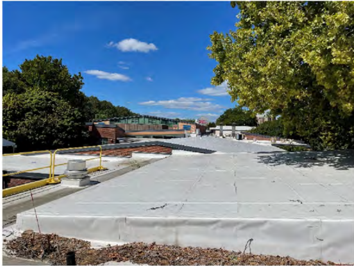
AE-59: Representative PVC roofing assembly
