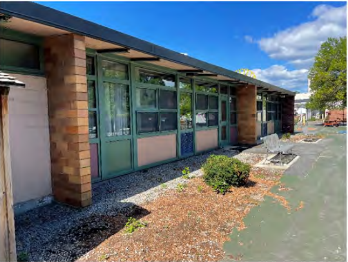
AE-10: Typical East façade at E Wing
