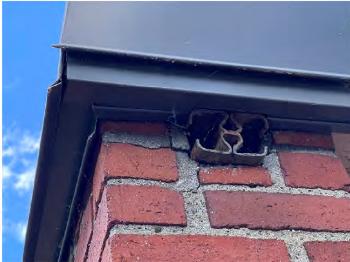
AE-22: Typical exposed metal roof truss at exterior of facade
