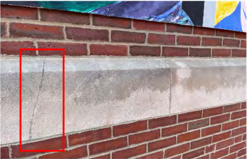
AE-13: Representative cracked limestone band
