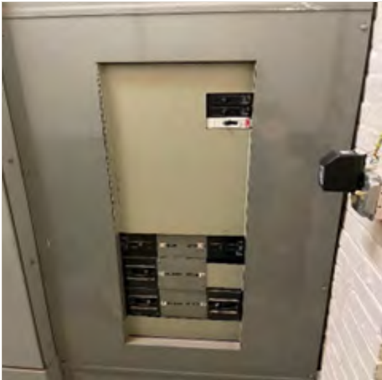
E-2: Existing ~1962 (Not replaced in 1982 Renovation)
