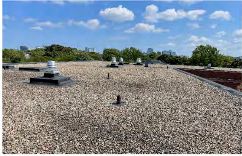
AE-27: Representative view of roof: Roof is ballasted EPDM
