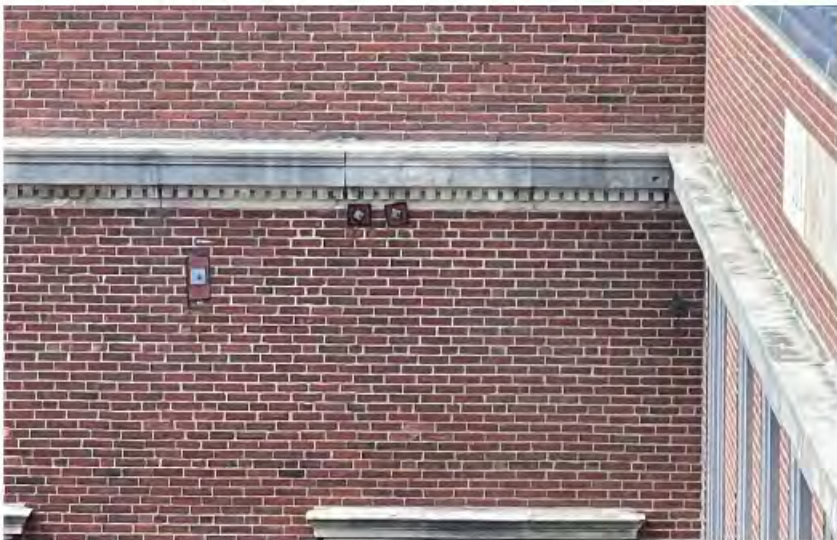
AE-8: Representative façade with tie backs
