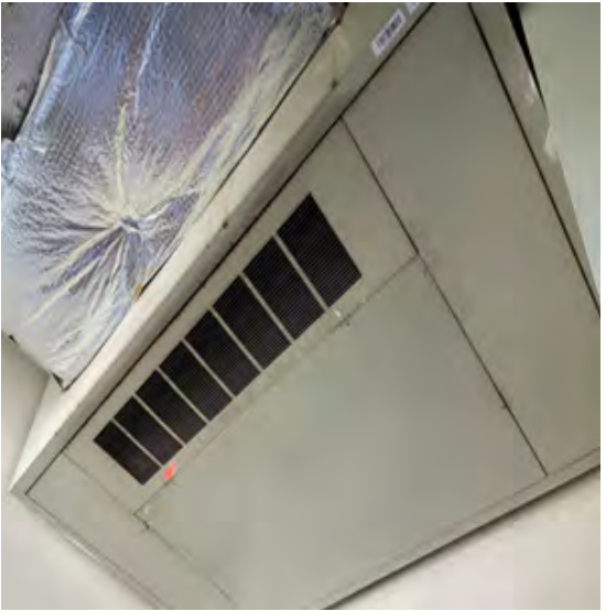
M-4: Fan Coil Unit Condition
