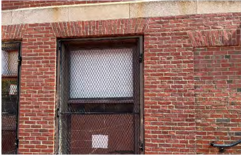
AE-21: Representative aluminum window. Note most lower level windows have security grilles.
