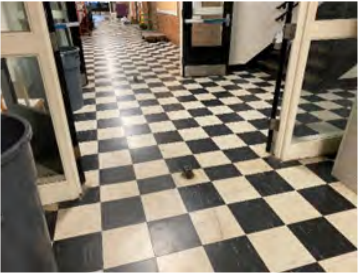
Center Stair Doors at Basement Level
