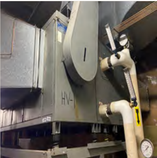
M-3: Air Handler Condition
