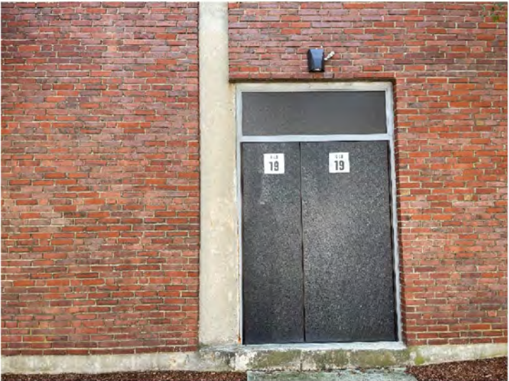
AE-38: Typical metal door assembly at exterior
