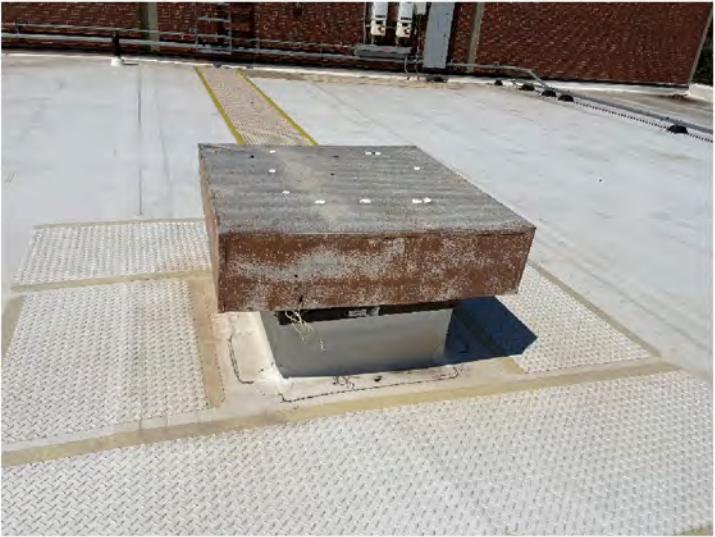
AE-56: Typical vent curb with walkway pads
