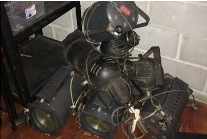
Obsolete Theatrical Lighting Fixtures
