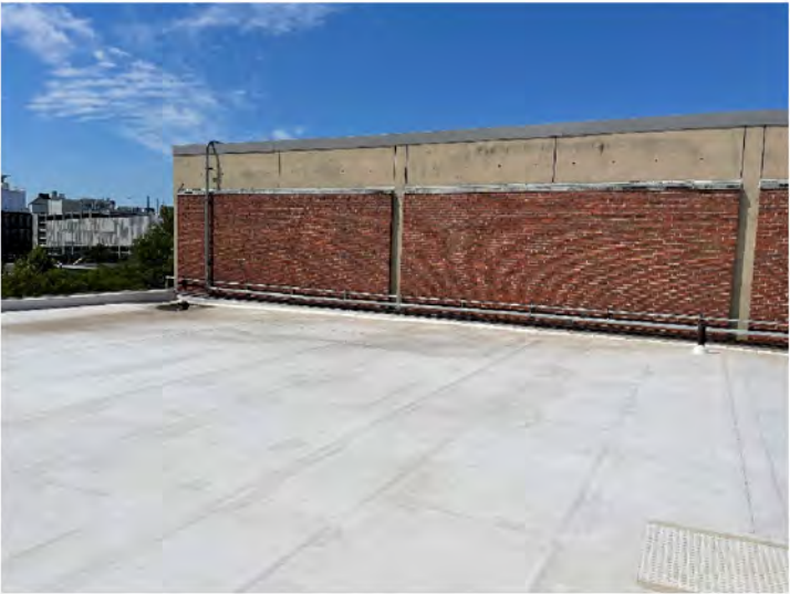
AE-49: Representative roof and façade area
