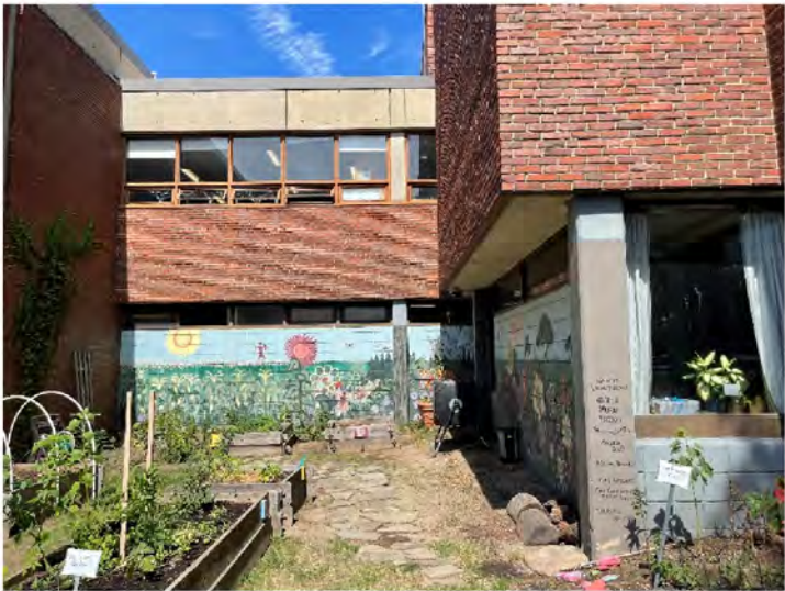
AE-7: Typical façade condition at lower level where concrete block provides façade infill between structural concrete elements.
