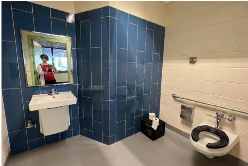
New restrooms 1st Floor
