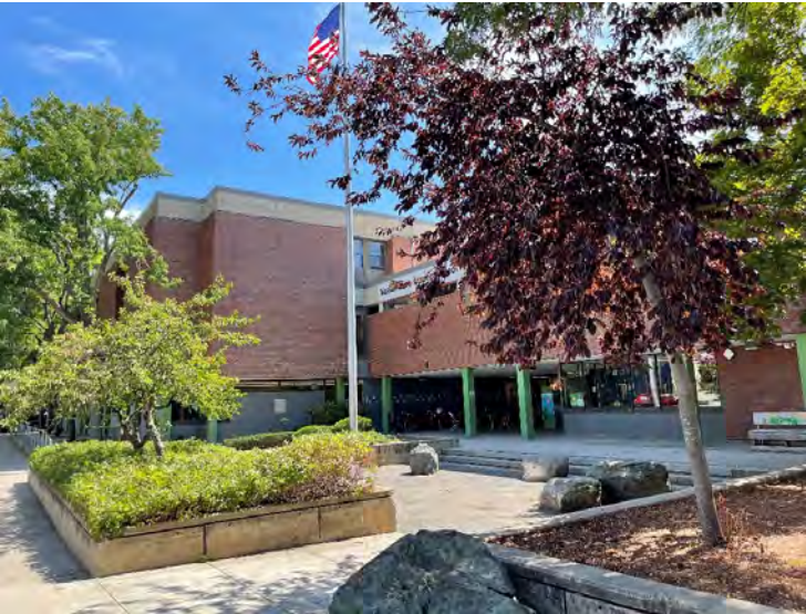
AE-A: Typical façade area at main entrance
