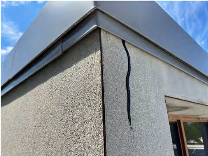
AE-21: Typical sealant application on crack in cementitious cladding at roof monitor.
