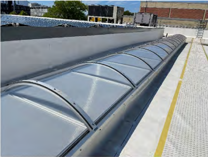
AE-48: Exterior of long unit skylight
