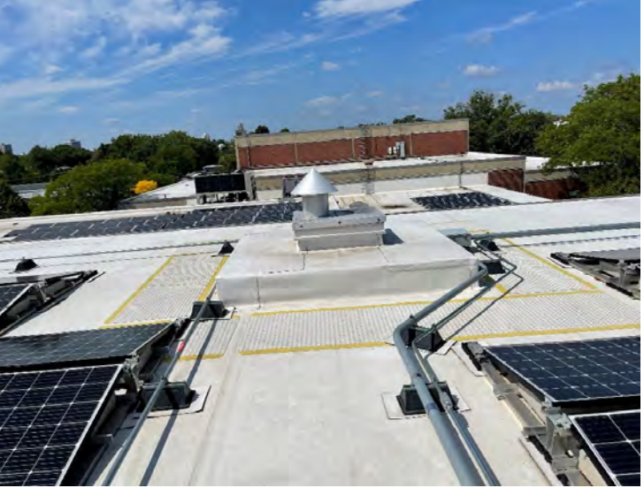
AE-D: Representative newly installed TPO roof
