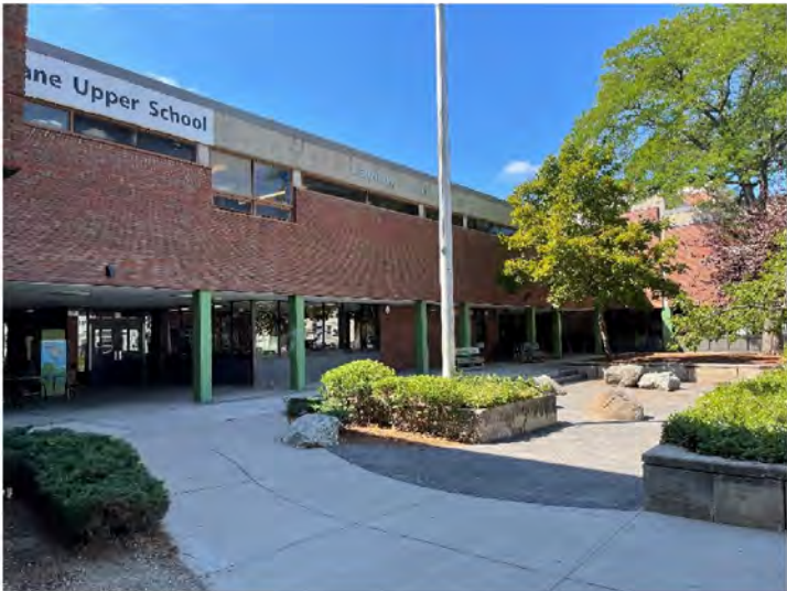
AE-2: Partial North elevation at main entrance
