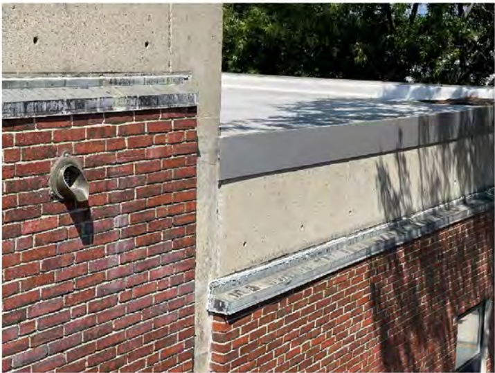
AE-13: Typical cast in place concrete structural elements and brick façade, with metal flashings along top of brick.
