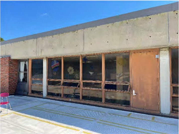
AE-27: Representative steel framed windows located above the roof.
