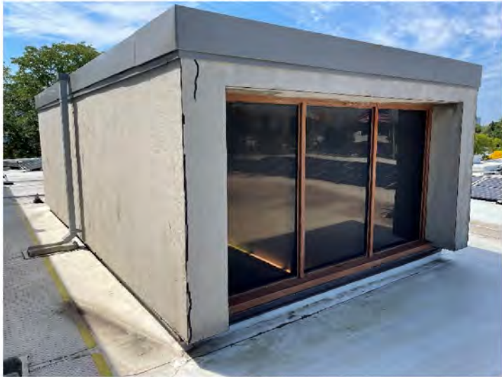
AE-20: Representative roof monitor with metal framed windows and clad with cementitious panels
