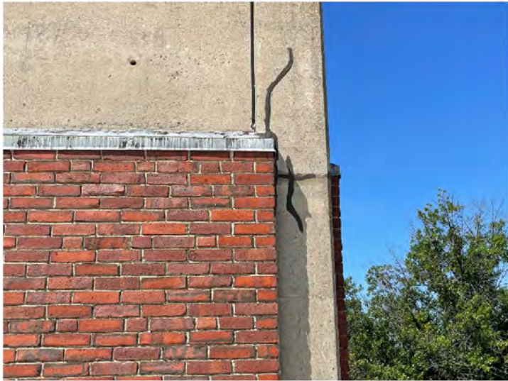
AE-18: Typical sealants applied over cracking in exposed cast in place concrete structural elements.
