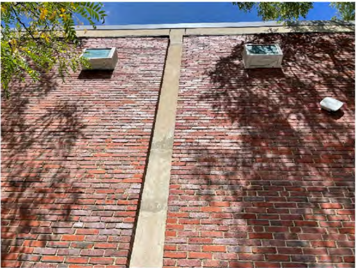
AE-8: Representative façade conditions with exposed cast in place structural concrete and brick infill facades.
