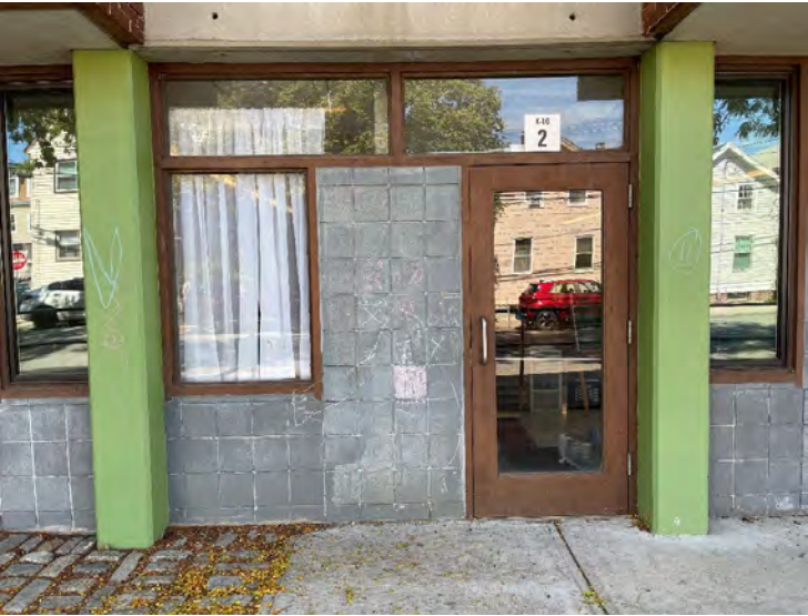
AE-C: Representative steel window and door assembly with concrete block façade at exterior of typical ground level classroom.
