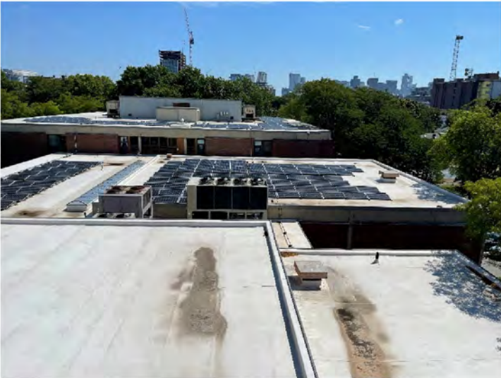
AE-43: General view of various roof areas comprising the school
