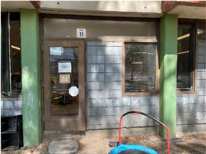
AE-37: Typical metal door with full glass lite in classroom condition
