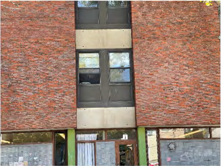
AE-6: Typical façade conditions with hung windows, exposed concrete floor at floor slabs and brick masonry veneer.
