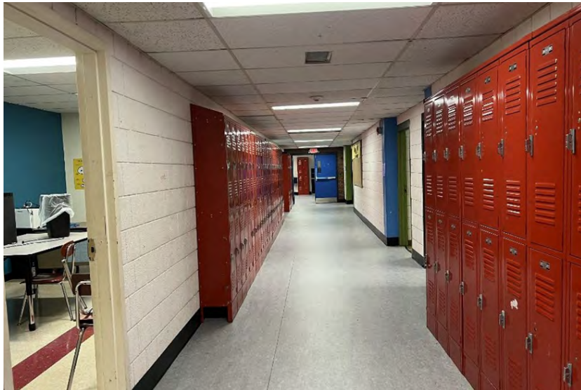
Third Floor Upgraded Corridor
