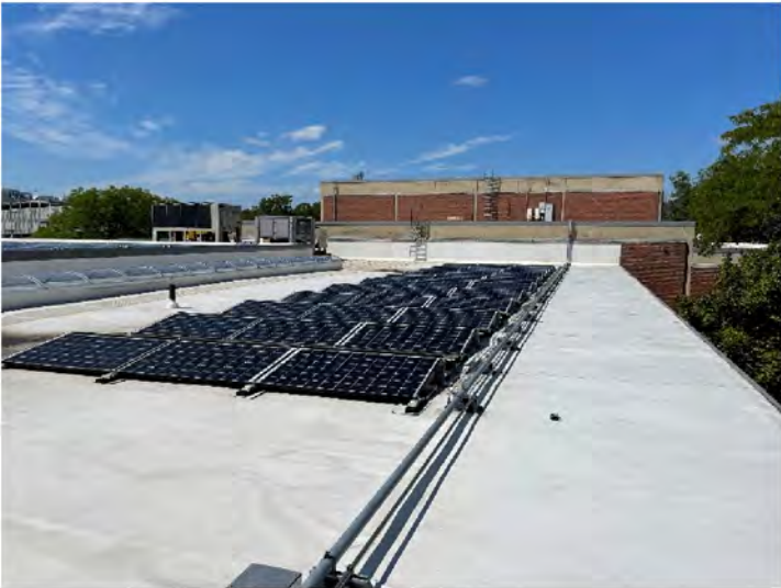
AE-46: Partial view of roof area over main lobby
