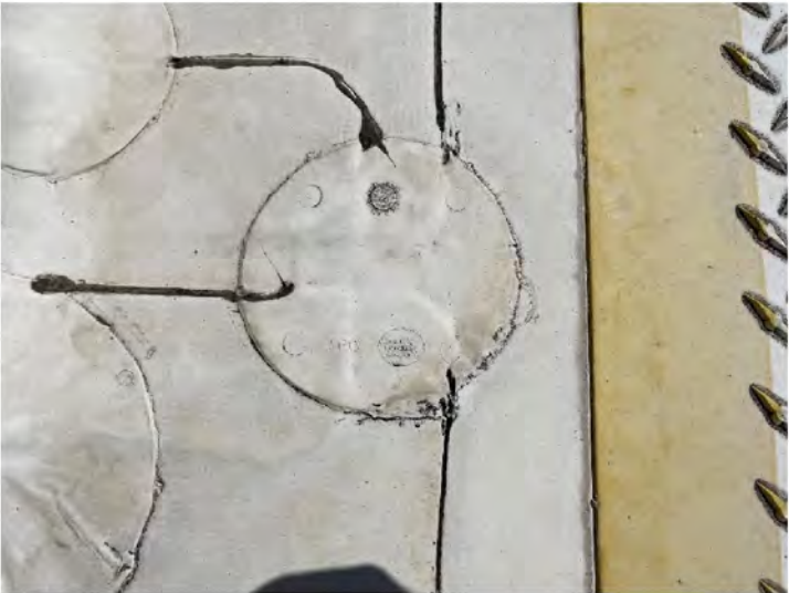
AE-57: Representative TPO patch at seam in roofing membrane
