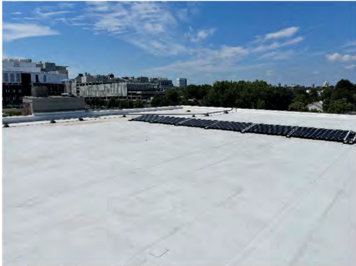
AE-44: Representative roof area
