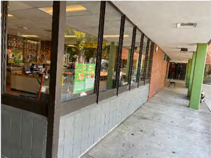
AE-29: Exterior of atypical steel framed window assemblies at front office
