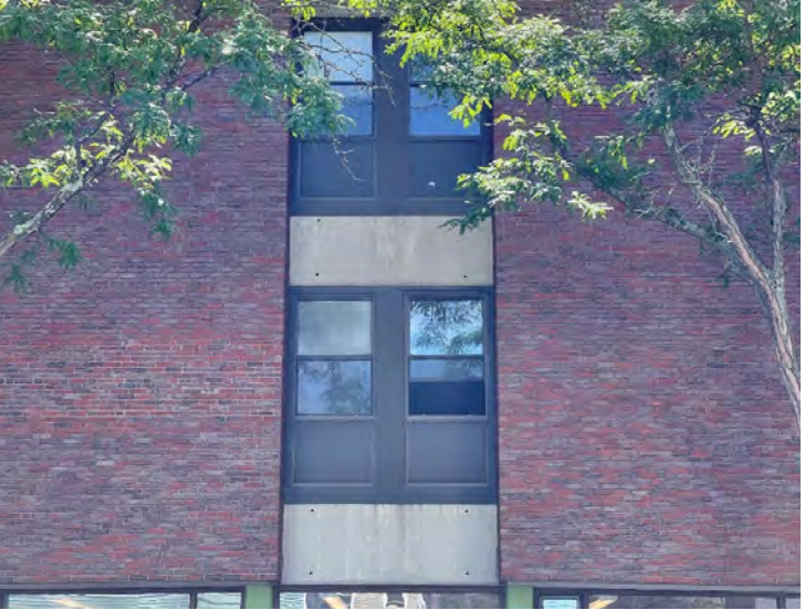
AE-B: Typical aluminum hung windows with aluminum spandrel panels
