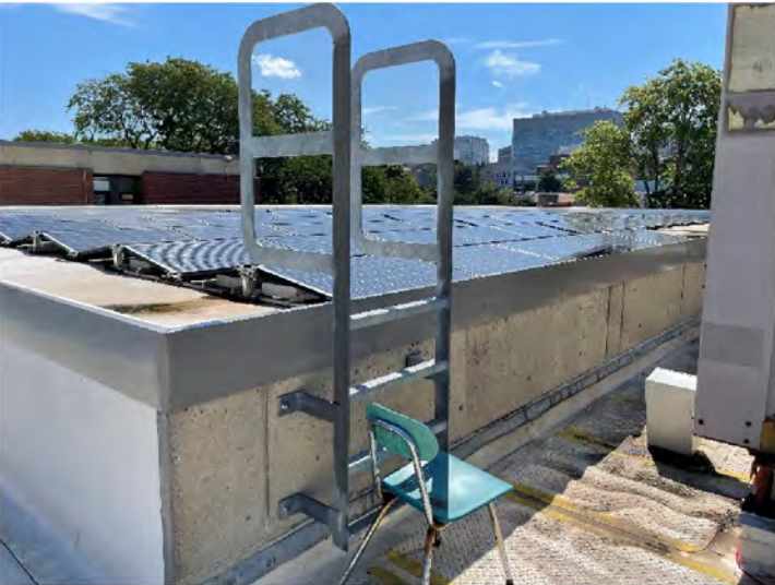
AE-58: Typical roof access ladder
