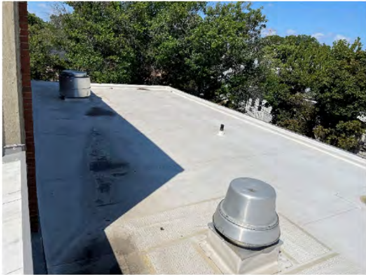
AE-50: Typical low roof, note some gathered sediment along cricket
