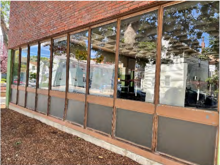
AE-30: Exterior of typical steel framed window assembly with fixed glass lites and metal spandrel panels.
