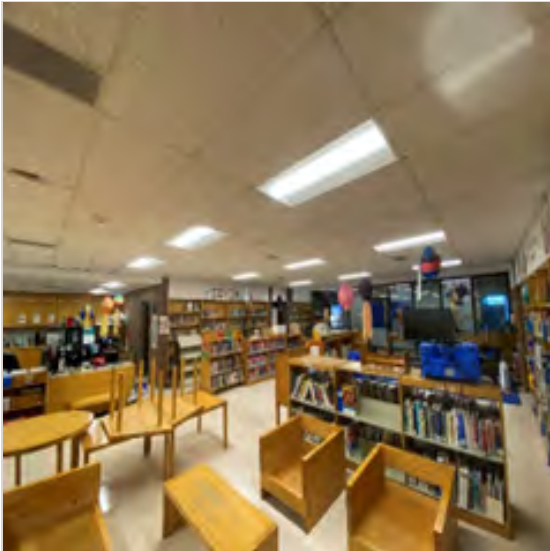
E-8: Typical Lighting Upgrade
