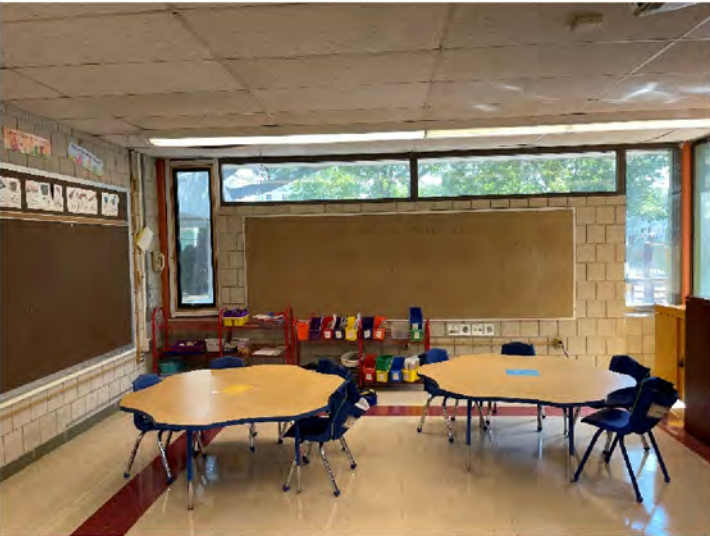
AE-34: Interior of typical classroom windows
