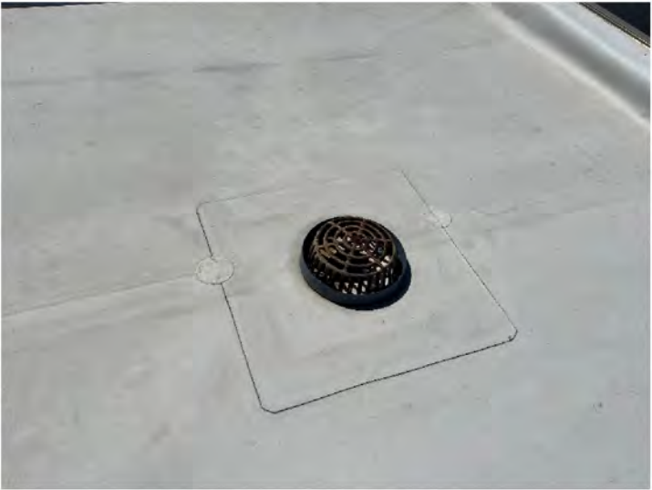
AE-54: Typical roof drain assembly
