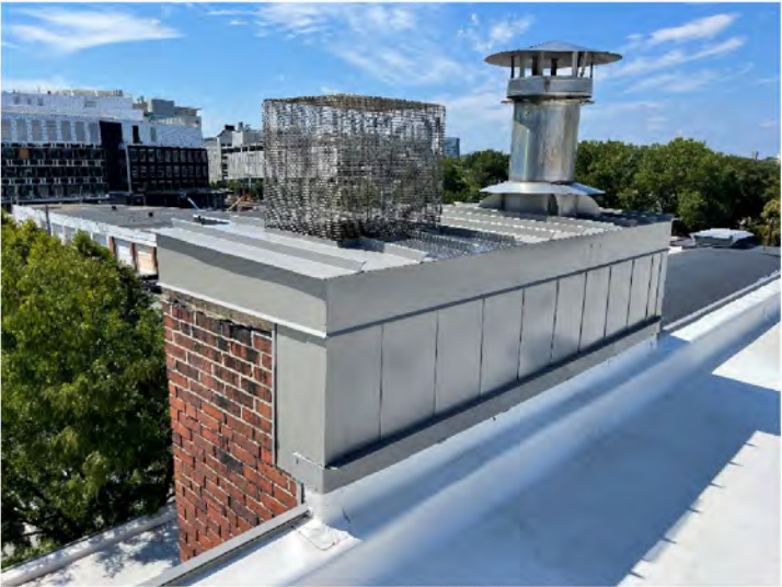
AE-59: Chimney with metal standing seam cap
