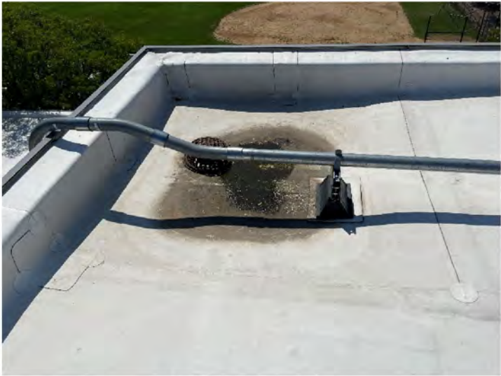
AE-53: Typical roof drain sump with some sediment build up
