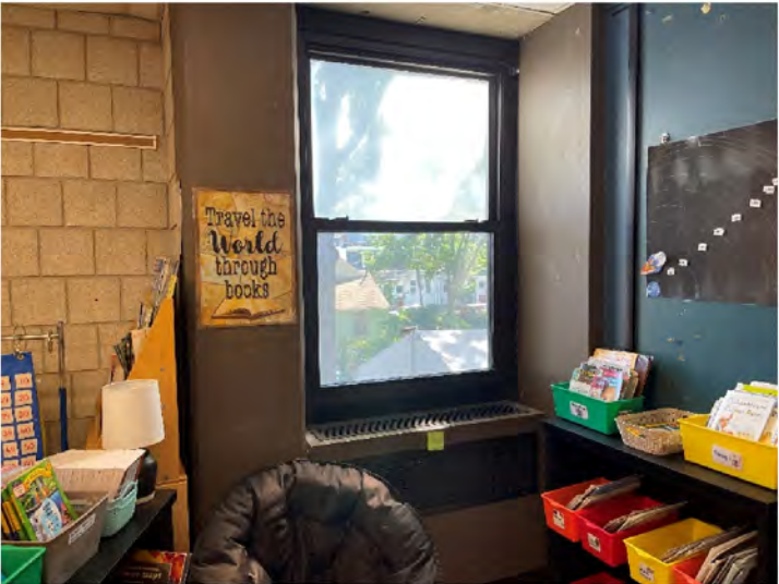
AE-33: Interior of typical aluminum window assembly within classroom
