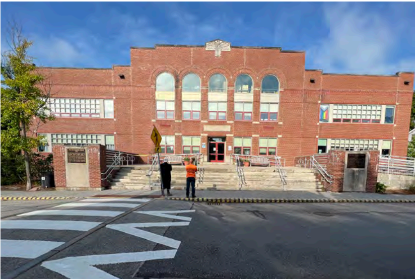
Front entrance, East
