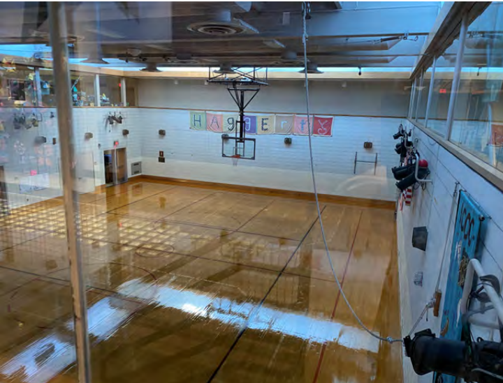
Two-Story Gym Floor Opening
