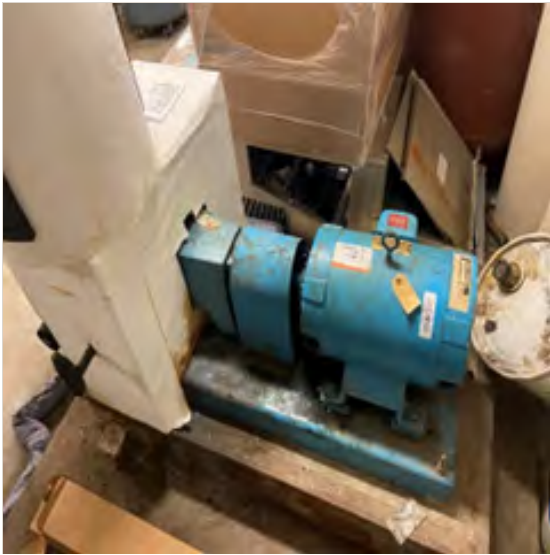
M-2: Original Dual-Temperature Pump
