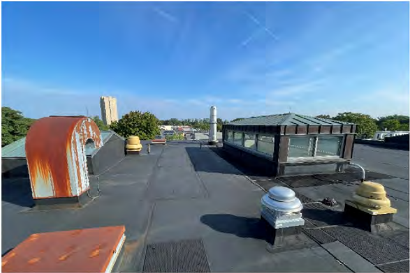
AE-37: General view of Main Roof
