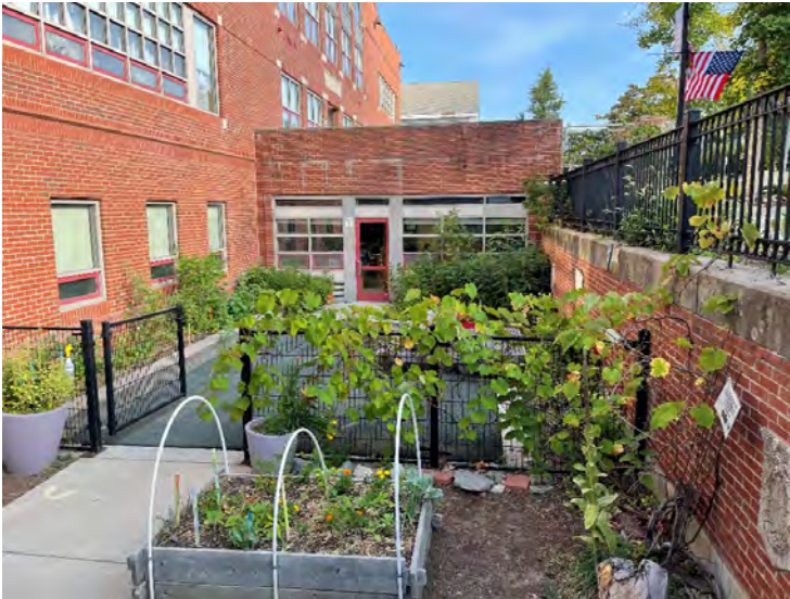
AE-A: East classroom wing below Main Entrance sidewalk
