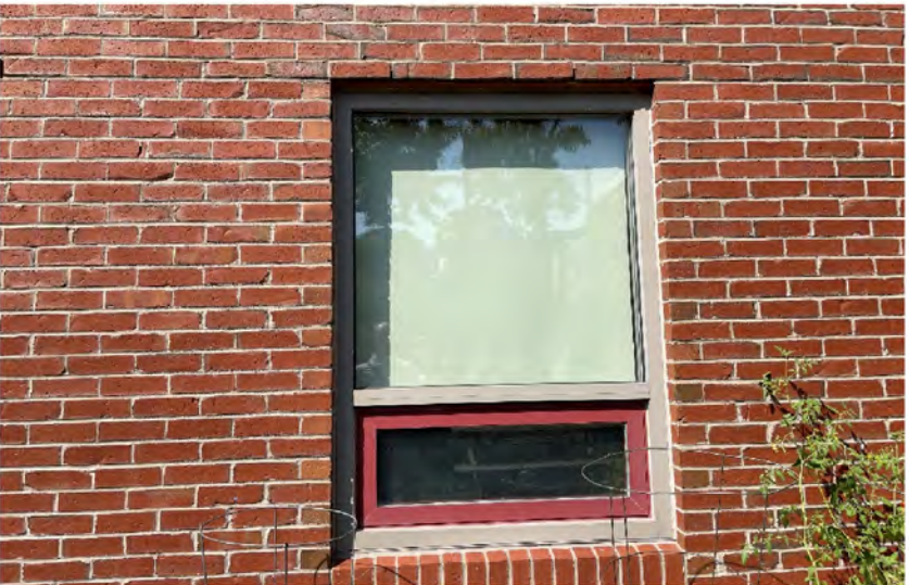
AE-24: Representative aluminum window assembly with fixed and operable components
