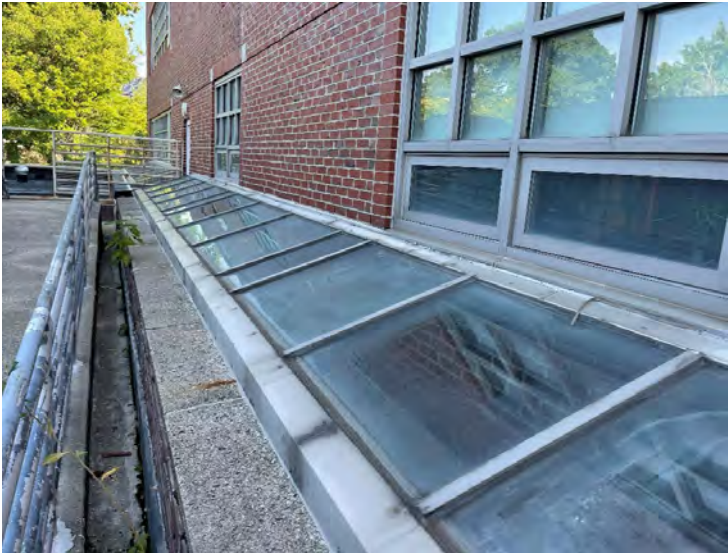
AE-B: Sloped glazing at transition from Main Building to West Wing
