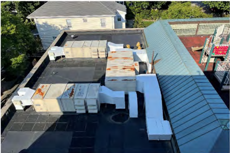
AE-39: General view at South portion of West Wing Roof: Note metal standing seam roofing over Gymnasium clerestory at perimeter of playroof
