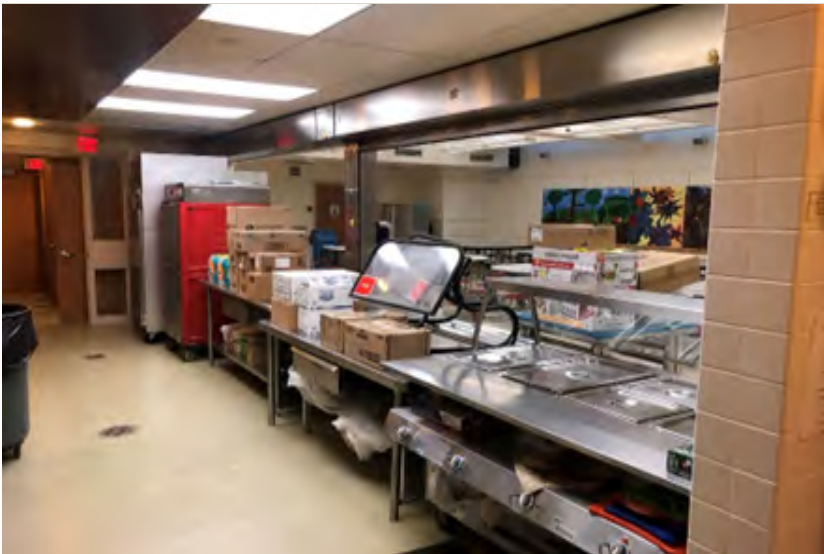
FS-2: Serving line components are made up of several different tables all at different heights. The tables also lack undershelves for additional storage capacity. The differential in heights make the serving area difficult to operate and challenging to clean. This photo also shows no refrigerated components which limit the ability to store and serve cold foods at proper temperatures.
