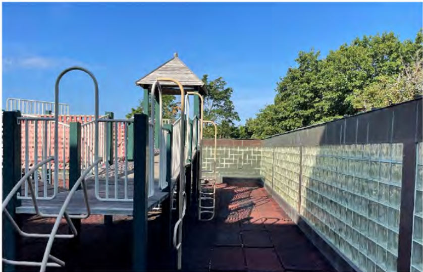
AE-19: Glass Block facades above roof at West Wing: These serve as clerestory for Gymnasium below
