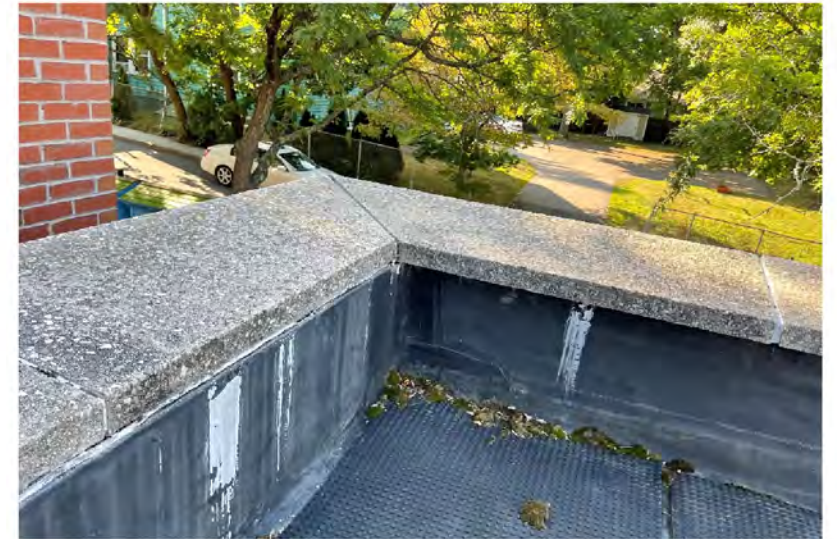
AE-8: Representative precast concrete coping cap at West Wing
