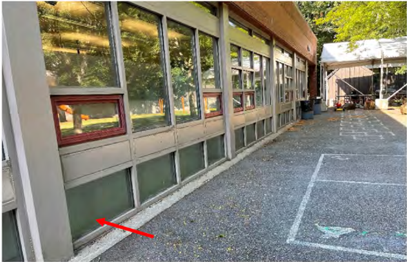
AE-25: Representative aluminum storefront at West Wing and East Classrooms below Main Entrance: Lower lites of storefront provide daylight into Cafeteria below.
