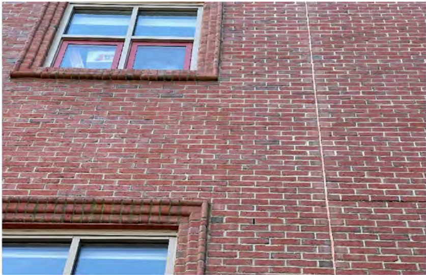
AE-6: Representative façade conditions: Brick veneer and aluminum window
