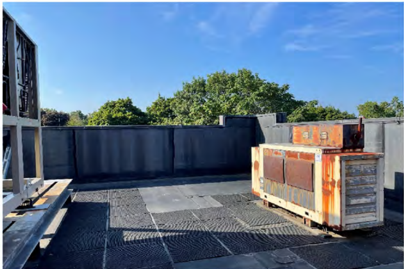
AE-36: Representative view of lower South EPDM roof at Main Building
