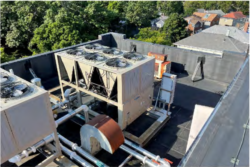
AE-38: Representative view of lower North EPDM roof at Main Building
