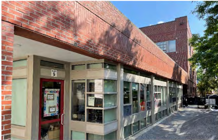
AE-5: South Elevation of West Wing
