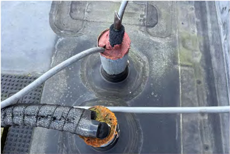
AE-45: Representative conduit penetrations in roof with spray foam and sealant applied around conduit.
