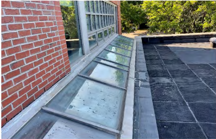
AE-29: Sloped glazing at transition between Main Building and West Wing, located above interior corridor
