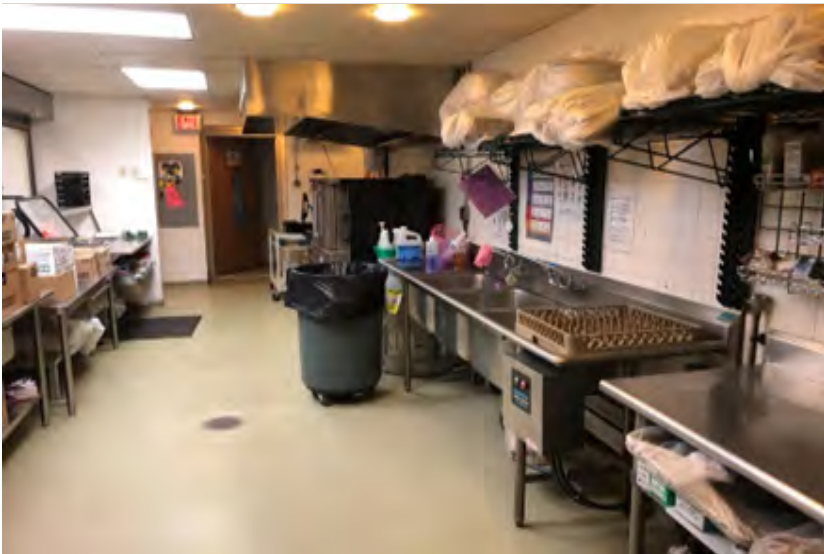
FS-1: The three-compartment sink is located directly adjacent to the cookline. With no dedicated food prep area, this sink is serving dual purpose as both preparation and ware washing. This situation presents cross contamination issues with modern day food code. The food code states that preparation and pot washing areas must be separated and labeled accordingly.
