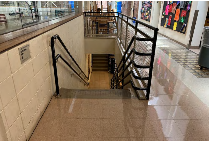
First Floor Corridor
