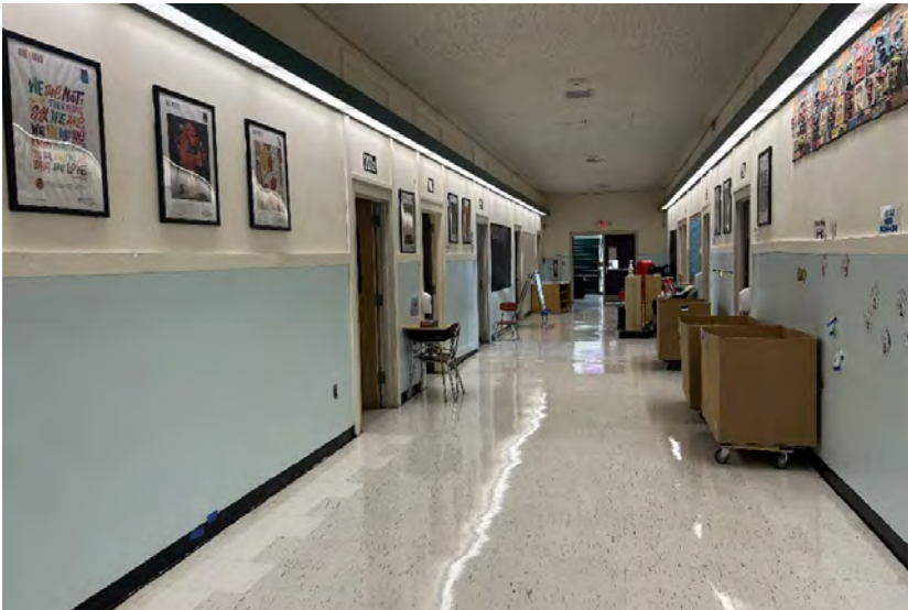
Typical Corridor – Second Floor
