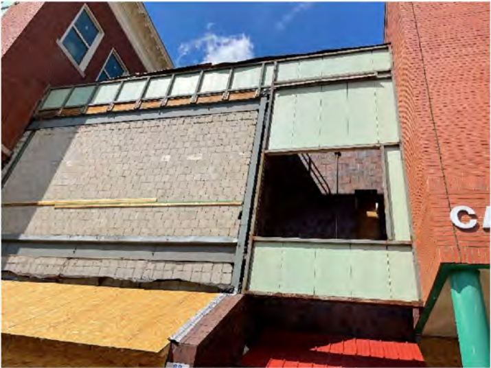
AE-22: Area on East Elevation where existing insulated metal panels have been removed, will be replaced.
