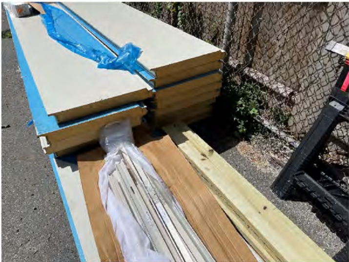
AE-23: New insulated metal panels stored on site for installation
