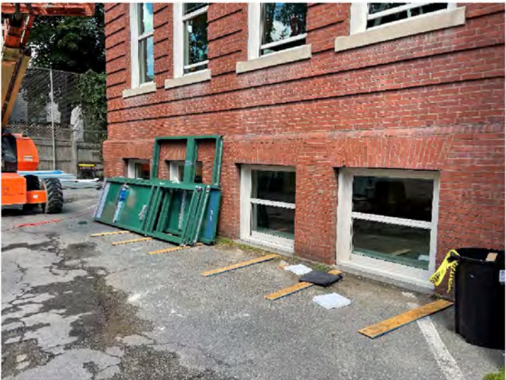
AE-24: Representative thermally broken aluminum storefront entrance stored on site, prior to installation
