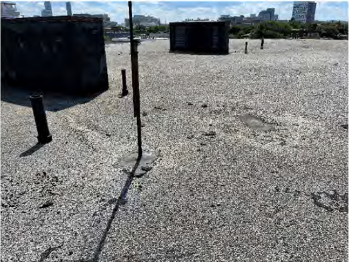
AE-38: Typical penetrations within South roof
