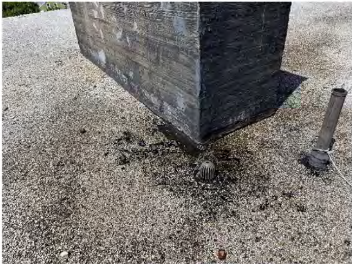
AE-36: Typical roof drain and penetrations in roof over South wing
