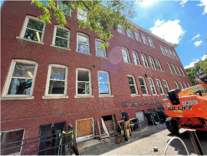
AE-6: West Elevation, South wing
