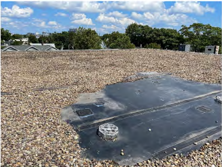
AE-31: Ballasted EPDM roof over Gymnasium, some ballast has been moved around
