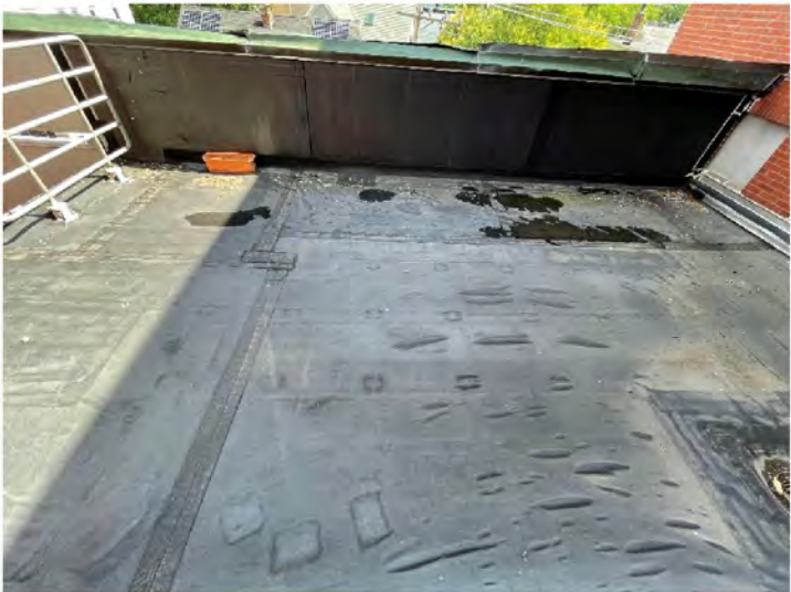
AE-28: Representative patches throughout East EPDM roof deck
