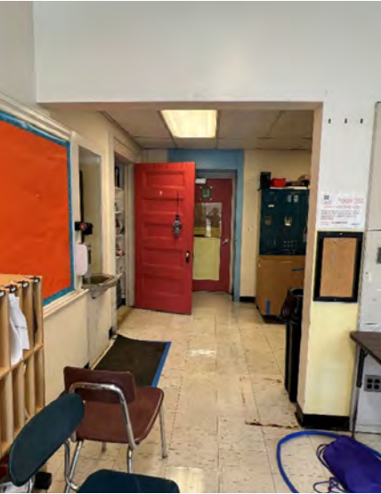
Typical Classroom Cubbie/ Entry Area – First Floor
