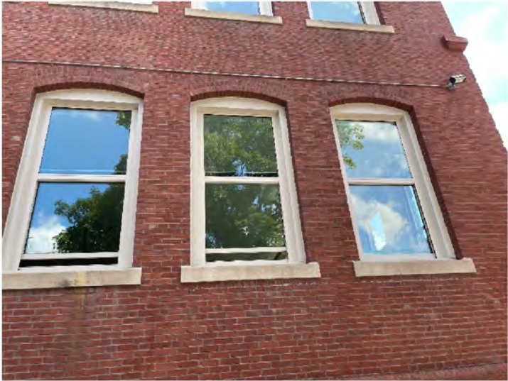
AE-7: Representative multiwythe brick masonry with limestone sills and new windows at South wing
