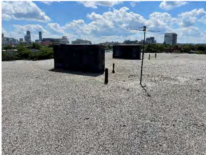
AE-35: General view of roof over South wing
