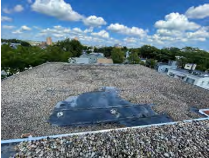
AE-D: General view of ballasted EPDM roof at North addition over Gymnasium
