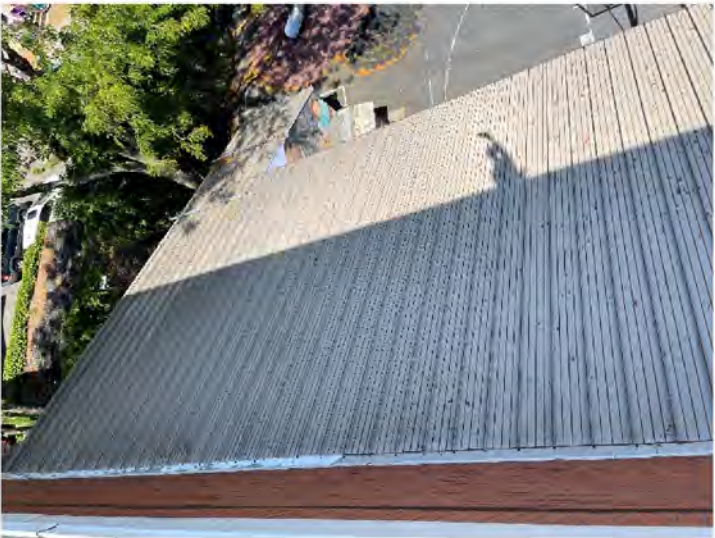
AE-40: Metal roofing over Stage and stair at North end of building
