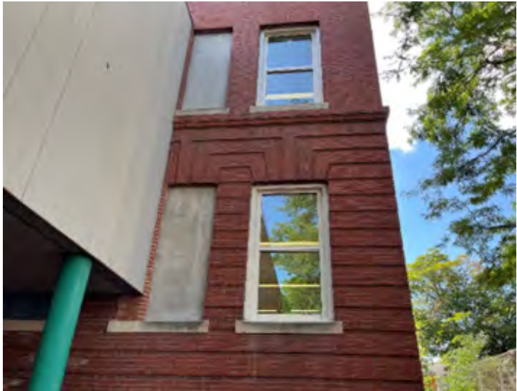
AE-B: Transition from original building to North addition along West Elevation
