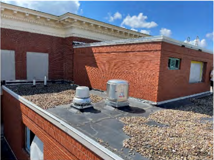
AE-30: Mid-level roof at East side of North wing.
