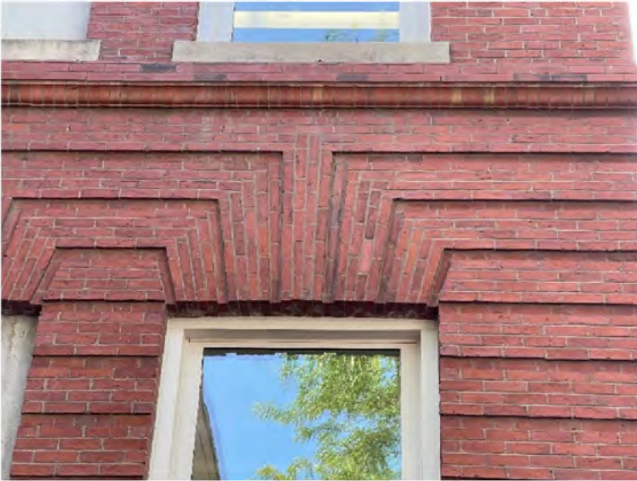
AE-8: Representative multiwythe masonry at South wing
