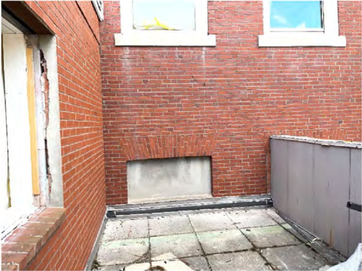
AE-26: West roof deck, covered with pavers
