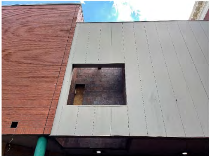
AE-20: Typical insulated metal panel façade along East Elevation of South wing
