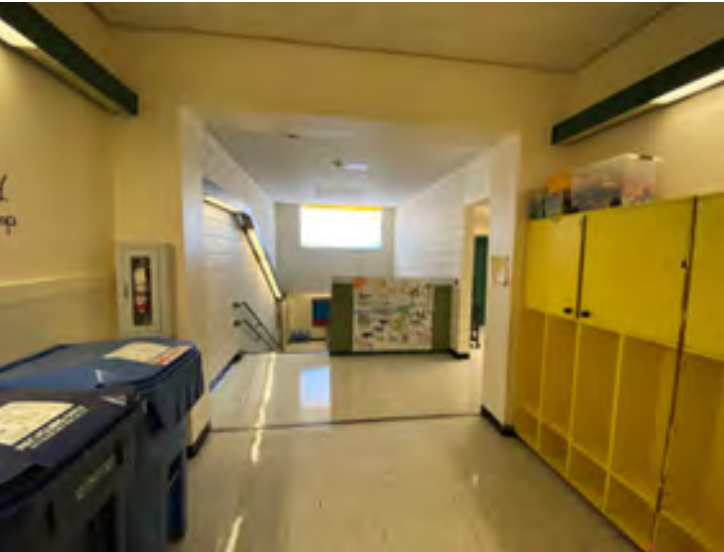
Open Stair At 3rd Floor
