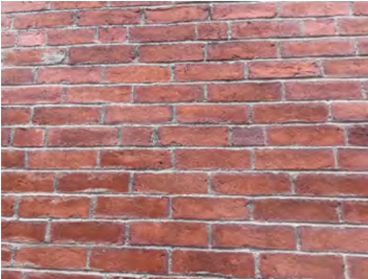
AE-A: Representative multiwythe brick masonry at South wing / original building
