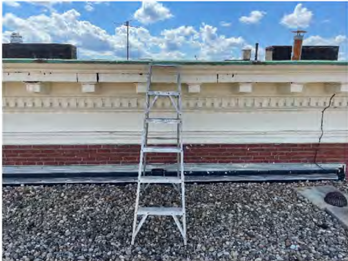
AE-34: Step ladder used to achieve roof access to South wing roof
