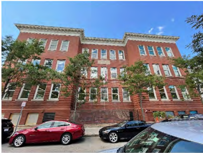
AE-2: East Elevation, South wing
