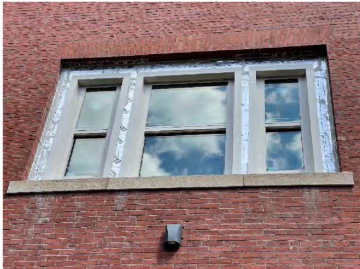
AE-9: Representative multiwythe masonry with limestone sills and new windows at South wing
