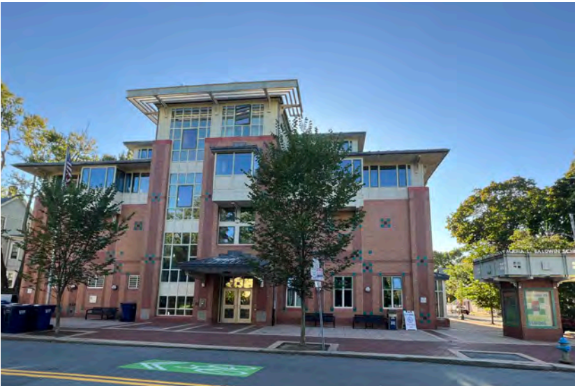
East Side of Site
