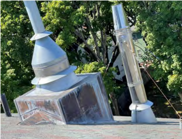
AE-D: Representative MEP penetrations in shingled roof
