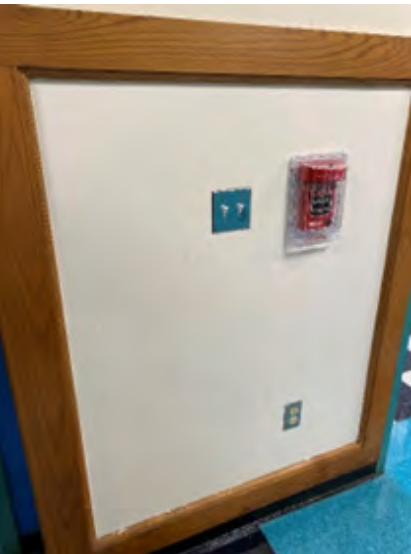
E-3: Switch and outlet condition
