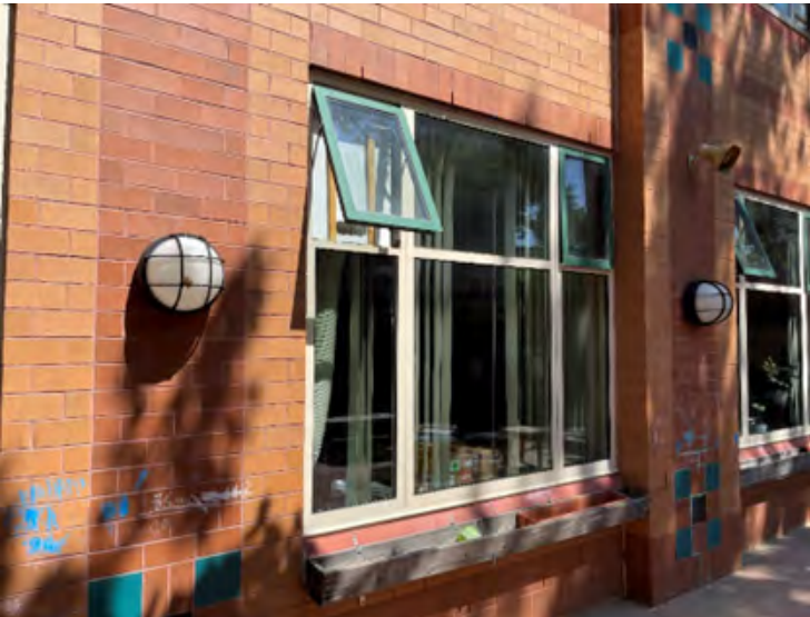
AE-B: Representative fenestration with fixed and operable components
