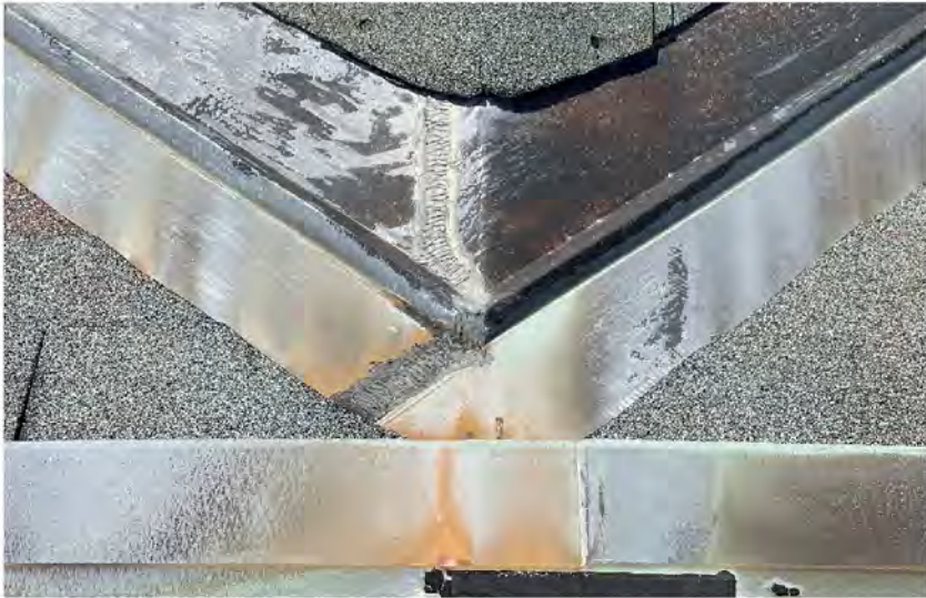
AE-26: Representative metal valleys, roof edge flashings within shingled roofing system
