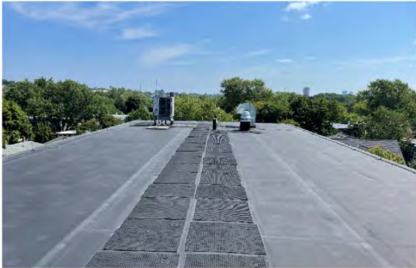
AE-21: General view of EPDM roof
