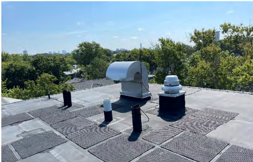
AE-23: Representative roof vent penetrations, vent hood on curb
