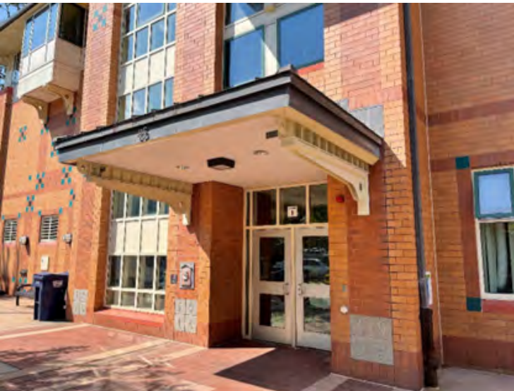
AE-A: Main Entrance, representative brick and curtain wall assemblies
