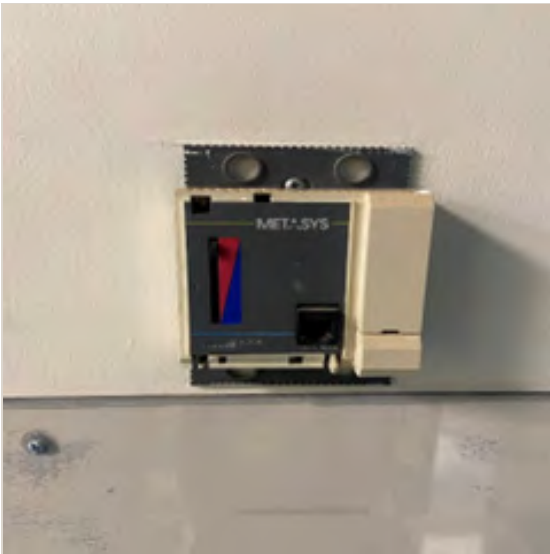
M-7: JCI Metasys Temperature Sensor
