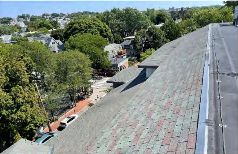
AE-25: Representative asphalt shingled roofing at transition with EPDM
