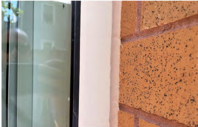
AE-12: Representative window perimeter sealants in good condition
