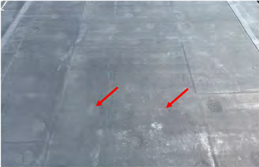
AE-22: Representative EPDM membrane, adhered to mechanically fastened substrate. Fastener plates visible from below membrane.
