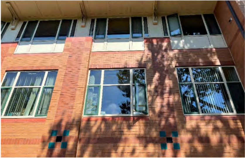
AE-5: Representative façade conditions: Metal soffit panels, brick masonry and storefront assemblies.
