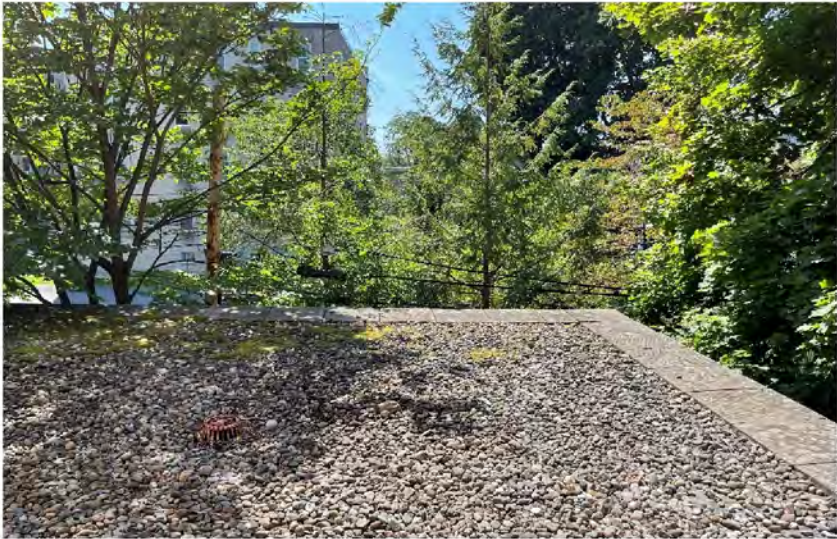
AE-30: Ballasted roof at South Elevation
