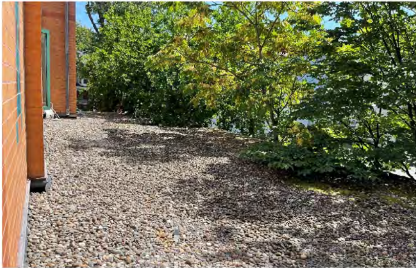
AE-29: Ballasted roof at South Elevation, looking East
