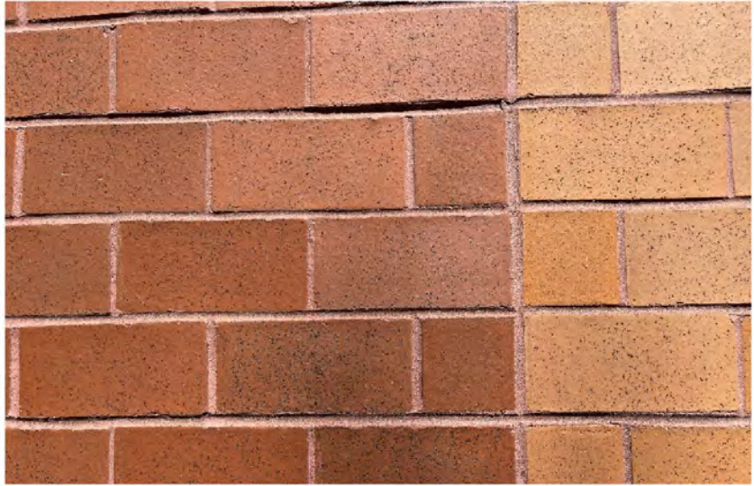
AE-7: Representative brick masonry facade
