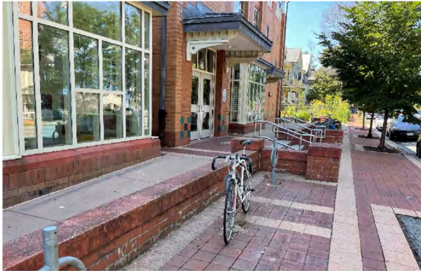
AE-33: Representative masonry walls along ramp at North Elevation
