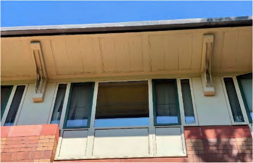
AE-6: Representative façade conditions: Metal soffit panels, brick masonry and storefront assemblies.
