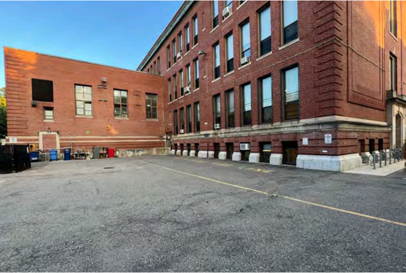
Drop off/parking area, North
