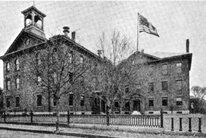
Webster School, Upton St., Demolished. Buildings Survey of Architectural History in Cambridge: Cambridgeport by Cambridge Historical Commission, The MIT Press 1971, 92.
