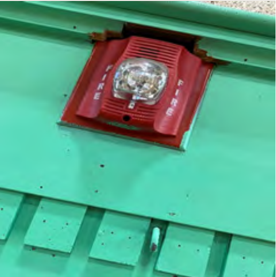
E-5: Existing Fire Alarm Device
