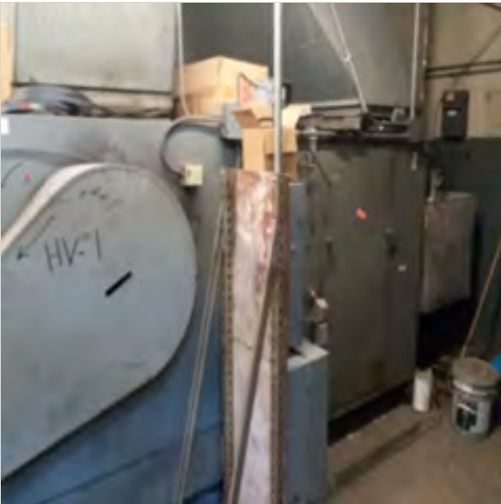
M-5: General Condition of Unit HV-1
