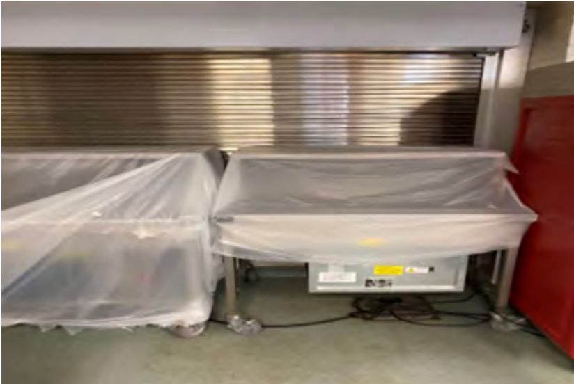
FS-2: The serving counters are limited to only (1) each of mobile hot and cold mobile units. For this population of students, the operations team would greatly benefit from additional temperature-controlled food at the serving line. The sneeze guards are full length and make passage of food to be challenging.
