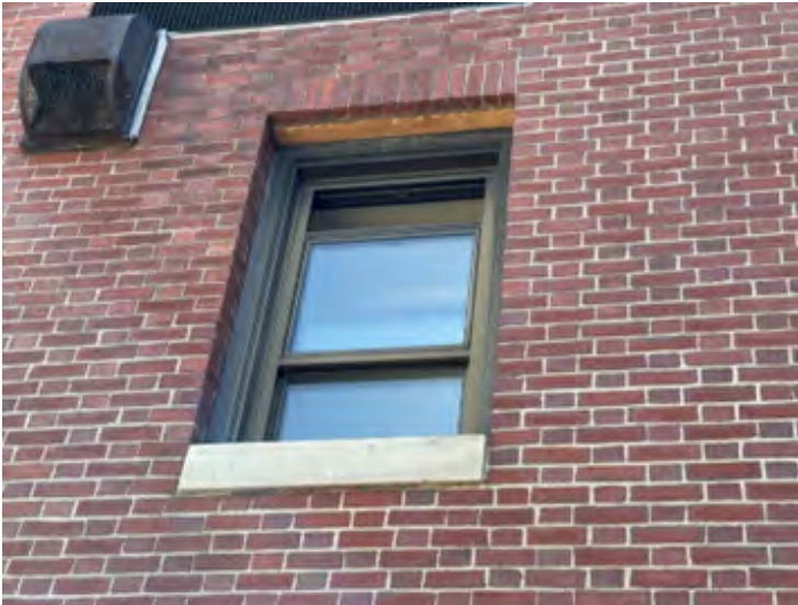
AE-B: Typical aluminum window within brick masonry façade, with limestone sill and painted steel lintel.
