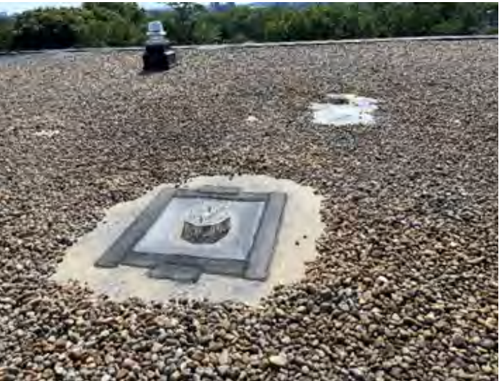
AE-D: Representative ballasted EPDM roof with newer roof drain assembly.
