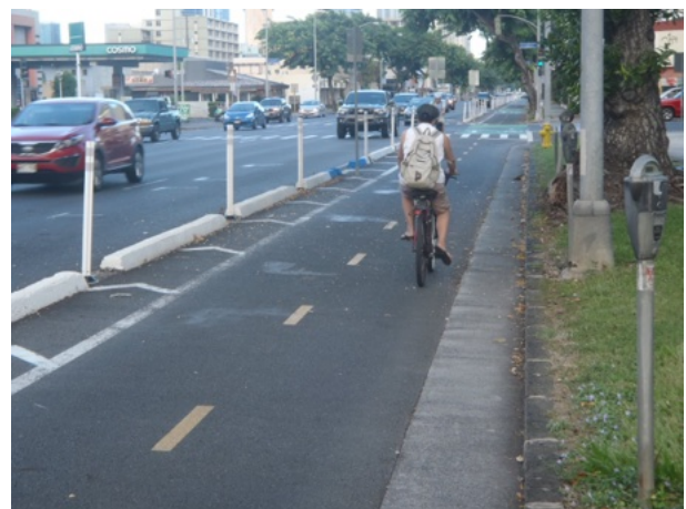
Example of protected bike lane created with paint, curbing, and vertical delineators.
