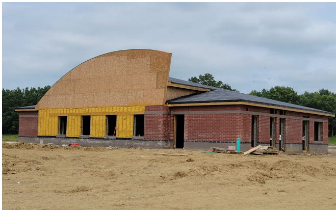
Multi-use athletic building with ticket booth, restrooms, and concession stand
