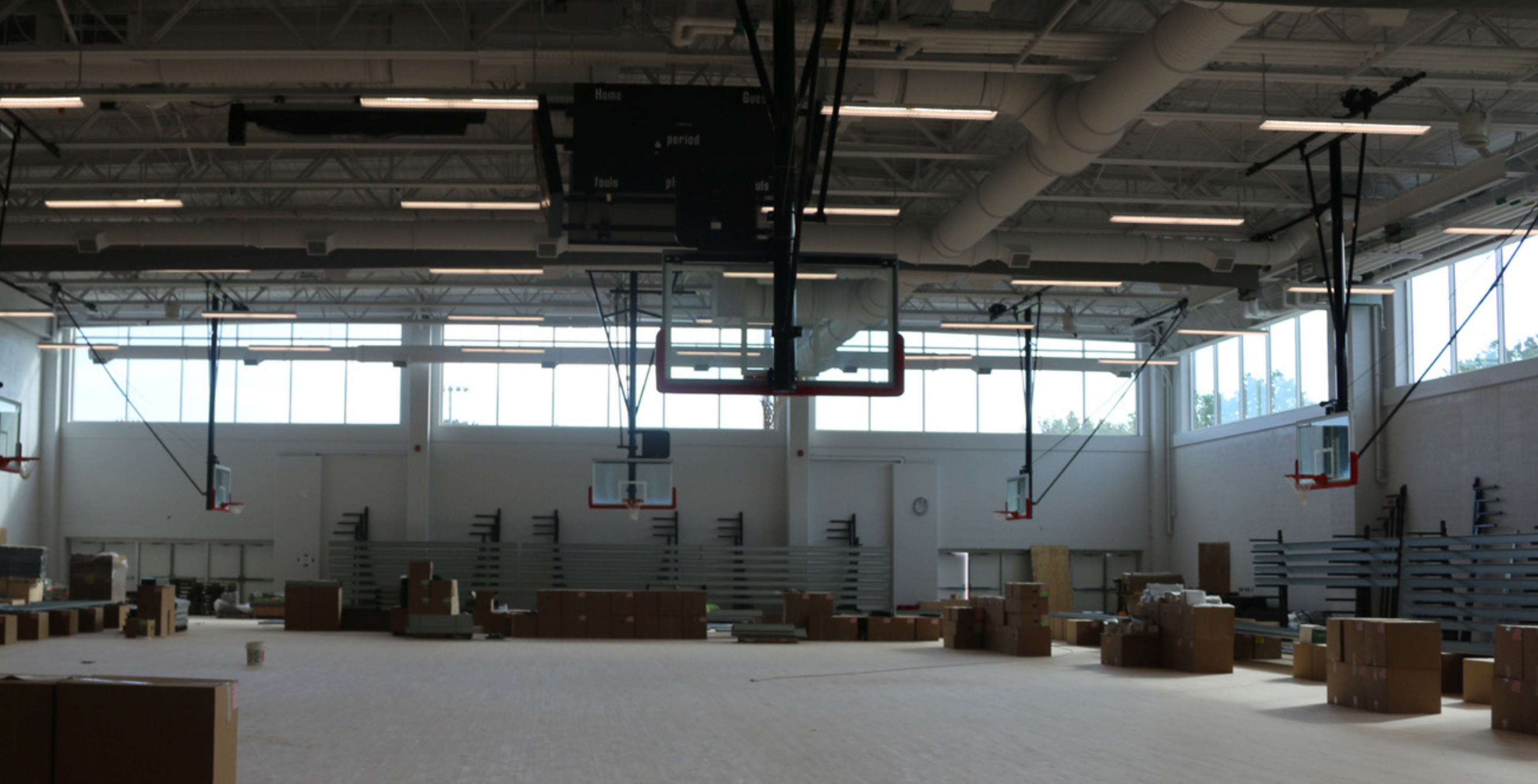
Main gymnasium Gimnasio principal
