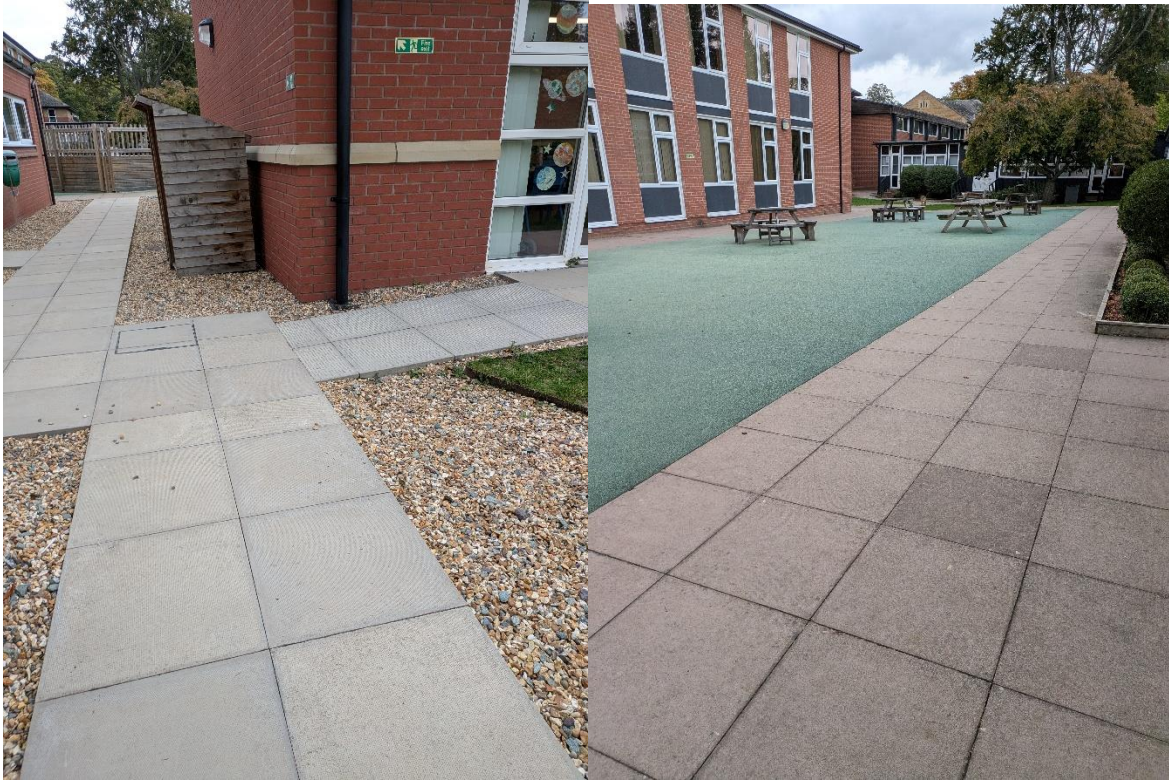
Outdoor flooring adapted; patio slabs increase accessibility.
