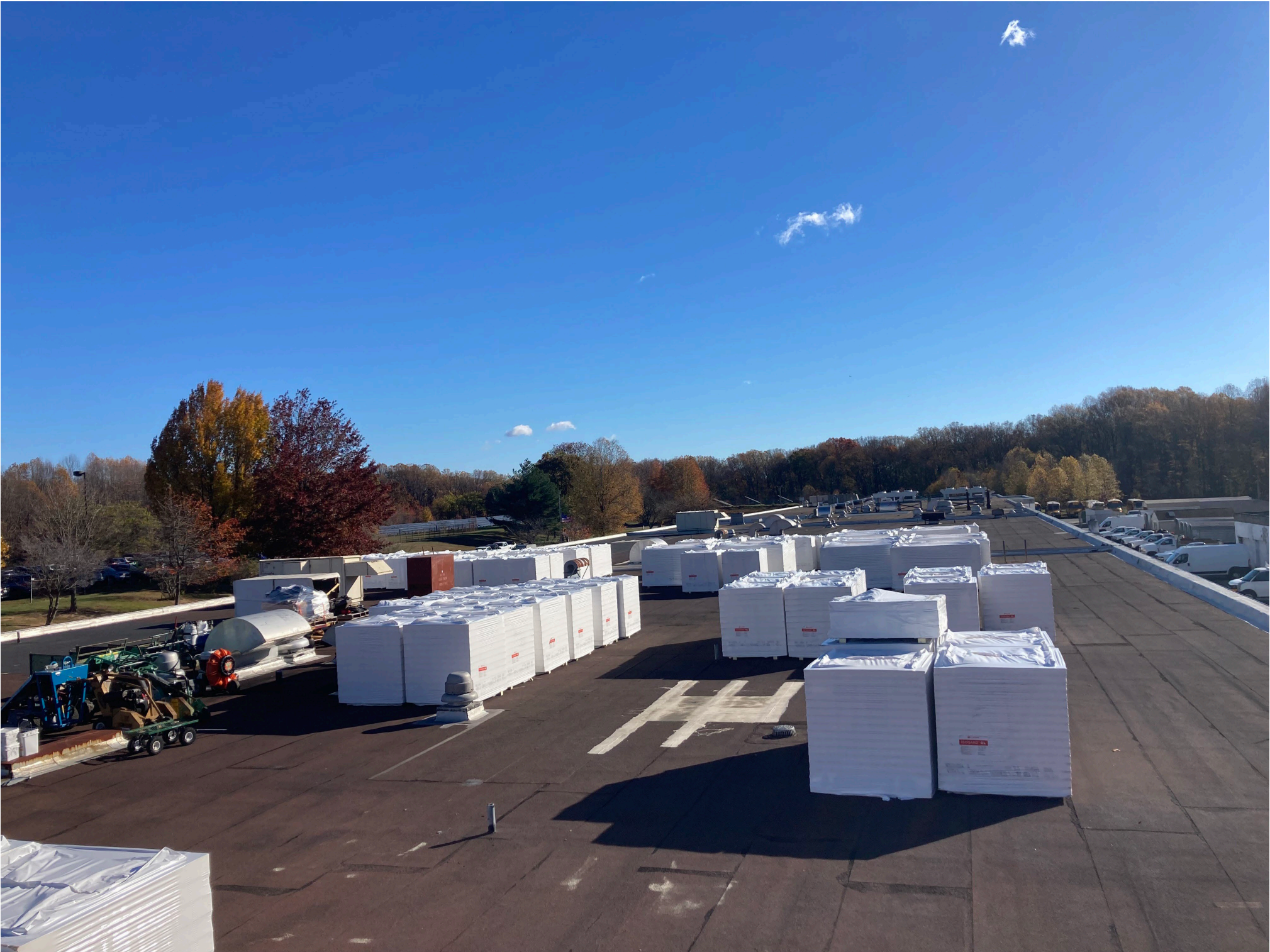
ADMINISTRATIVE SERVICES CENTER – ROOF REPLACEMENT
