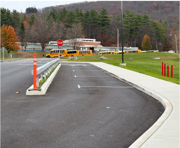
New drop-off lane at the West End. Complete and functional.
