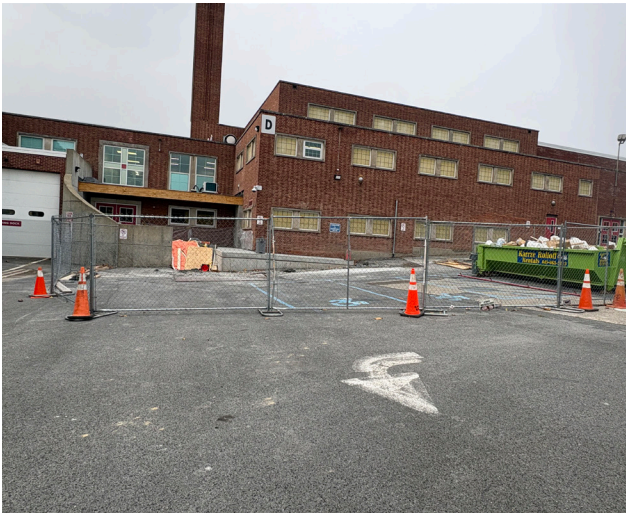
Loading Dock Entrance—still under construction. Check back in for updates next issue!
