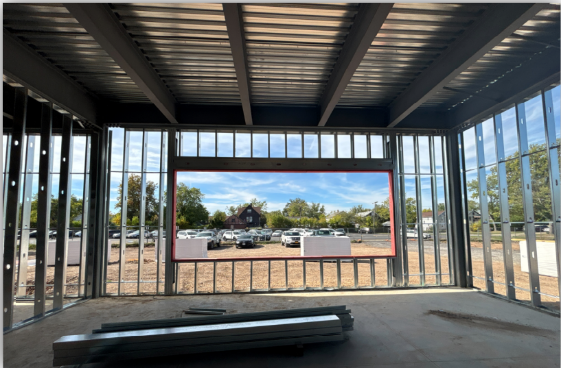
Metal Framing at Windermere UPK Addition
