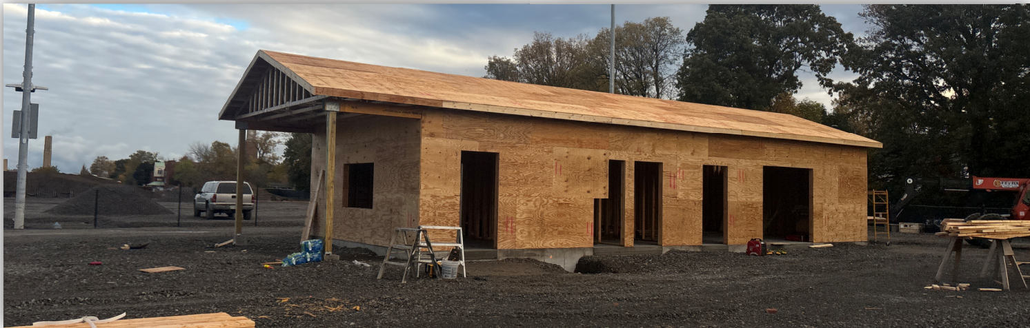
Wood Framing Process at the Concessions
