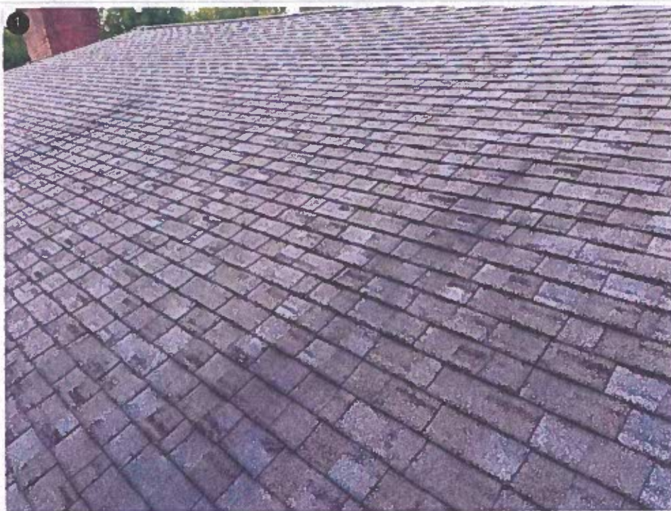
The pitched sections are served by asphalt shingles, which are estimated to be 25+ years old
