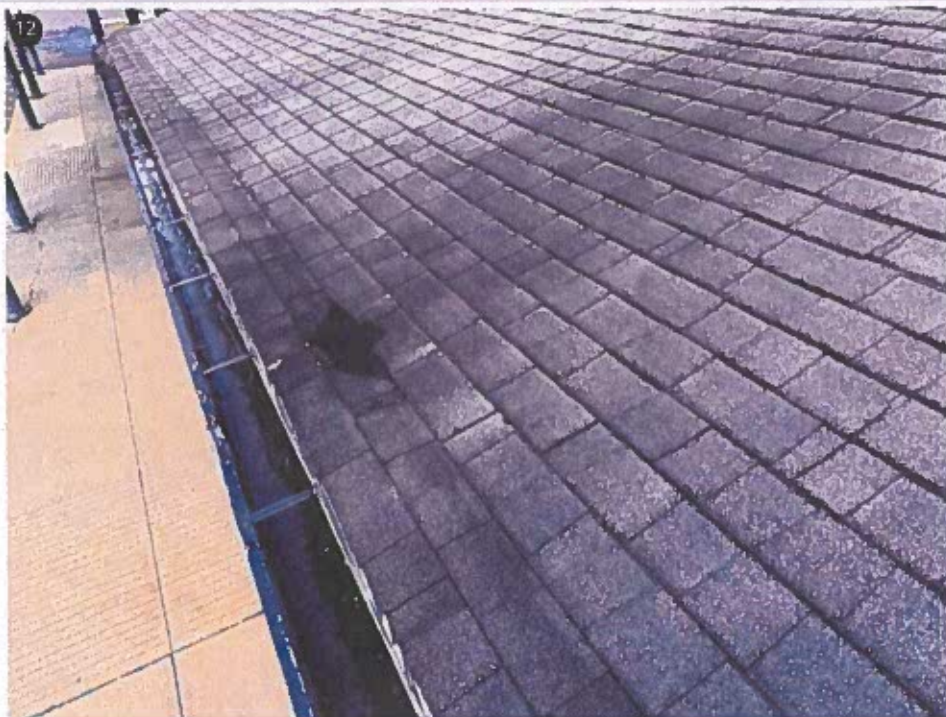
Lower roof over the administration offices
