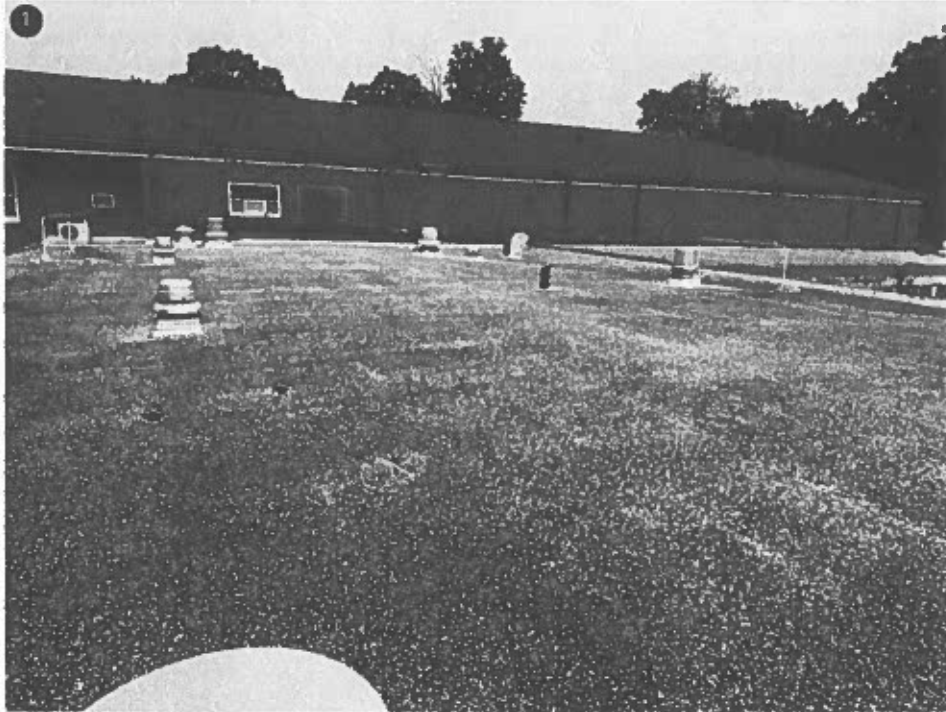
Overview of the low-slope roof. Multi-ply modified roof system in hot asphalt with a gravel surface.
