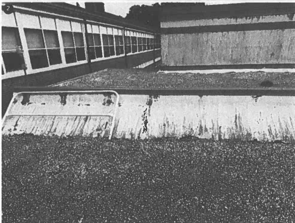
In spite of being 10 years old, the flashings are holding up well. Typically, flashings and perimeters are the first components of a roof to first show signs of issues.
