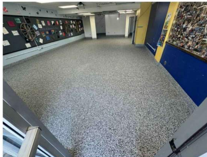
PR08 Epoxy Flooring Complete
