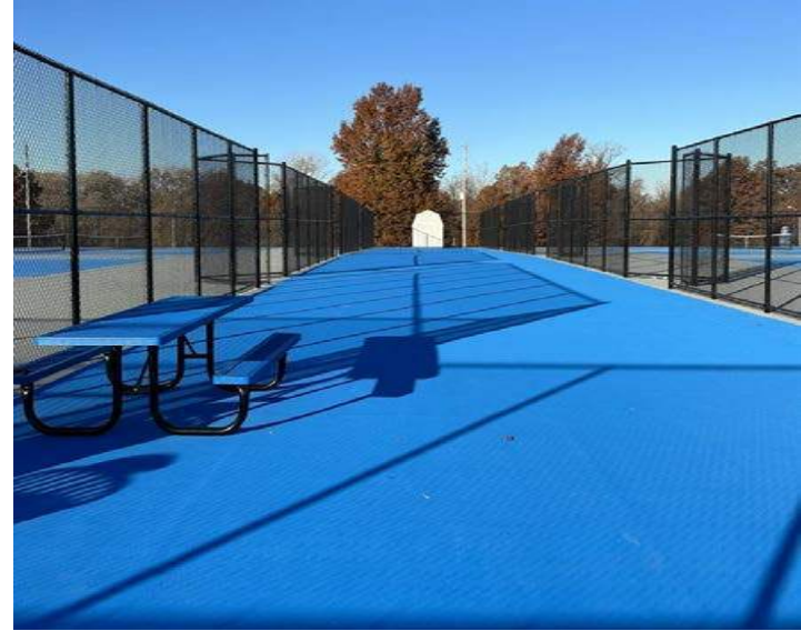
Center Spectator Concourse Looking West
