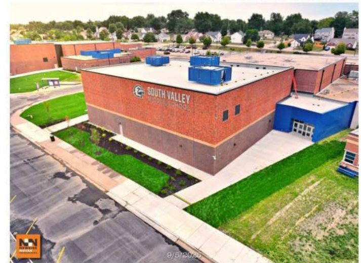
SVMS Exterior View
