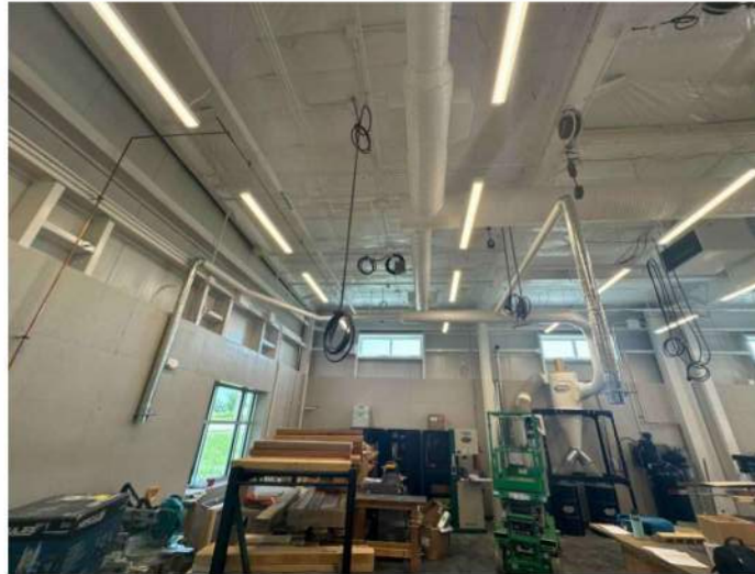
Dust Collection Install Complete in Shop
