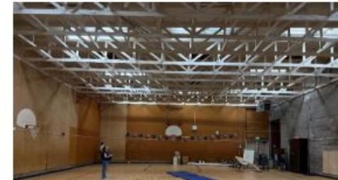
Auxiliary gym with no acoustic treatment.
