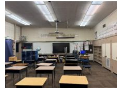
5. Typical classroom, original casework, fluorescent lighting, painted block at exterior wall.
