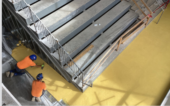
09.25 - The terrazzo mixture at Eastman is made up of marble chips and concrete.
