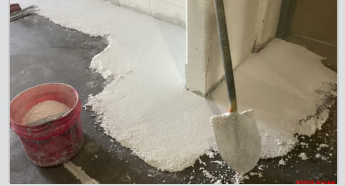
09.25 - The terrazzo mixture at Eastman is made up of marble chips and concrete.
