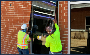
First floor glass install (Area B)
