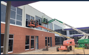
Glass stop install (Area B)
