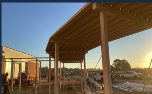
Bus canopy install
