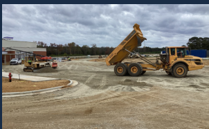
ABC stone placement at bus parking
