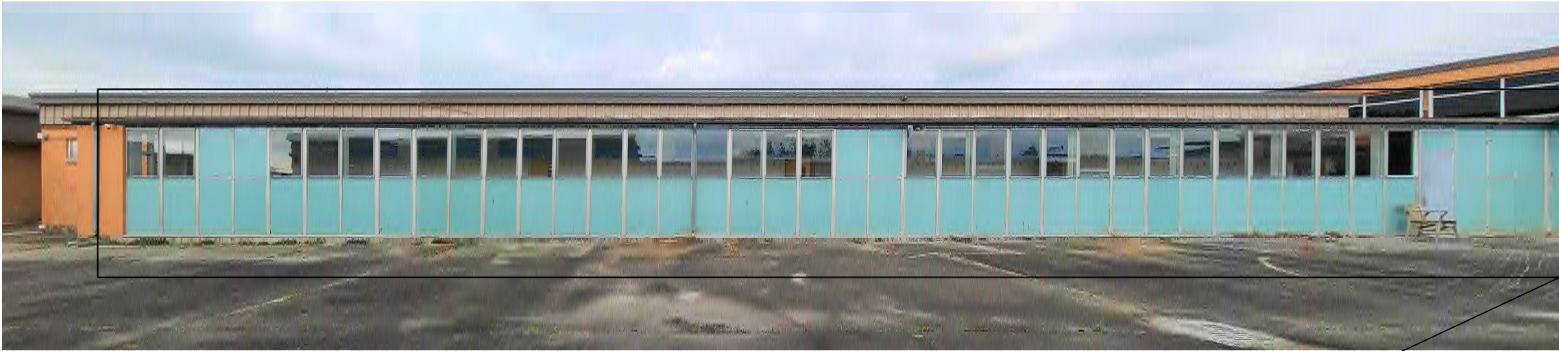
EXTERIOR TRANSITE REMOVAL - REFERENCE ARCHITECT SHEET A2.03 - NOT TO SCALE
