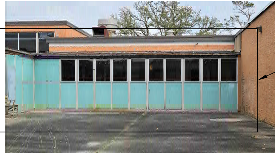
EXTERIOR TRANSITE REMOVAL - REFERENCE ARCHITECT SHEET A2.05 - NOT TO SCALE
