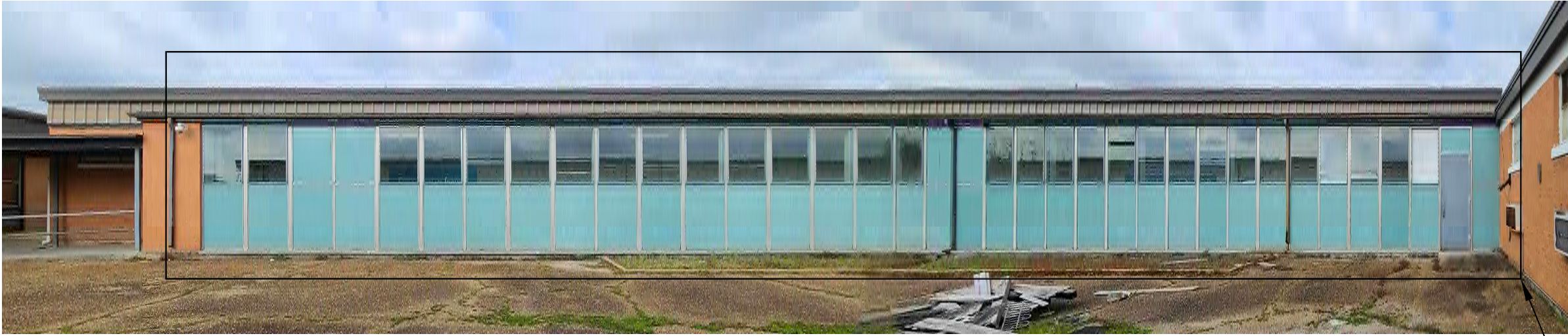
EXTERIOR TRANSITE REMOVAL - REFERENCE ARCHITECT SHEET A2.02 - NOT TO SCALE
