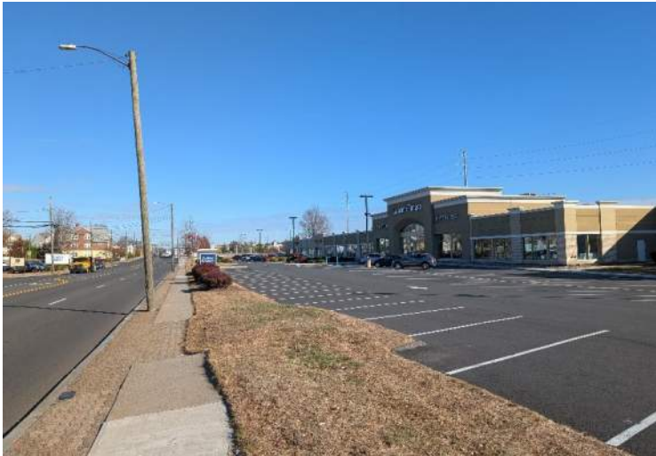
Exhibit 15: Vegetation overgrowth on sidewalk
