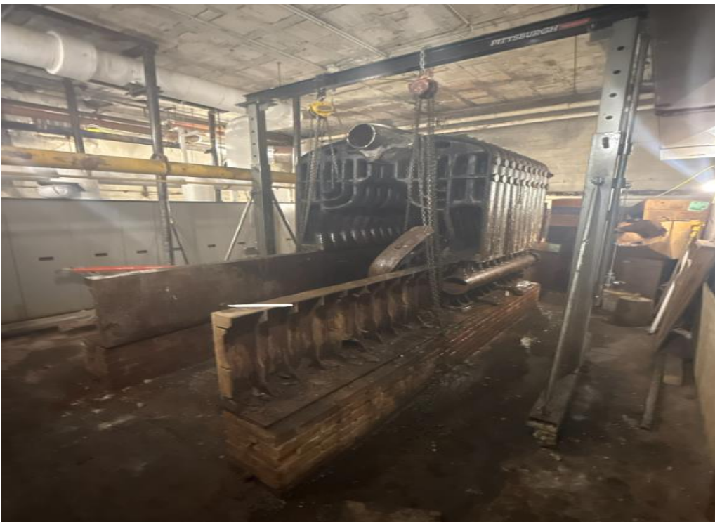
Hempstead ABGS MS – Boiler Abatement/Demo
