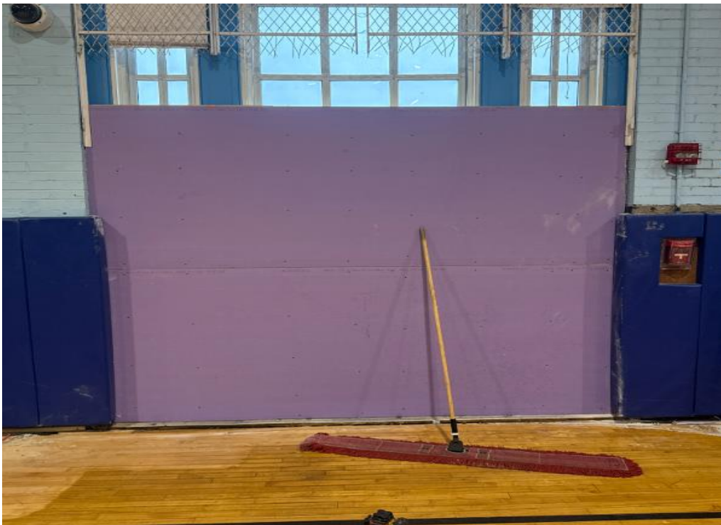
Hempstead ABGS MS – Temp Smoke Doors/Partitions
