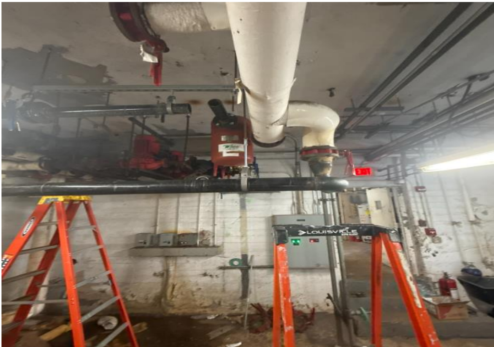
Hempstead McNeil ES – Boiler Replacement
