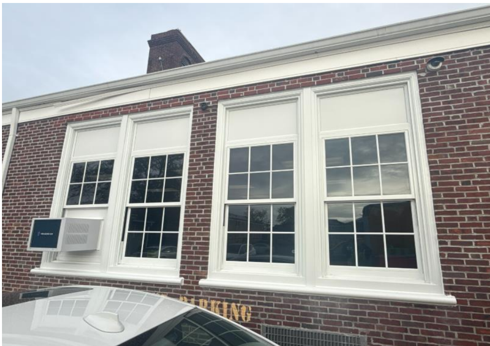
Hempstead McNeil ES – Window Replacement
