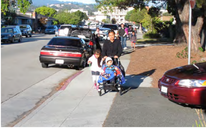
Driveway crossings without landings result in uncomfortable cross-slopes.
