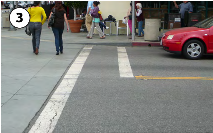
Advance stop bars provide more space for pedestrians and increase visibility.
