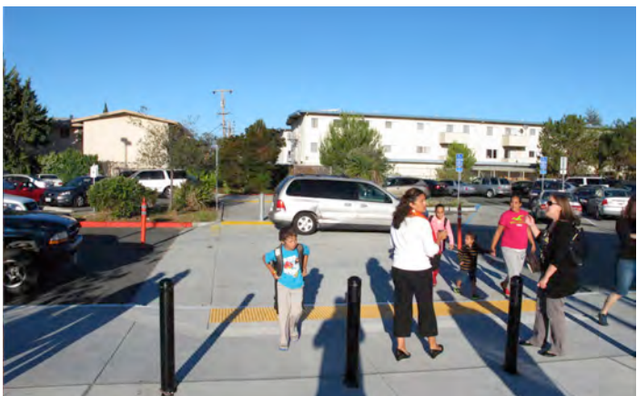
Raised crosswalks encourage slower travel speeds.
