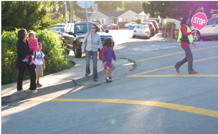
Several intersections near the school lack corner curb ramps.
