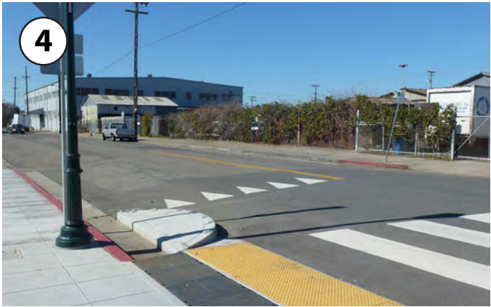
Advance yield lines/sharks teeth instruct motorists where to yield at uncontrolled crosswalks.
