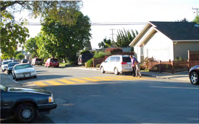
Parked cars impede the line of sight for crossing pedestrians at the uncontrolled crosswalk.
