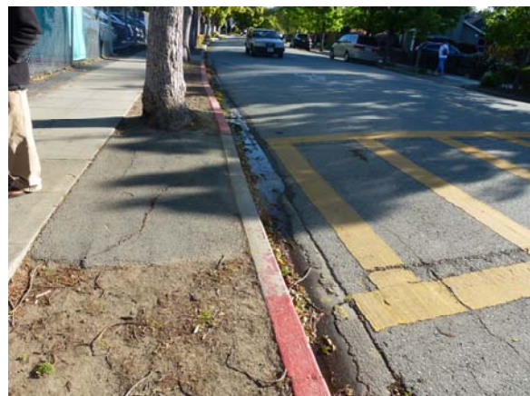
The midblock crossing of Arroyo Avenue needs some improvements for accessibility.
