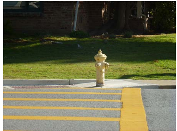
The intersection of Cordilleras Avenue and Belle Avenue has sidewalk, curb ramp, and drainage challenges.
